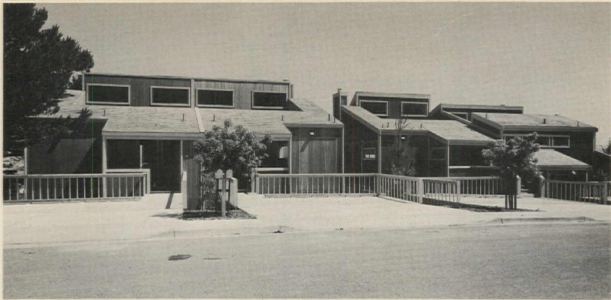
Uphill elevations of downhill townhouses have two-car parking pads which lead to sheltered entrance decks and outside storage.
