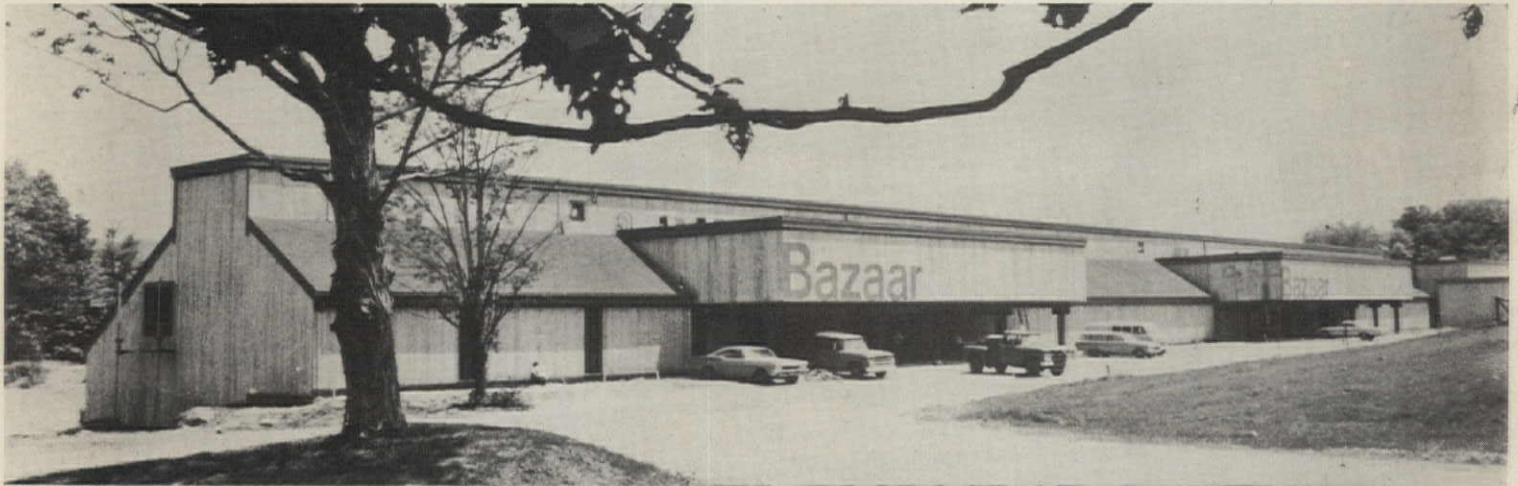
Plan of 50,000-sq.-ft. Bazaar (top) puts shops on four different levels connected by stairways (right). Shaded areas are shown in photos. All-wood building (above) is heated and cooled by heat pumps.
