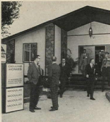
Romney's tour of convention begins with visit to modular house, then . . .
