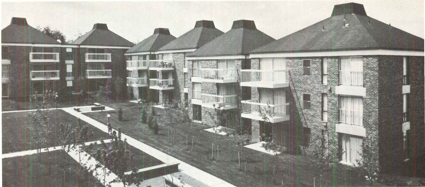
Living room balconies face garden courts—away from parking areas—offering further privacy. Wood-truss roof is capped with cupola, creating distinctive design.
