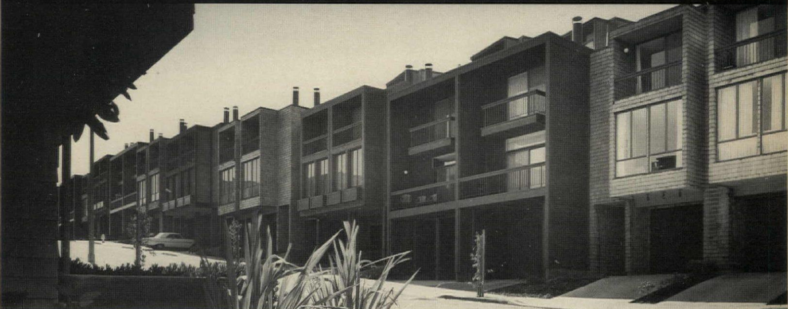
Gold Mine Hill Apartments, San Francisco, California. Certigrade Shingles No. 1 Grade, 18" Perfections. Architect: Fisher & Friedman Associates
