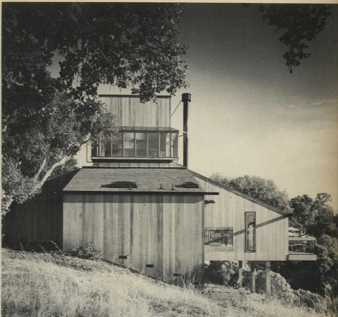
Side view of house shows master bedroom wing in foreground and living room wing at right. Perimeter skylights beneath rooftop studio bring daylight into central gallery.
