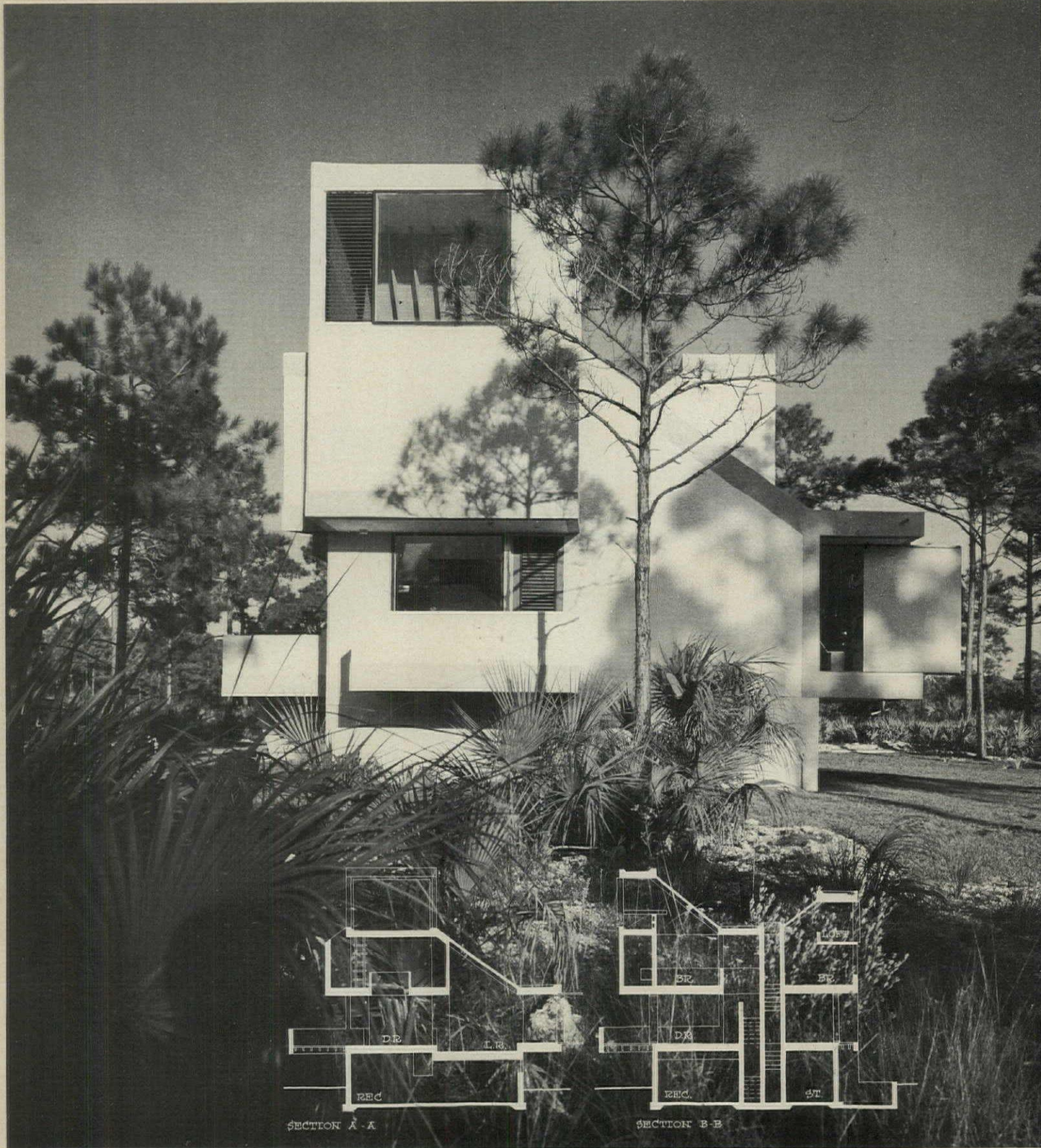
Projecting boxes (photo above) enclose the master bath, in center on the third level; a loft above it; and a living room extension, at right on the second level. Entry deck is at left on second level.
