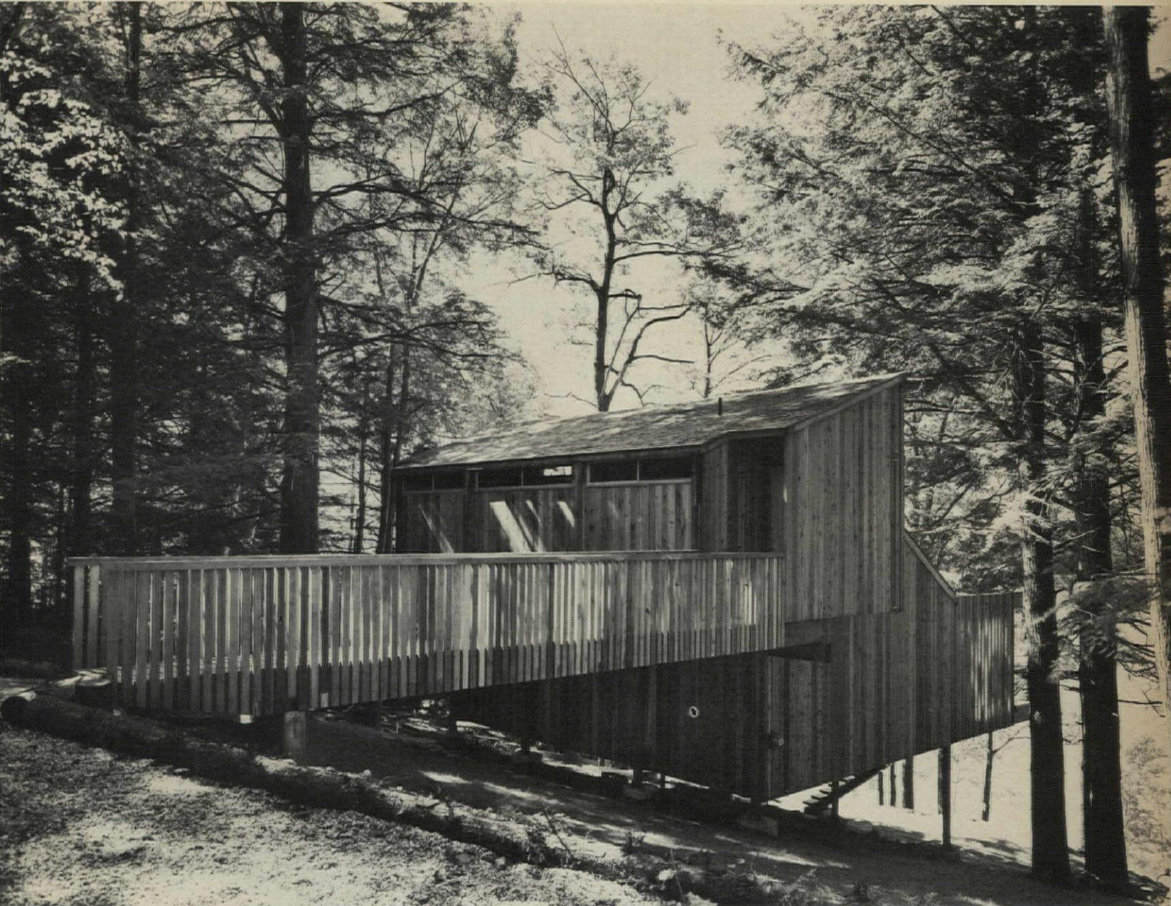
Entrance bridge leads from parking area, in foreground, to upper level (plan, below) of hillside house, which is set on piers. Side walls are blank and street windows high for privacy from nearby neighbors.
