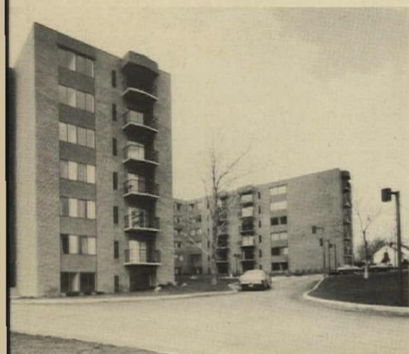
Brittain Place, another AMHA building.
