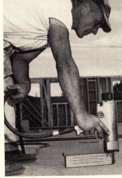
It's a pneumatic floor stapler. Or an all-purpose power stapler.
