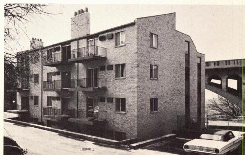
**REAR ELEVATION** shows sunken terraces. Shed roof permits clerestory windows at top level.
