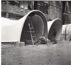
MODULES are prefabricated in a factory . . .
