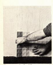
Pre-grouted tiles come in sheets of nine 41/4" x41/4" ceramic tiles that can be installed as one unit. Flexible grout permits the panels to be bent at the joints for corners or for curved surfaces. Grout strips fill between panel Amsterdam, New Circle 310 on Reader Service card
