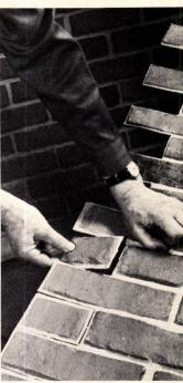
Plastic masonry now comes with selvage pretrimmed for quick installation. Half-bricks on the panel end are perforated, can be snapped off to fit two panels together in a brick-bond joint. Colonial red and colonial white. Cavrock, Vernon, Conn. Circle 313 on Reader Service card
