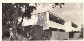
**CANTILEVERED BALCONIES**, which also shade fenced patios, are on the front facade.
