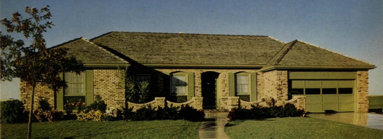
Kingsberry's "Marseille," as built by Friedrich and Sons, Inc., Ames, Iowa.
