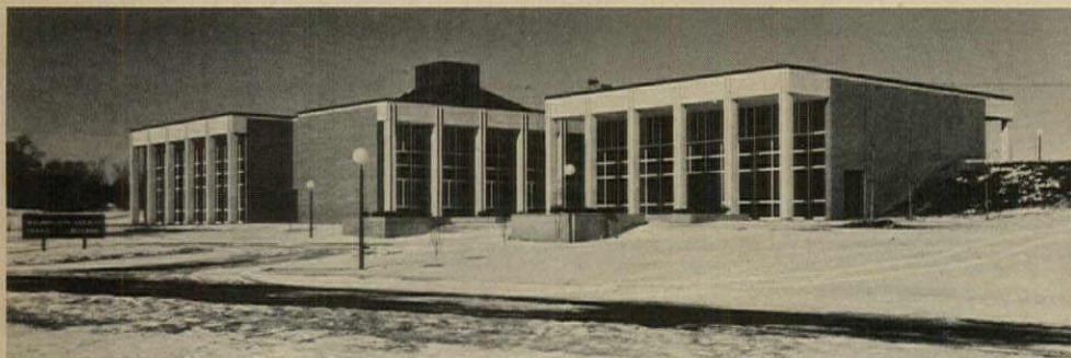
GLASS CURTAIN WALL used in two-story office building, below, was assembled with stock-size vinyl-clad window units: 3'x4' fixed sash, 4'x6' fixed sash and right- and left-hand-opening casements.
