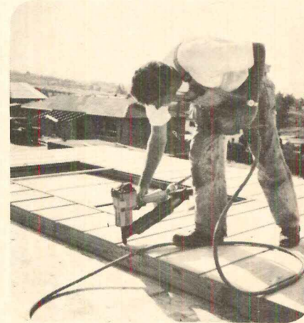
Fast on-site component construction with CN-137
