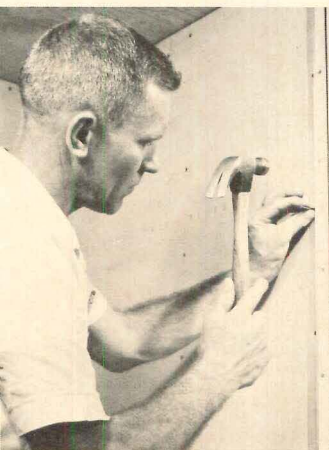
Molding base is installed . . .
