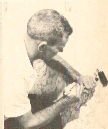
Panel is bonded.
