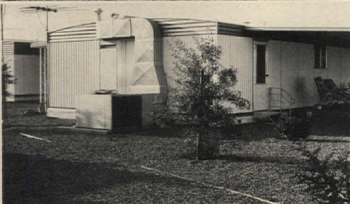
UTILITIES and heating/cooling equipment are kept out of sight at rear lot lines. To minimize maintenance, crushed stone is used as ground cover.
