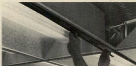
Lighting coffer clips into grid.
