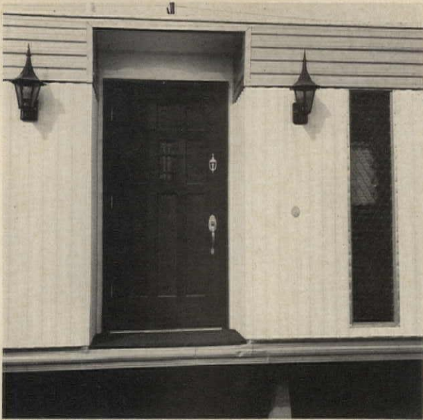
RECESSED ENTRY flanked by carriage lamps is set off by a sand-blasted wood door. Strip window is amber-colored plastic.
