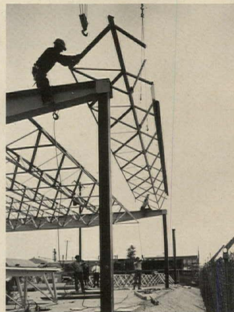
Trusses being set in place by crane.
