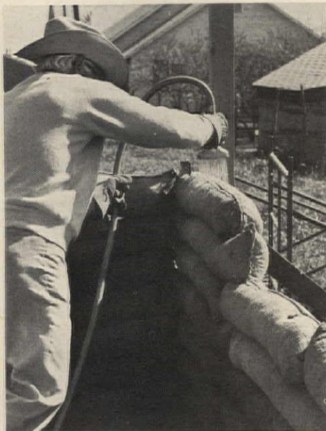
4. SOAKING with a garden sprinkler is gauged visually according to degree of sack slump.
