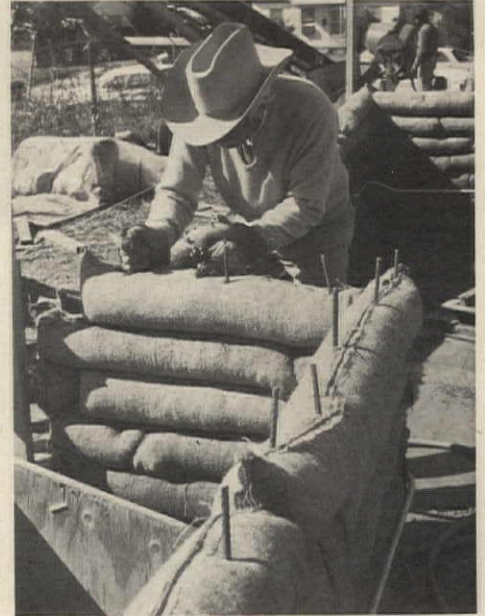
3. REINFORCING RODS —8" long, 12" o.c.—are driven between courses as sacks are laid.
