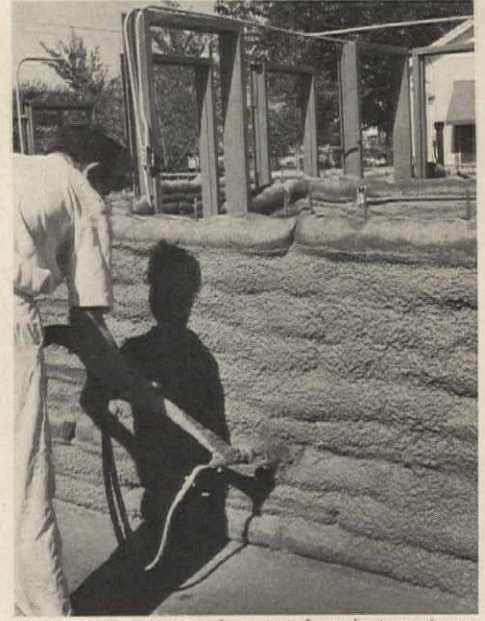
6. CEMENT FINISH is sprayed on in two stages, starting when walls are half raised.
