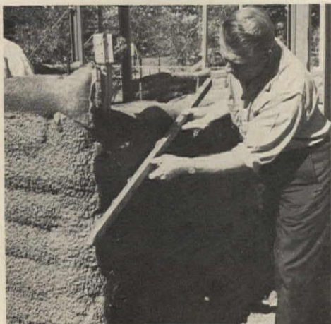
7. WALL TEXTURE can be varied from smooth to rugged according to degree of hand tooling.
