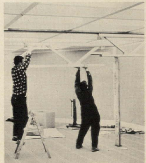
Secondary truss supports folding wall.
