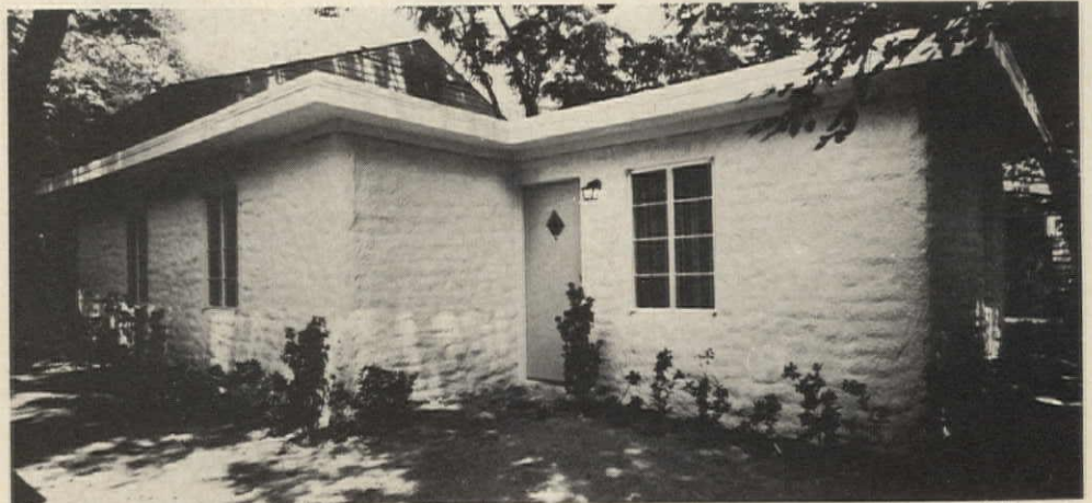
COMPLETED HOUSE has an adobe appearance, but design is unlimited. Windows and doors can
