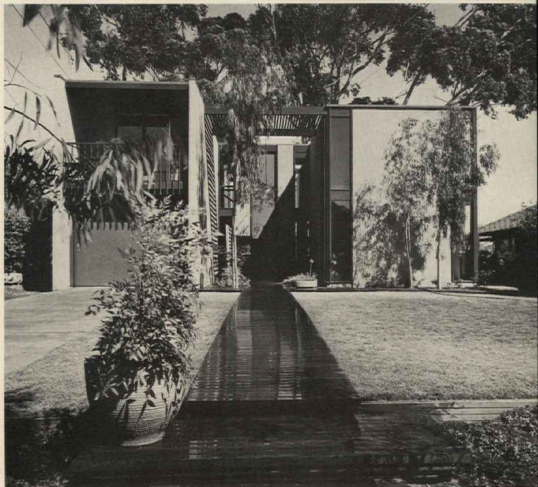
VIEW FROM STREET shows recessed entry court. One-car garage is at left, kitchen wing at right.
