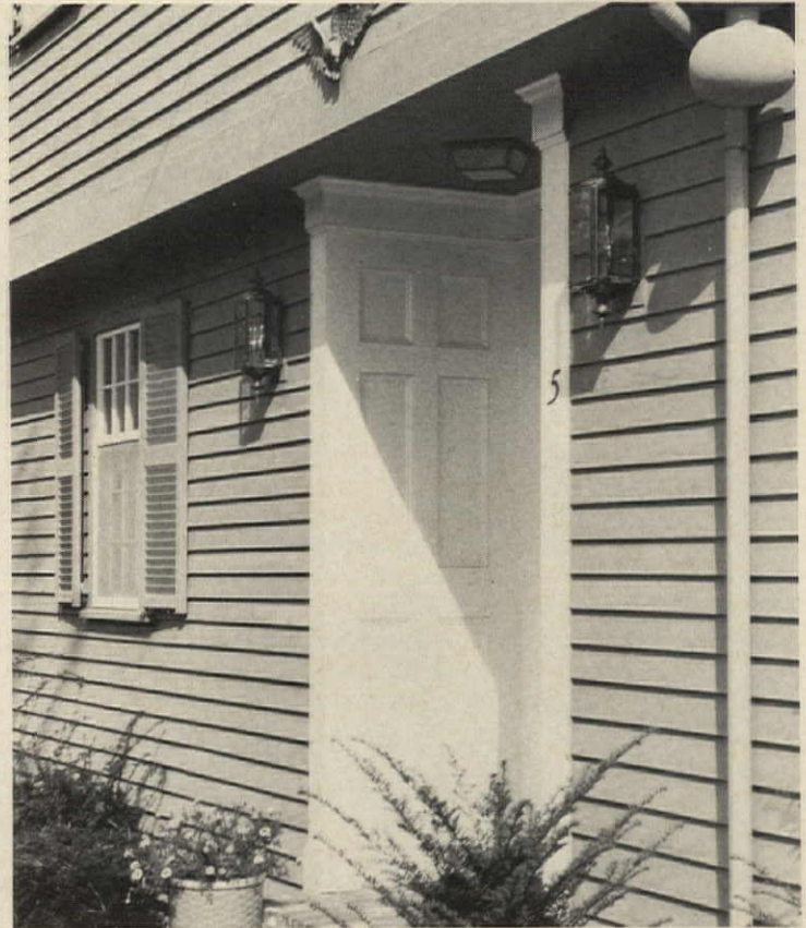
STOCK DOOR —a six-panel interior model—is nailed to the wall of a recessed entryway to avoid job-applied moldings and save finishing time.
