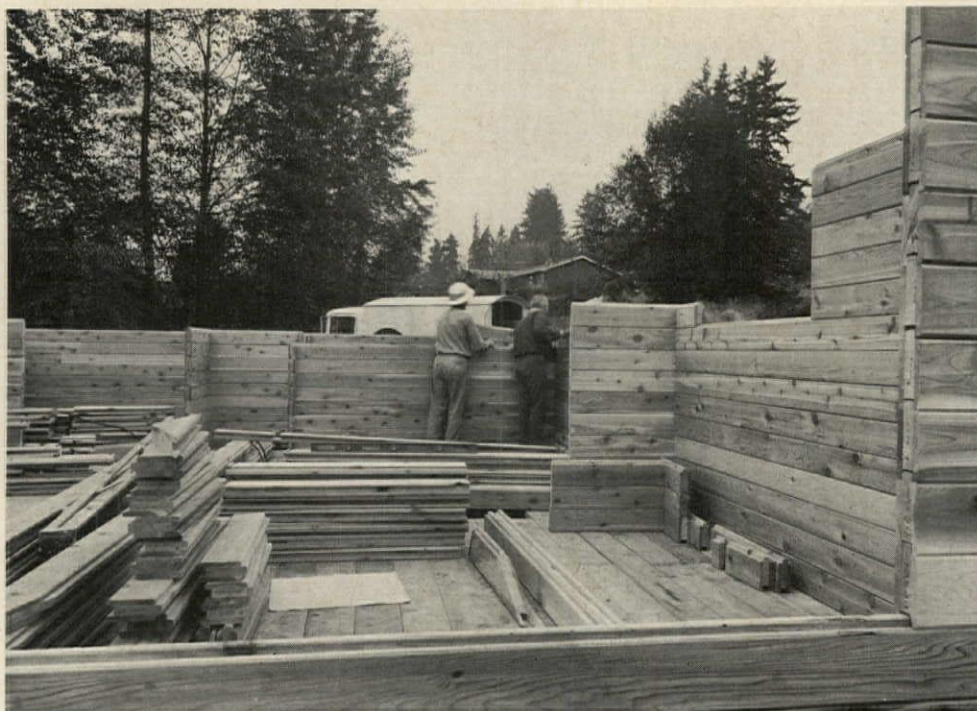
DECKING SHELL by Potlatch Forests is made of stacked-up members notched at intersections.
