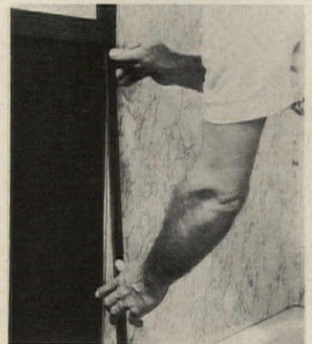
4. Press top molding into base.
