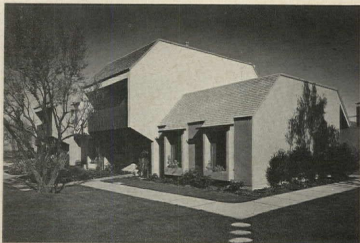
ONE-STORY UNIT on end of block follows the same roof line as the larger units. Walk leads to side entry under roof overhang at far right.
