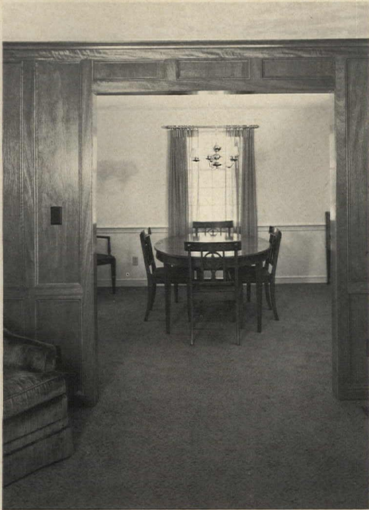
PANELED ARCHWAY —an adaptation of Linn's rail-and-stile paneling—typifies the thorough planning he puts into his interior finishing work.
