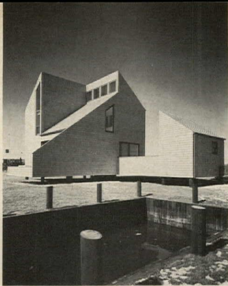
WOOD PILINGS raise house above floodwater mark. Normal level of canal shows in foreground.
