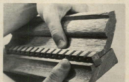
FOOLPROOF CORNICE ASSEMBLY provides a groove for locating and aligning dentil strip. Systems like this, which simplify complicated trim work, let Linn subcontract all his finishing.
