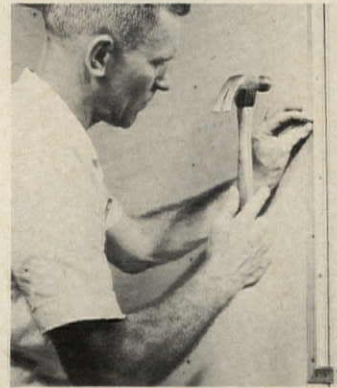
1. Nail on female molding base.
