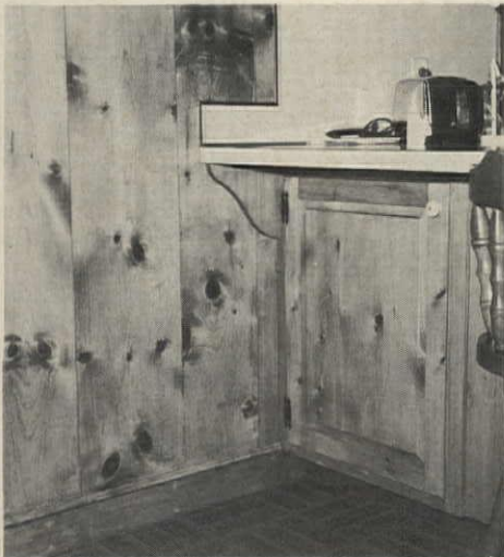
EXTRA BASE CABINET under a kitchen snack counter is another Linn standard. It makes use of dead space that is normally sealed up because
