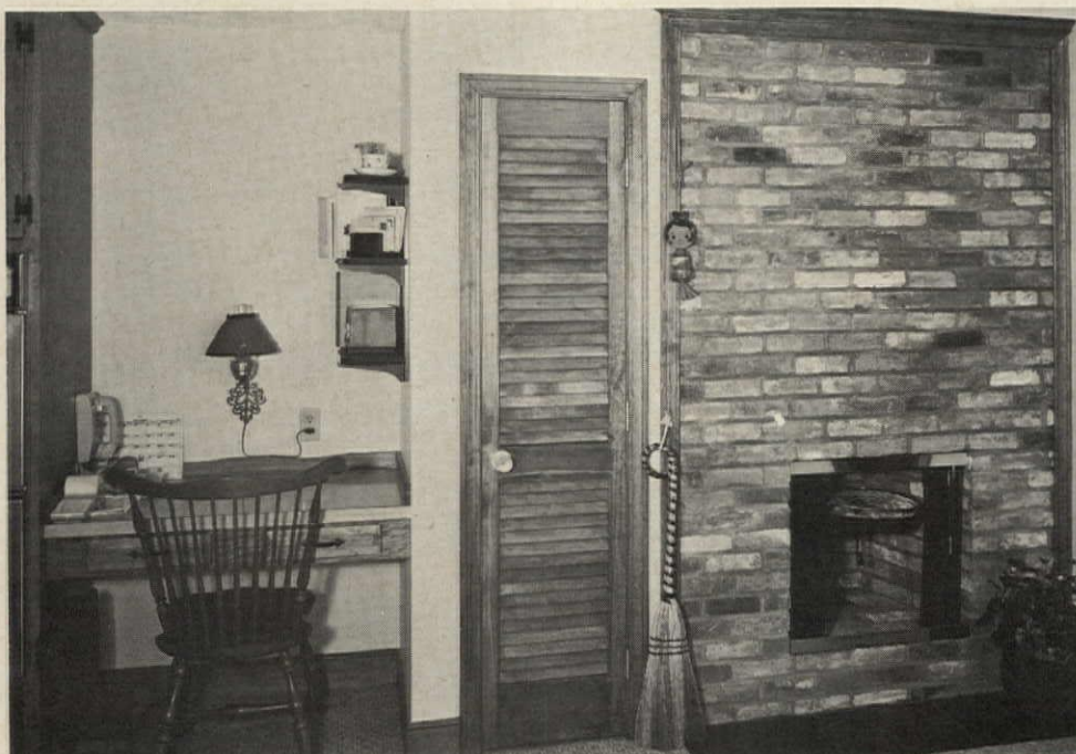
KITCHEN FIREPLACE WALL for a compact kitchen-dining area incorporates framed-in broom closet and desk nook. Linn includes a crane, for open-hearth cooking, with all kitchen fireplaces.
