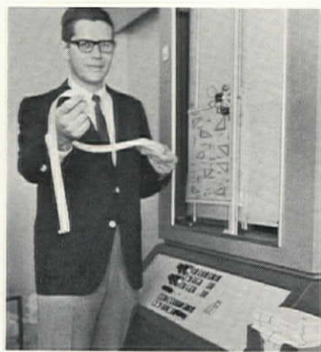
COMPUTER TAPES guide electronic plotter (left), which makes drawing of truss at designer's
