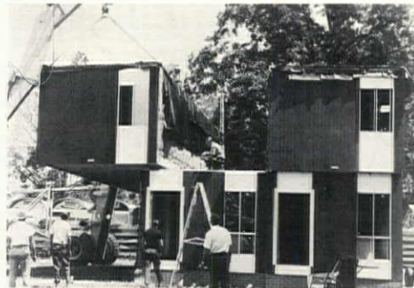
STACK-UP UNITS are positioned by a crane.
