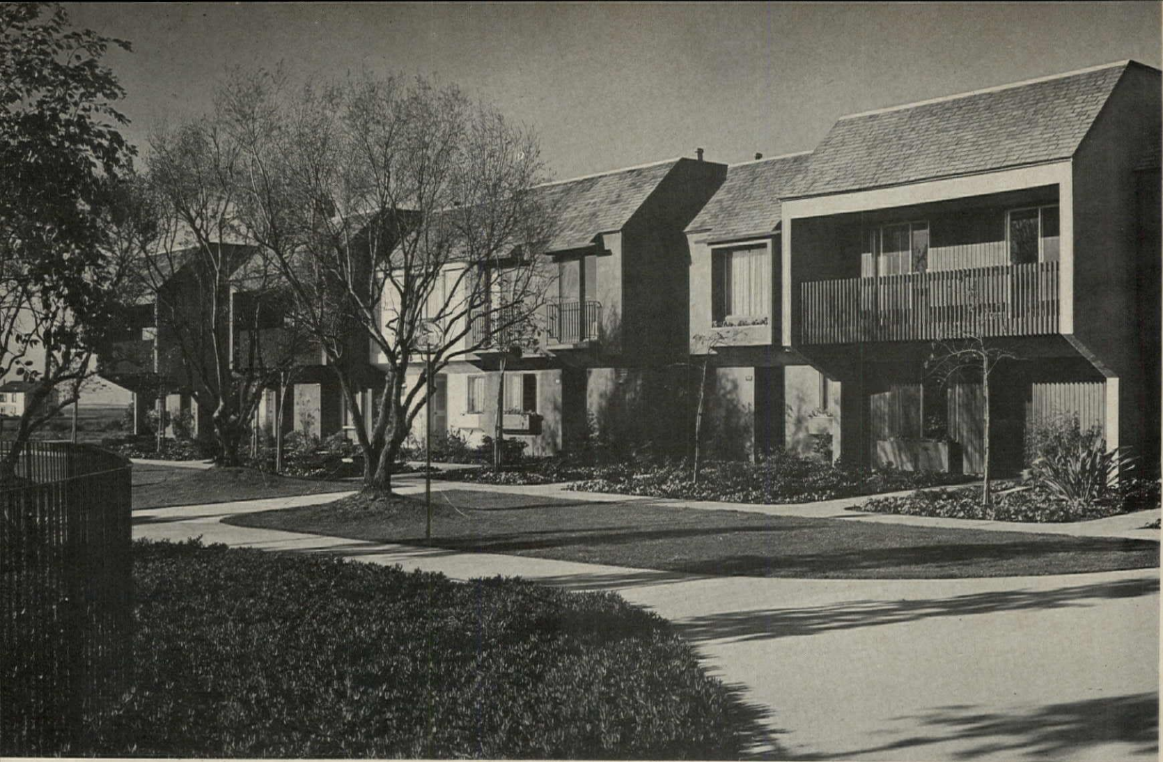
CONTINUITY OF DESIGN is apparent in this block of eight townhouses. Units appear similar at first glance, but no two of them are exactly alike.
