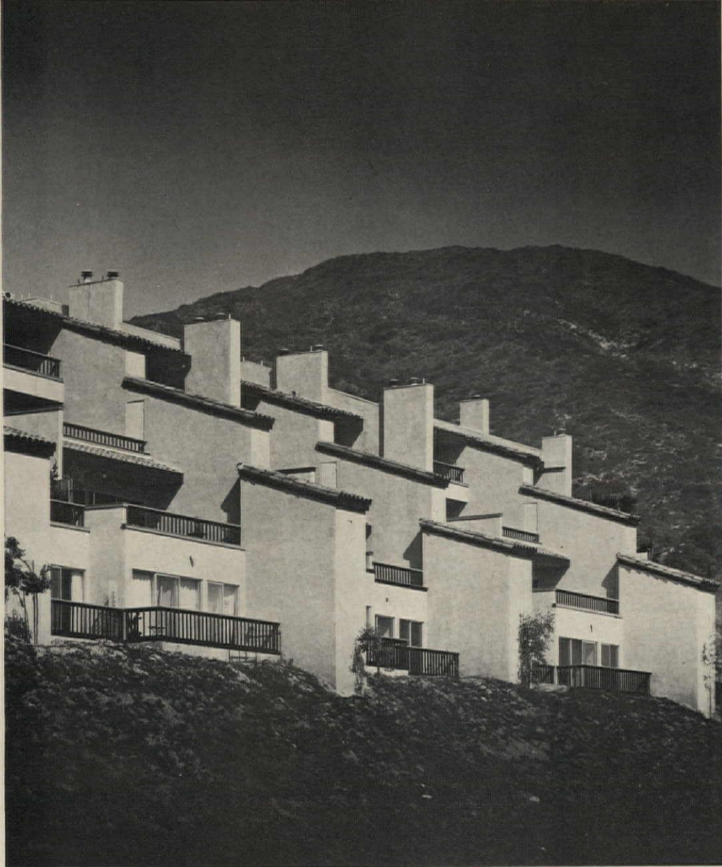
Narrow projecting walls between pairs of units enclose emergency stairways to upper units.
