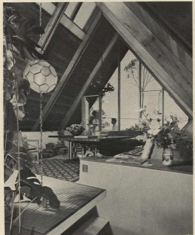
MAIN LIVING AREA of studio unit has glass gable wall that opens to deck. Additional daylight comes in through skylights at roof ridge.
