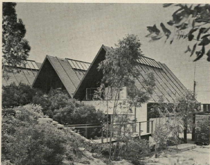
ENTRANCE BRIDGE to end unit is reached by steps leading down from parking area. It cut down grading, helped keep site in natural state.
