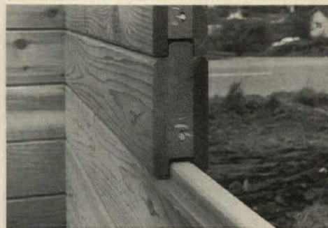
DECKING SHELL by Potlatch Forests is made of stacked-up members notched at intersections.
