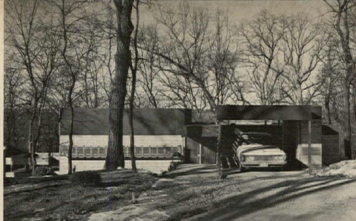
VIEW FROM STREET on uphill side shows on-grade entrance gate and carport. Horizontal strips, left, screen windows of kitchen-dining area.
