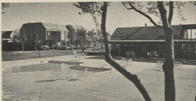
COMMUNITY AREA has two pools. Clubhouse at right contains community lounge, kitchen, shower rooms and two private meeting rooms.
