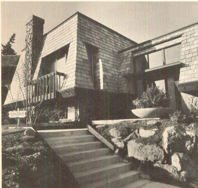
Residence, split entry (Shingles on Mansard roof) Seattle, Washington Quality Pacific Homes
