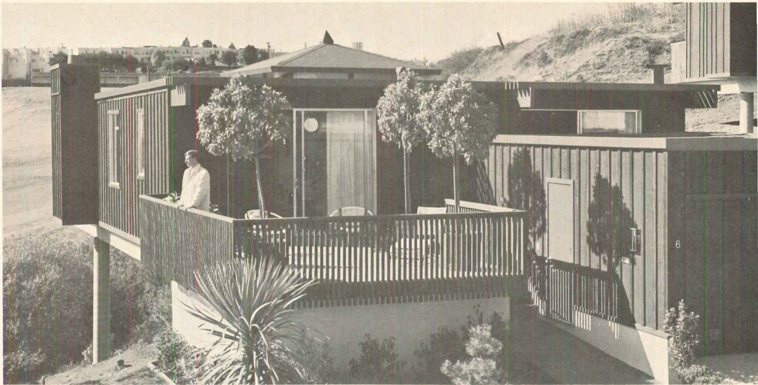
ONE-STORY HOUSE on downhill slope is supported at rear by piers. Deck is on same level as main house, garage at right is dropped about 2'.
