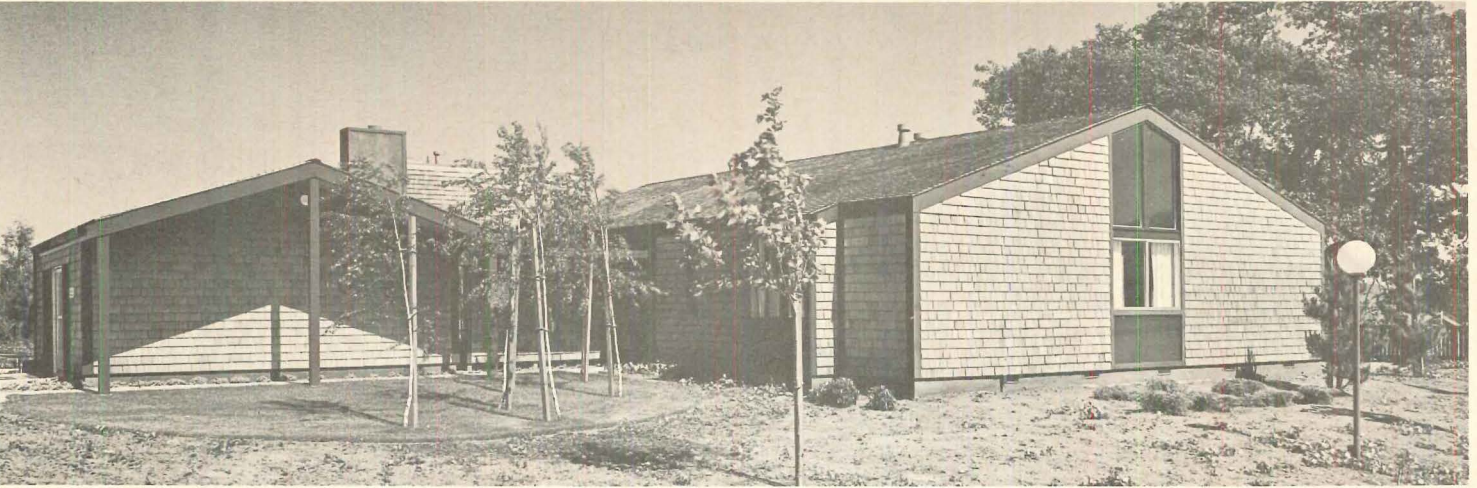
IDENTICALLY PITCHED ROOFS are used on both house and garage to maintain uniformity of design. Extended garage roof provides sheltered walk.
