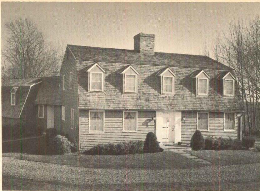
Residence, Early American (Shingles on gambrel roof) Weston, Connecticut Hearthstone Homes, Inc.
