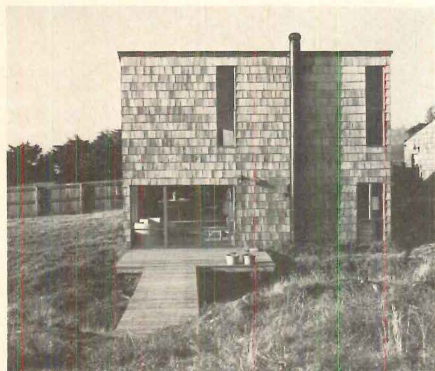
WINDOW WALL on leeward side opens to small deck. Windows above are in bedrooms.
