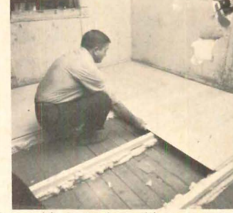
FLOOR LEVELING on rehab job was done with foam, but without new system. Jacks on screeds leveled sleepers ( top left ) until foam was applied ( top right ). After foam solidified ( bottom left ), subfloor was laid ( bottom right )
