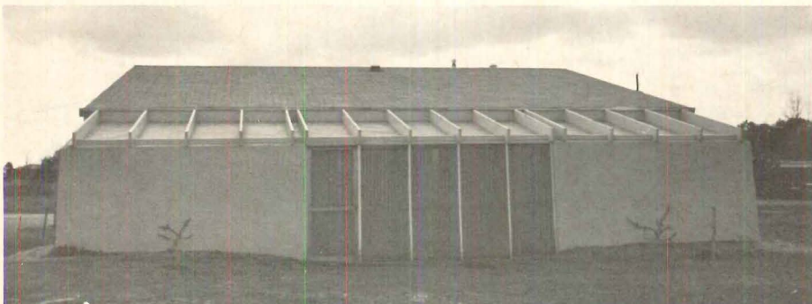
REAR WALL closes off full-width patio. Solid sections screen bedroom courts at either side (plan, above), while louvered section in center provides ventilation for the living room.
