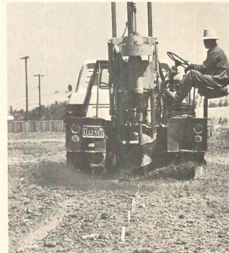
DRILLING FOUNDATION HOLE
