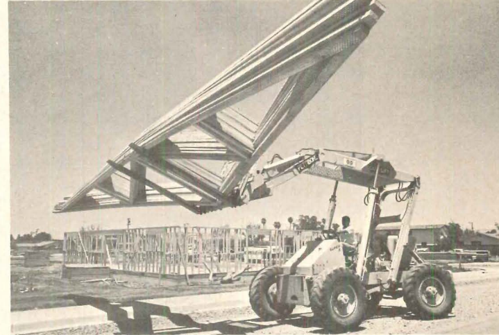
TRANSPORTING TRUSSES
