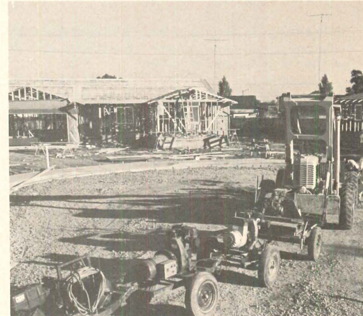
HAULING GENERATORS AND COMPRESSORS
