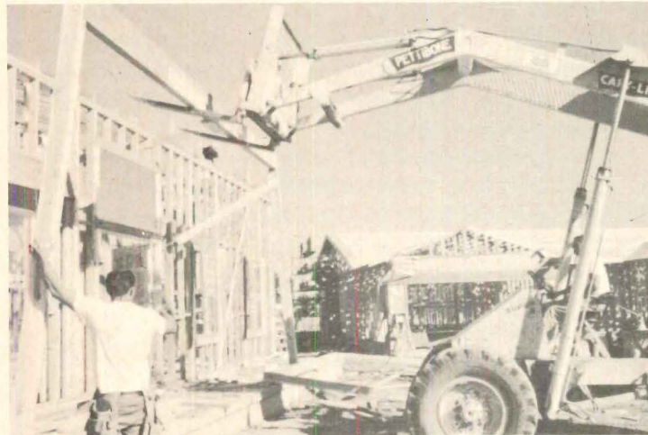
SETTING SUB-ASSEMBLED PORCH COLUMNS
