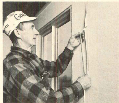
5. Remove excess vinyl strip from each flap.
