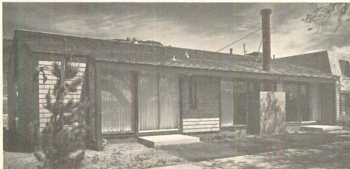
REAR ELEVATION has large areas of glass protected by short roof overhang. Sliding doors lead to master bedroom, left, living room, right.
