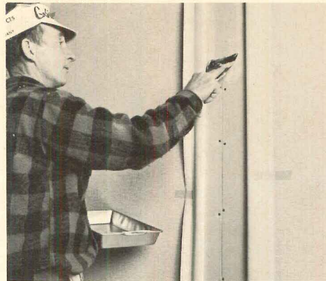
2. Apply two coats of joint compound.
