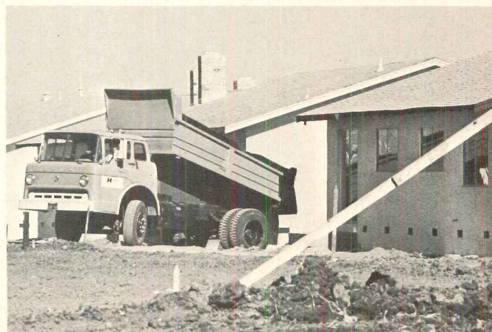
DUMPING TOPSOIL
