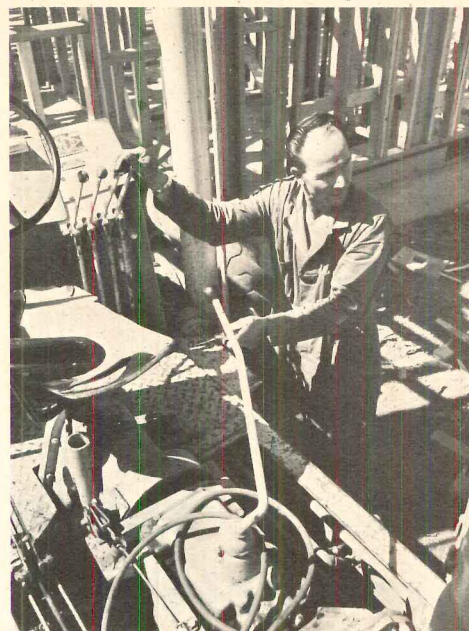
REPAIR JOB AT HOUSE SITE
