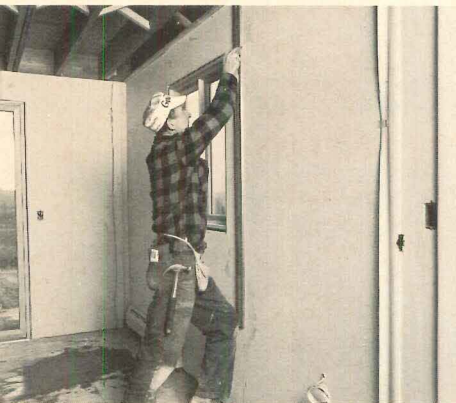
4. Cut through both vinyl flaps at one time.
