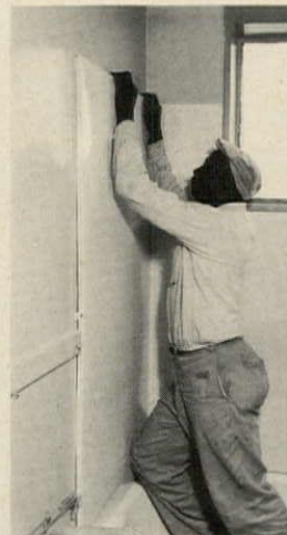
3. End-wall panel is set. Panels are forced on clips.
