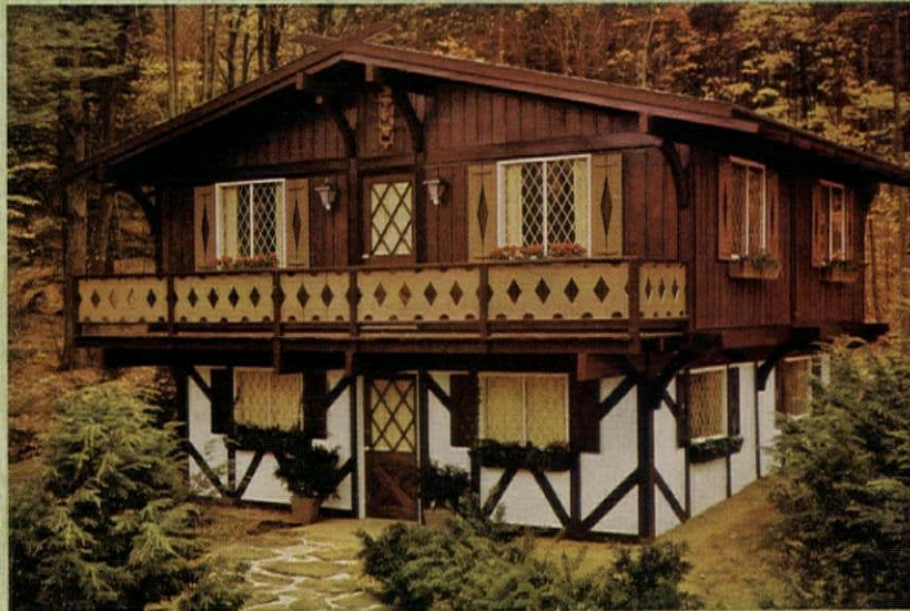
New England chalet by Stanmar Inc., Sudbury, Mass.; Architect: Robert Dion; Cabot's Stains throughout.
