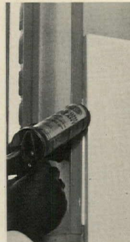
4. Silicone sealant fills all panel joints and seams.
