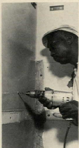
1. Zinc-coated clips are fastened to bathroom walls.
