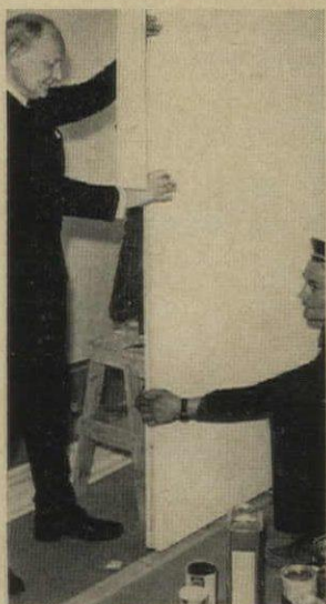
MOVABLE PARTITIONS are locked in place by plastic strip at top and expansion bolts at bottom.
