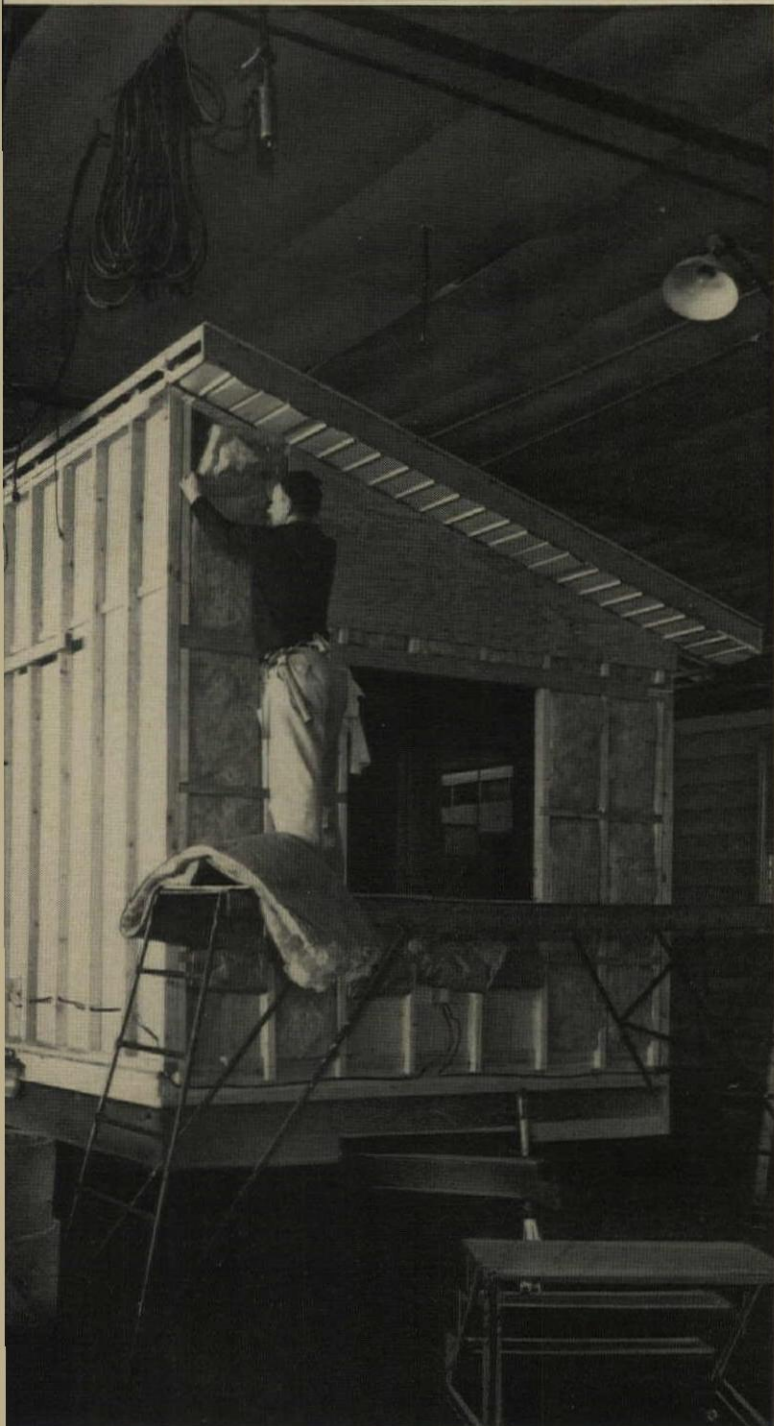
insulation in a factory-built sectional house.
