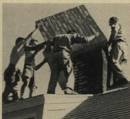
PREFABRICATED CHIMNEY-TOP made of plywood and fiberglass brick fits over old masonry chimney and doubles its size. Metal cap completes job.
