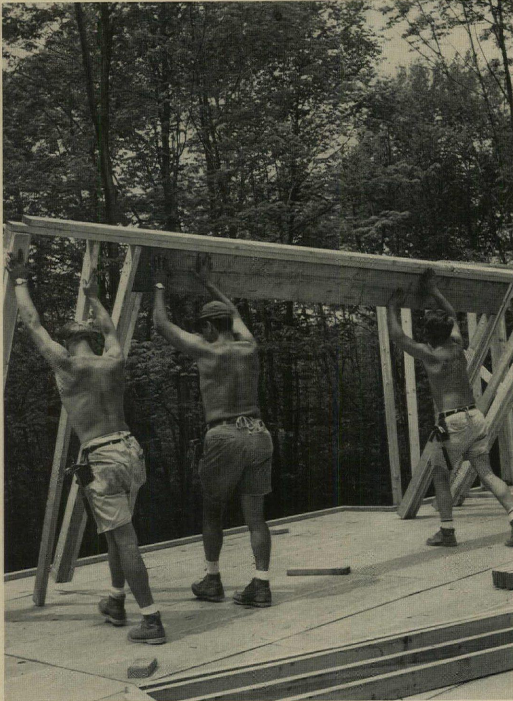
CONVENTIONAL FRAMING CREW tilts up wall on a custom-house deck.
