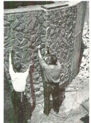
FIELD STONE fiberglass panels come in a self-blending pattern.
