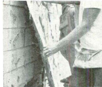
APPLYING AND FINISHING fiberglass stone involves adhesive, shingle nails and matched-color compound which can also be used to repair damage.
