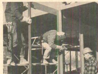
Cutout wall panels—for windows or doors—are welded at flanges.
