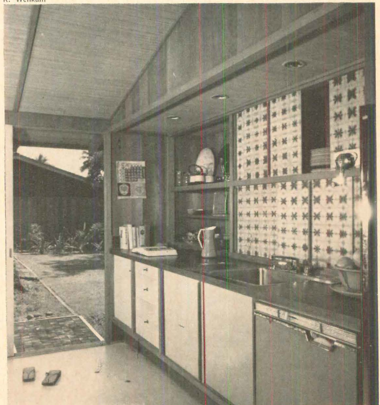
RECESSED CABINETS bring overhead storage right down to counter level. Arch.: Dennis, Whitaker & Slavsky. Location: Hawaii.
