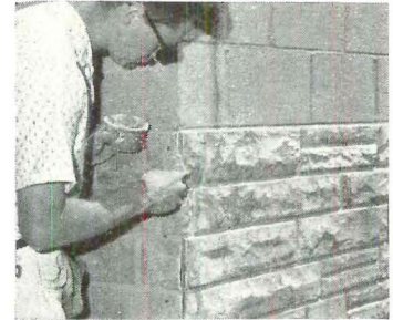
APPLYING AND FINISHING fiberglass stone involves adhesive, shingle nails and matched-color compound which can also be used to repair damage.
