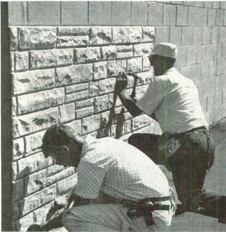
CUTTING AND FITTING panels of fiberglass split-face stone is done with a carbide-tipped saw and finger-joints formed by removing end stones.
