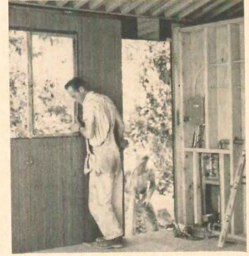
Sandwich-panel walls are prefinished skins glued to polystyrene.
