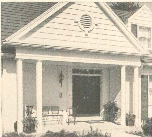
Four extruded aluminum columns add classic beauty to this custom home. The 8" aluminum siding with long lasting Colorweld® finish gives years of service and beauty without repainting.
