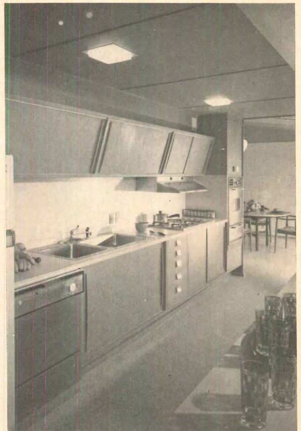
SLANTED CABINETS make top shelf easy to reach because narrow bottom shelf isn't in the way. Builder: Kaiser Ind. Location: Hawaii.
