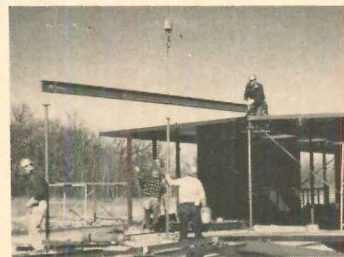
Standard steel beams and columns are used for center bearing wall.
