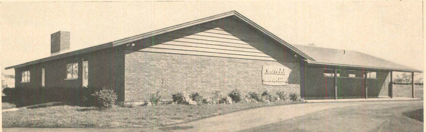
RECREATION CENTER at Scottsdale combines function of civic center and clubhouse. Place & Co., South Bend, built the entire complex, including pool, for $120,000.
