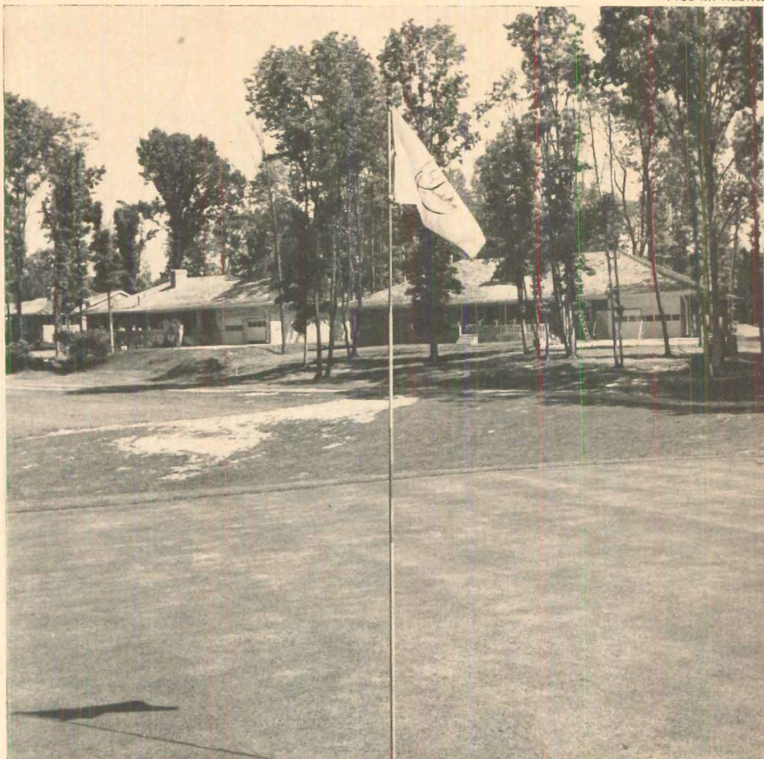
FAIRWAY HOUSE LOTS at Tantallon in Maryland bring 25% to 50% more than off-course sites. Prestwick, Inc., the developer, has 200 sites around its 135-acre course.
