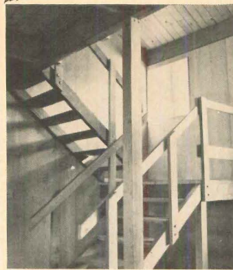
All-wood interior is provided by exposed surfaces of load-bearing decking.
