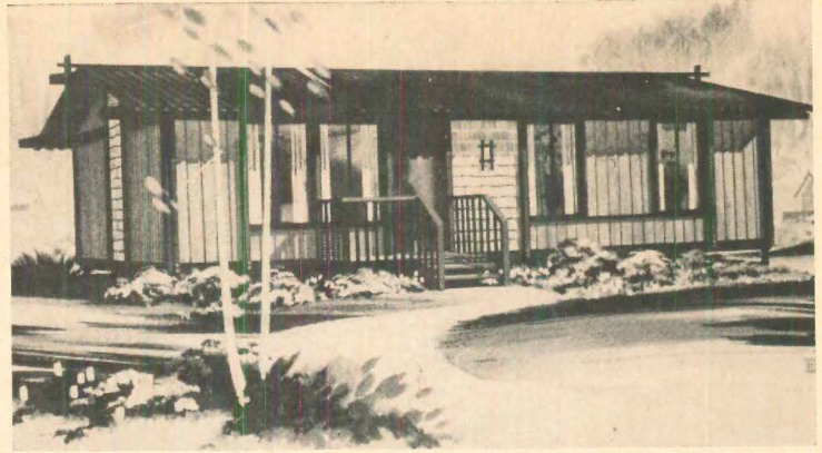
Exposed posts and beam ends serve as trim highlights in exterior design.
