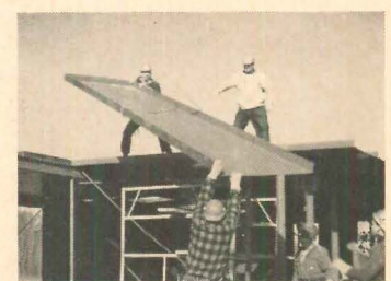
Lightweight roof panel is welded to adjoining roof and wall panels.
