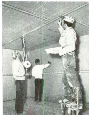
SINGLE-LAYER RADIANT DRYWALL goes up just like any other drywall job. Advantage in winter: Heat can be turned on before joints are taped.
