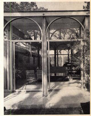
Decorative arches set within the 6' module of the steel frame appear at either end of the 30' living-music room (view E). I-beams form the columns and bent channels the arches.
