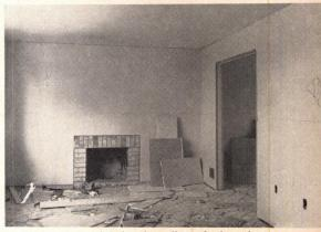
LONG SHEETS minimize drywall cracks by minimizing seams. Henry stocks the longest sheets he can buy (14'), uses them wherever possible.
