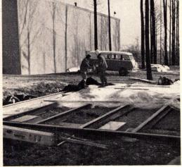
REGISTER DUCTS are hooked to main duct through footing knockouts before subfloor is fastened down.
