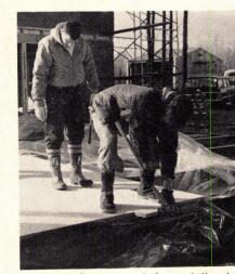
PLYWOOD SUBFLOOR is fastened directly to I-beams. A heavier floor panel may permit 5' joist spacing.
