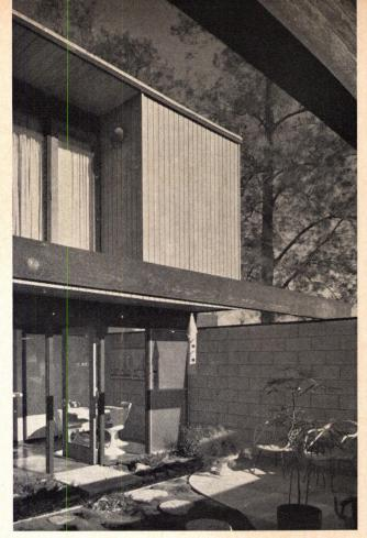
A glass wall opens the entire rear of the lower-level living area to the inner courtyard (view C). The upper level also has a glass wall which is recessed 3' behind the master bedroom balcony. Solid section houses a closet.
