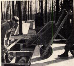
FOOTING POUR ties pre-leveled steel joists into footings. Reinforcing rods are hooked to beam flanges.
