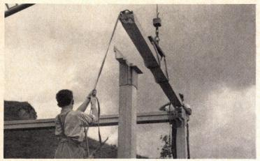
FRAMING for panels is concrete columns and beams poured in plastic forms.
