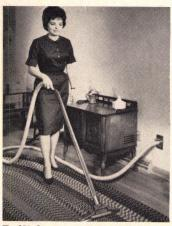
Built-in vacuum cleaner, called Vacu-Flo, has a plug-in hose connected to tubing in the walls. Tubing funnels dirt and dust to large receptacle that can be located in the garage, basement or utility room. H-P Products, Louisville, Ohio.
