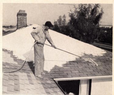
**Plastic roofing** is said to prevent wind lifting damage to composition shingles and loss of granules and weathering of asphalt shingles. Permalume Titanium can be applied with rollers, brushes or sprays. Permalume Plastics, Vancouver, Wash. *Circle 238 on Reader Service card*.
