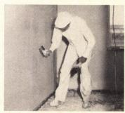
Wall system has a pre-catalyzed gypsum base that requires one coat of high-density plaster. Pabcoat is completely cured in 24 hours so paint or wallpaper can be applied the next day. Fibreboard Paper Products, San Francisco.
