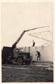
Hydraulic crane extends to 36' and will lift up to 650 lbs. to 44' height. Truck-mounted unit will also lift up to 1,460 lbs. within a 6' to 22' boom radius. Boom folds forward over cab or backward over load. Hiab Hydraulics, Wilmington, Del. Circle 233 on Reader Service card
