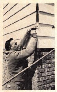
**Steel siding** is coated with zinc for additional protection. The siding resists denting and hail damage and does not require backer board, according to the manufacturer. Siding is applied with ordinary tools. Aluminsteel Corp., Hammond, Ind.
