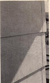
Rough sawn siding, which takes paint or stain, comes in lap (above) plain or grooved types. Ruf-X-Ninety has a tenyear guarantee on the surface finish and a 25-year guarantee against exposure damage or defects. Masonite, Chicago.
