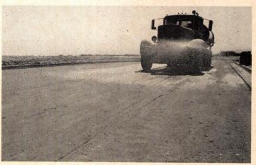
**8.** Fogging provides the moisture required in cement-treated road base. After cement-and-sand windrows are shaped down by a grader, the mixture is compacted by a 12-ton roller, then a 30-ton roller, with fogging in between.
