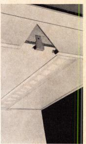
Soffit system, called Vinyl-Bond, includes panels, three color-matched metal accessories and a louvered venting strip. The wall angle and fascia cover are said to simpify installation. Soffit system does not require painting. Insulite, Minneapolis.
