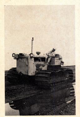
Crawler tractor with extra-wide track shoes squeezes water from newly placed hydraulic fill before big scrapers move in for final grading.
