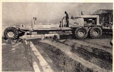
**7.** Cement is mixed directly into roadbed soil by windrowing, forming a 5" to 7" base for all streets and boulevards. High-quality sand fill makes this possible, saving \$600,000-worth of trucking in aggregate for rock base.
