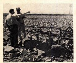
1. Plowing is followed by disking, with a drying period after each. This strengthens muddy soil so scrapers can make cuts in it.
