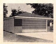
Garage door has six sections. Straight track door has pinchproof joints, recessed lock handle and a continuous interlocking hinge. The units are factory finished and available in all standard sizes. Taylor Garage Doors, Detroit.
