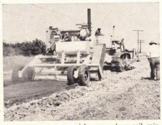
MIXER/PULVERIZER picks up roadway soil, mixes in lime, redeposits it at speed of 1½ mph.
