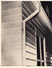
**Gutters and siding** are made of vinyl that will not chip, corrode, blister or peel, says the manufacturer. Material does not require painting and won't burn or conduct electricity. Siding and gutters are guaranteed for 20 years. Monsanto, St. Louis.
