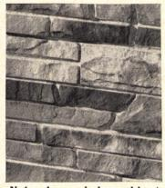
Natural-quarried marble is less expensive because of the installation process. A 3.5 wire lathe nailed to existing surface is the base f r application with concrete. A variety of shades are available. International Stone, Franklin Square, N.Y.
