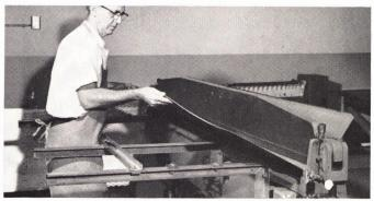
**POWER BREAK** is one of three 8' machines to permit prefabricating of standard 8'-long duct.
