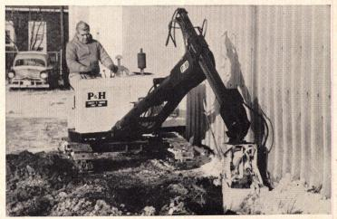
**Small excavator** has 2-cu.-ft. all-position bucket, a low silhouette and only 3.7 psi ground pressure which permits it to be used to dig beside existing buildings. It can dig to a depth of 11 ft. Harnischfeger, Milwaukee. (*Circle 227 on Reader Service card*)
