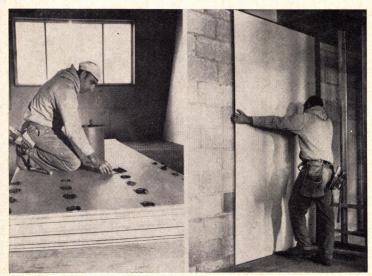
**Wallboard adhesive** is designed for trowel or spotting application of foamed plastics, plasterboard, plywood and other decorative paneling in above-grade installations. No clamps, braces or nails are used. Armstrong Cork, Lancaster, Pa. (Circle 221 on Reader Service card)
