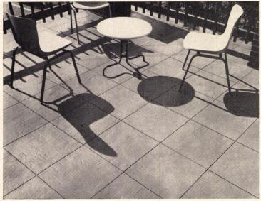
**Exterior deck surfacing** is made up of a waterproof, elastic base sheet bonded to the deck and a surface of resilient tile. Decking is said to be completely watertight. Cost: \$2 to \$2.50 a sq. ft. including labor. Armstrong, Lancaster, Pa. (Circle 231 on Reader Service card)
