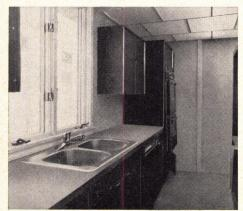
**LUMINOUS CEILING** of 2'x2' panels is suspended directly from trusses on 2' centers.
