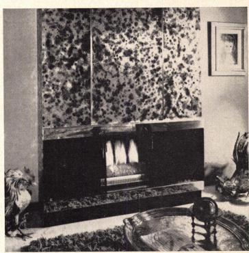
**Gas fireplace** has remote push-button control. Seven models are available, including a custom model with a variety of facing materials. Installation takes an hour and costs half as much as masonry fireplaces. Dyna Mfg., Los Angeles (*Circle 239 on Reader Service card*)
