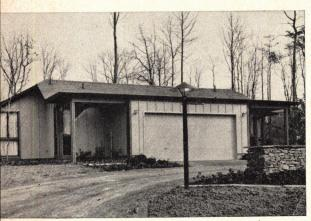
FRONT ELEVATION projects 8' to give garage adequate depth. Entry is set back at right.
