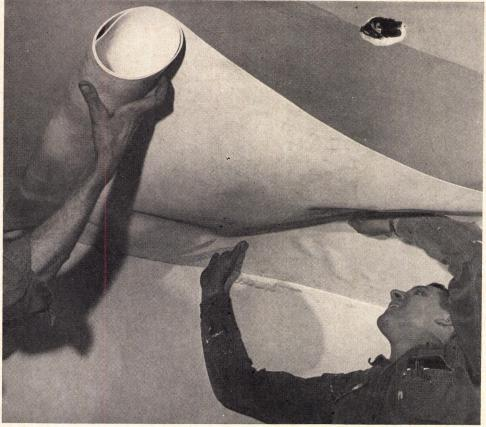
MASTIC COATING bonds radiant vinyl to ceiling. Bubbles are smoothed out with long-handled roller.
