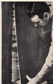
**Panel adhesive** is said to make installation of plywood paneling 50% faster than with nailing. Consistency of adhesive allows ample time to move panels into perfect alignment before final bonding. U.S. Plywood, New York City. (Circle 215 on Reader Service card)
