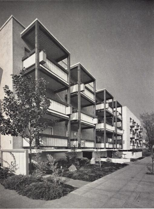
**PRIVATE BALCONIES** are supported by cantilevered slab which forms first floor of building.
