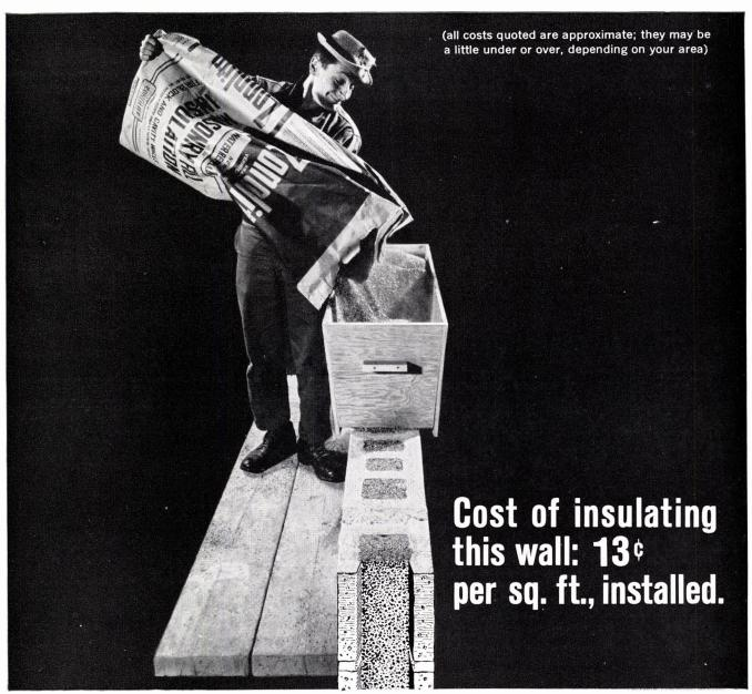
Simply pour water repellent Zonolite\* Masonry Fill Insulation into the cores of this 8" block.
