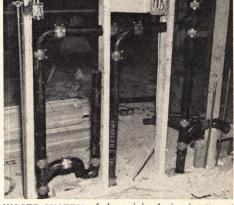
**WASTE SYSTEM** of sleeve-joined pipe is attempt to make plumbing layout more flexible.
