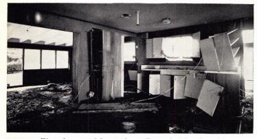
BEFORE: Water has staved in exterior wall, wrecked interior cabinets.
