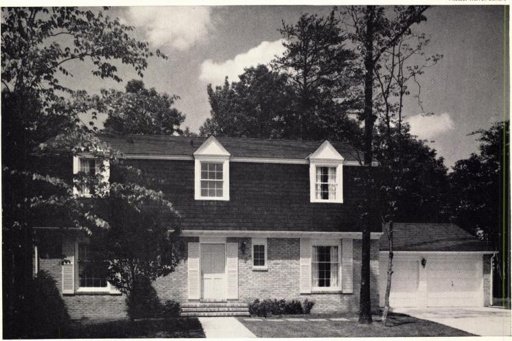
**FRONT ELEVATION** is clean and well balanced. Lower plane of gambrel roof is actually the front wall built out with falsework (see plan).
