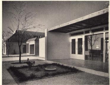
**ENTRY TERRACE** has deep roof overhang. Walls are masonry block with stucco finish.
