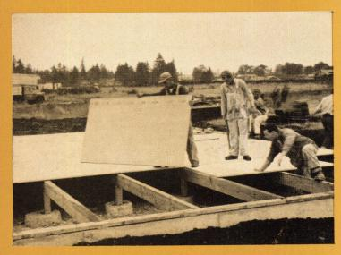
**1.** Foundation was poured the day before. Plywood floor on this model is 2.4.1, the 11/8-in.-thick combination subfloor-underlayment, with supports on 4-ft. centers.
