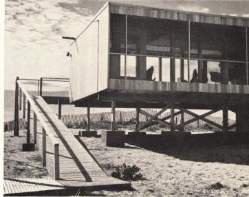
**SIMPLE FOUNDATION** consists of piers and posts. Cross-bracing resists racking stress.
