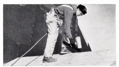
**POWER FASTENER**, used after all panels were positioned and tacked, saved one hour of labor on 2,000-sq.-ft. roof compared with hand nailing.
