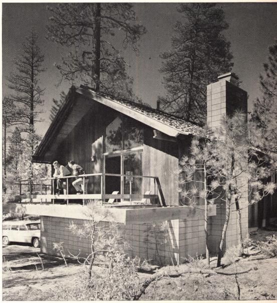
**GABLE ELEVATION** has deep roof overhang and deck supported by cantilevered 4x6 girders.
