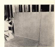
Sound-deadening board is gypsum board with a polystyrene foam-paper laminate. Silent-Cor is only ½" thick, yet reduces noise as effectively as many thicker materials. Wallboard can be nailed directly to studs. Monsanto, St. Louis.
