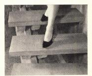
Nonskid surface material has a plastic-impregnated, waffle-patterned overlay on plywood. This easily installed material comes in natural tan, brown or black. Panels 4' x 8' are priced at 50¢ to 55¢ a sq. ft. Simpson Timber, Seattle.
