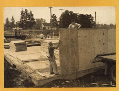
**3.** Wall components for this M/P model have plywood sheathing on studs; siding will be applied later. Components are stacked on the floor platform near where they'll be used.
