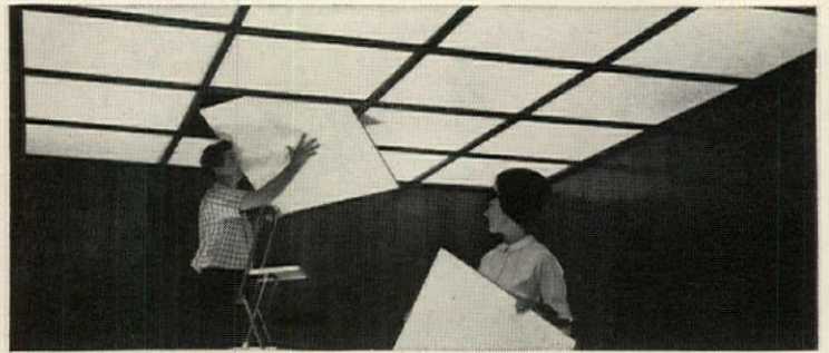
Acoustical ceiling with metal suspension system has wood-finish grids 1\frac{3}{4} " wide that extend 1" below the panels to look like beams. Glass fiber acoustical panels and translucent lighting panels are 3'x3'. Gustin-Bacon, Kansas City. (For details, check No. 28 on p. 209)
