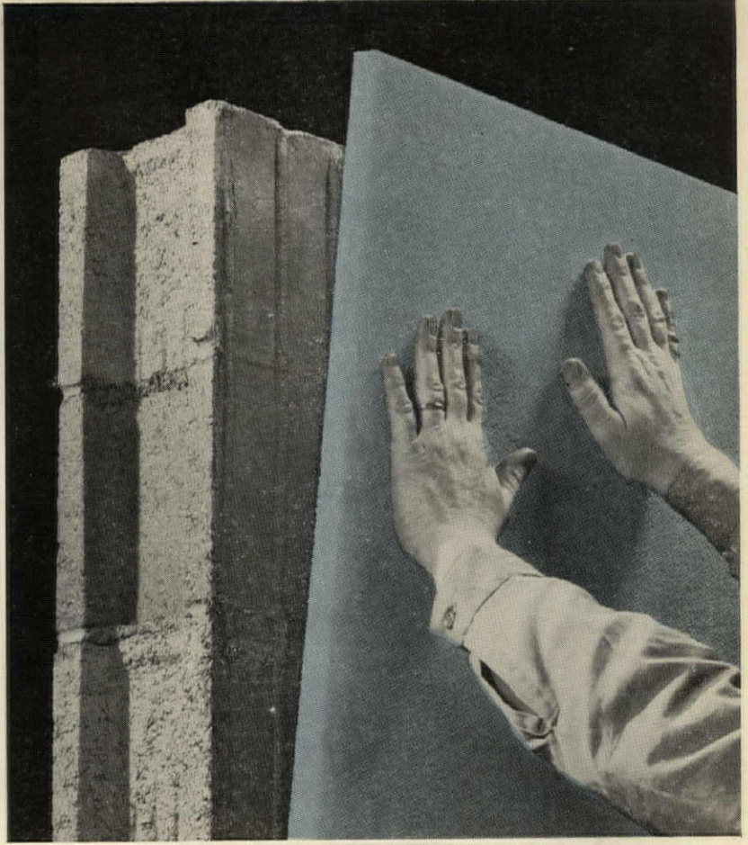
4. Press Styrofoam FR into place. It installs fast, resists heat transfer, stays dry for year-round comfort.
