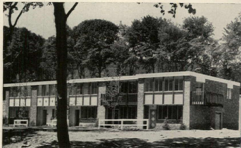
FRONT ELEVATION of a townhouse group shows the broad glass areas on both levels. Balconies were spotted for esthetic effect. There are nine styles of fronts and 27 floor plans. Each floor is roughly 20'x37'.
