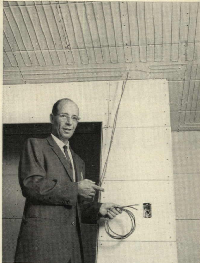
"ELECTRIC CEILING CABLE offers a lot of advantages to a builder," says Henry Motycki. "It's efficient, fast and easy to install, and takes up no space at all. It's dependable, too—literally the only thing that can wear out is the thermostat."
