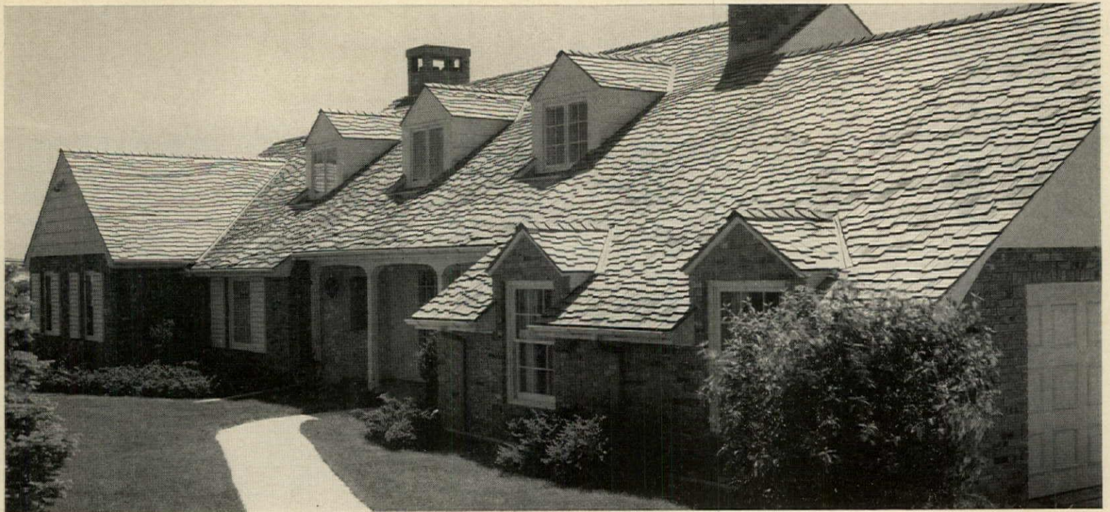
"Thatch" application. Residence, Kansas City, Missouri / Architect: John Hyde, Jr. / Contractor: Harry V. Peterson
