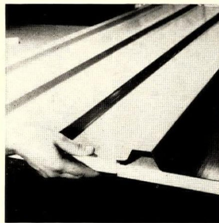
URETHANE FOAM CORE of panel is bonded to enameled steel skins on both sides.
