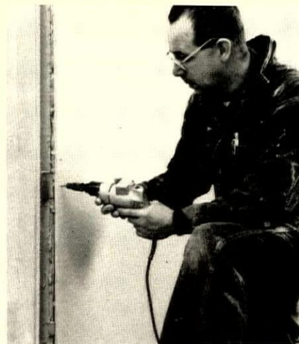
6. SELF-TAPPING SCREWS secure skin to screw plates and floor and ceiling channels.
