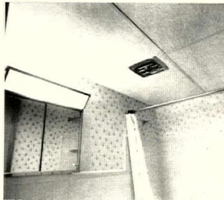
BRIGHTER LIGHTING and a ceiling with acoustical and thermal insulation are being tried in bathrooms of experimental models.
