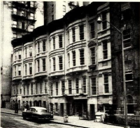
STOOPS VANISH AFTER RENOVATION
