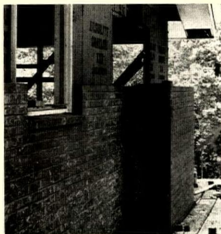
5 Chimneys outside the house eliminate delays and cut costs. Inside chimneys would cause schedule conflicts between carpenters and masons, require separate footings and special fireproofing of adjacent woodwork, and use costly inside space.
