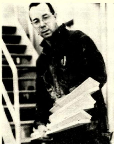
1. FOLDED GYPSUM STUDS are scored at factory, folded into delta shape at site.
