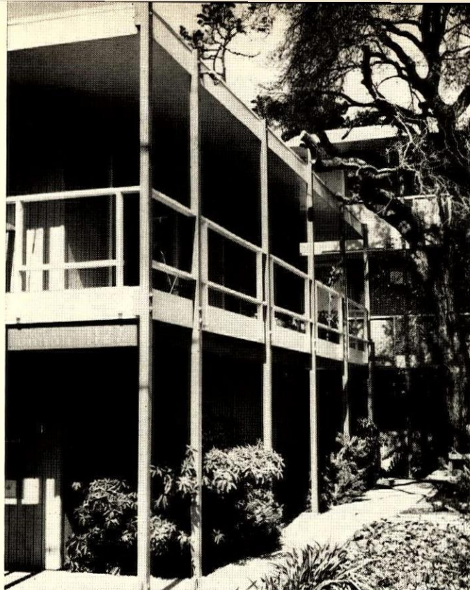
TRIM, WOOD-FRAME BUILDING has two-story wing on street, three-story wing (with eight of the nine apartments) at rear of the site.
