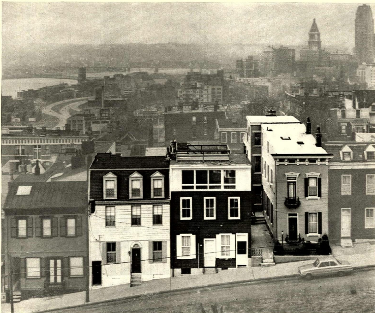
REMODELED HOUSES have rear view of the Ohio River. Raised roof on center house turned a low attic into attractive living space (see p 123).
