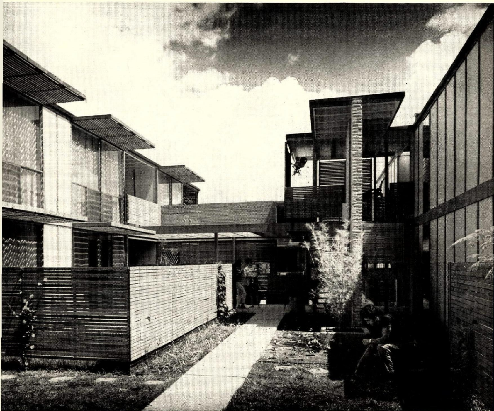
TWO-STORY UNITS have cement-asbestos exterior walls, with redwood battens. Screens enclose patios and shade big glass areas of apartments on both floors.
