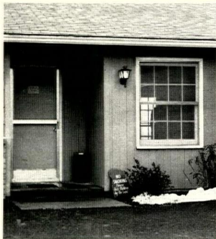
FRONT SCREEN DOOR should be screened full length, buyers say, and should be made of aluminum rather than of painted wood.
