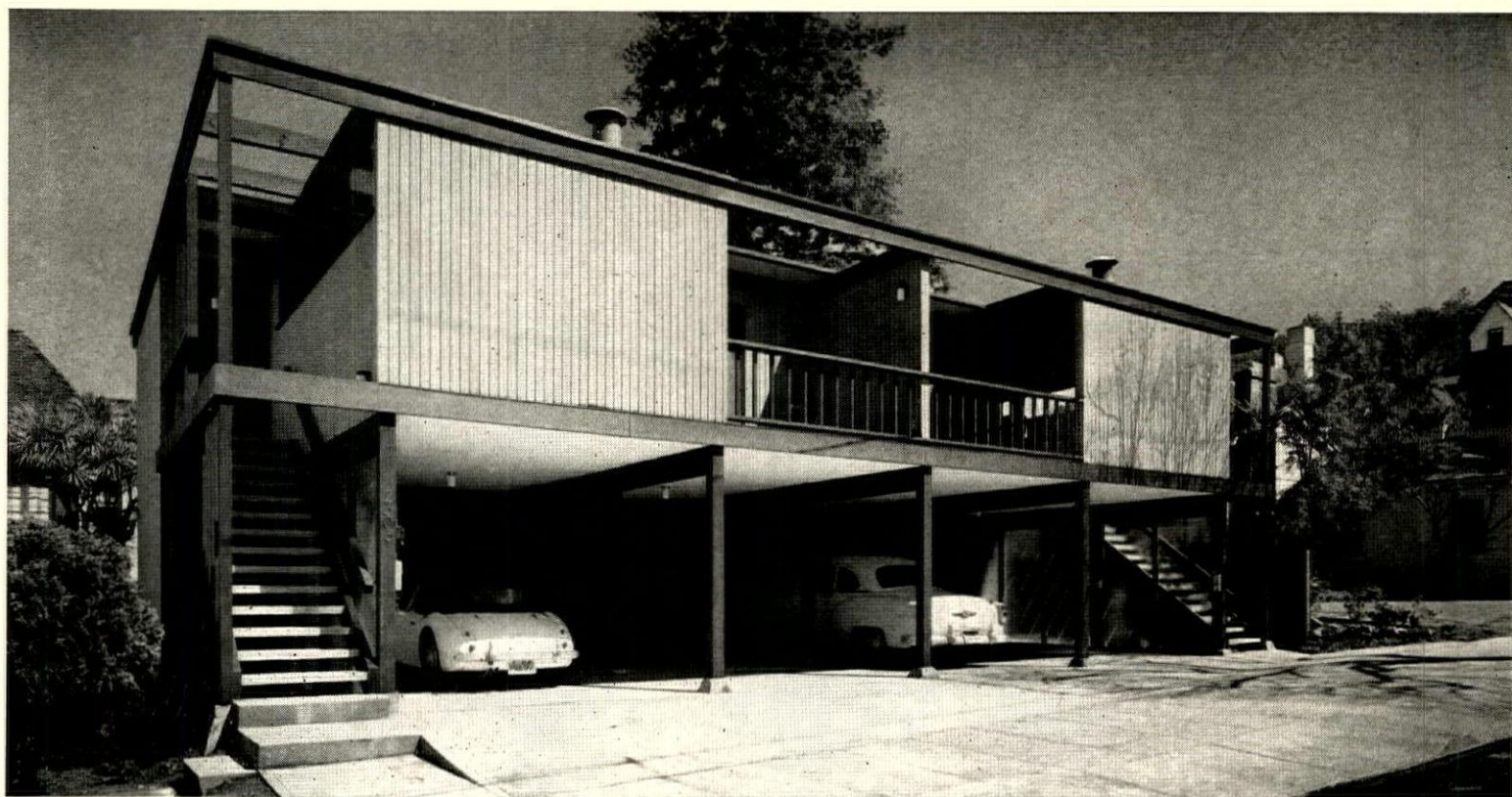
POST-&BEAM CONSTRUCTION has clean strong lines. Open-tread stairs at both sides add to balanced design, and different textures add interest.
