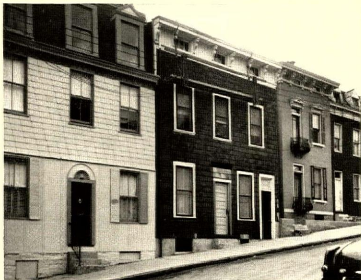
BEFORE REMODELING the three houses had weathered exteriors, generally run-down appearance. Note low top windows in attic of center house.
