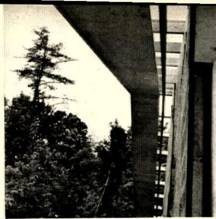
8 Overhang at gable end is formed by a prefabbed ladder panel. It rests on a special gable-end truss with a top chord 3\frac{5}{8} " lower than other trusses. It is also fastened to the first truss in from the end. Open strip in soffit is screened before installation, provides attic ventilation.
