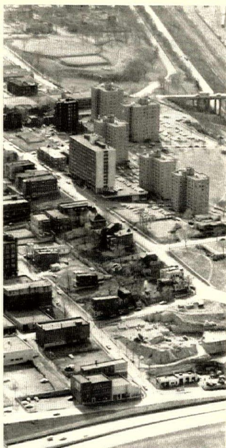
STRIP OF BLIGHT in foreground helped slow rentals in rectangular 11-story apartment (far left among the six high-rises). Slums will fall this autumn for a Hilton Hotel.
