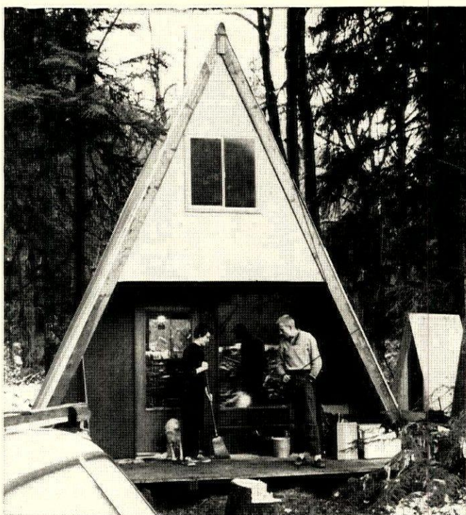
LUMBER DEALER'S MODEL is made by Sandpoint Builders Supply of Seattle, sells for $2,295 plus erection. Floors, end walls, and roof are made of panels trucked to site. Upstairs sleeping deck is 9' x 12'.
