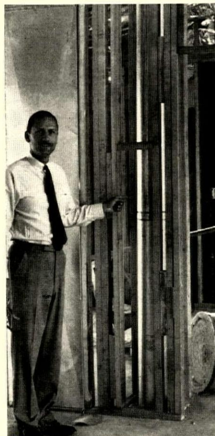
9 Kitchen-fan ductwork is run up between wall studs. This not only saves cabinet space (item 4, p 154) but since it can be installed at the same time as furnace ducts, it eliminates a separate trip for the tinsmith.
