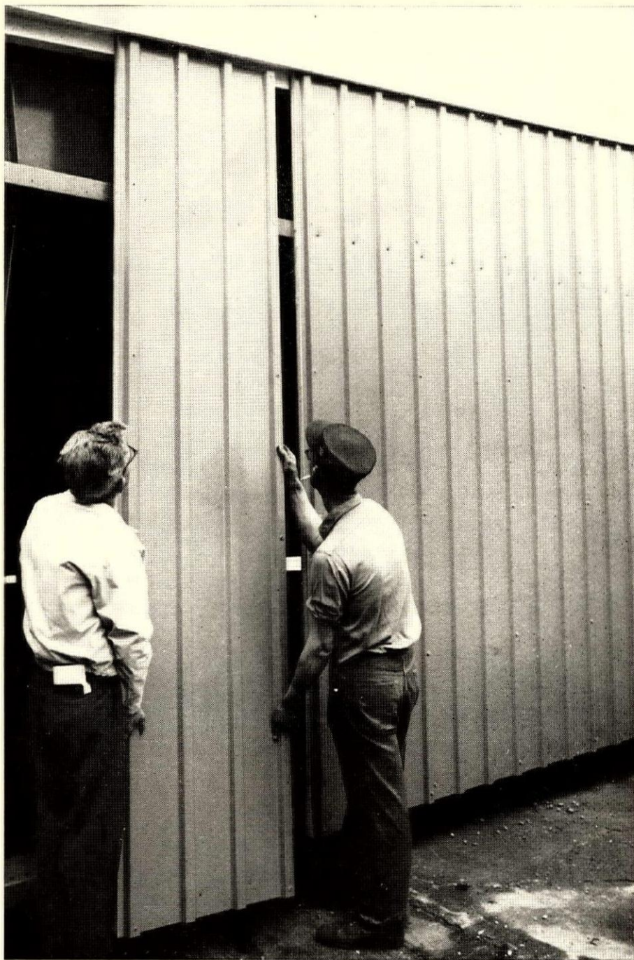
URETHANE FOAM CORE of panel is bonded to enameled steel skins on both sides.
