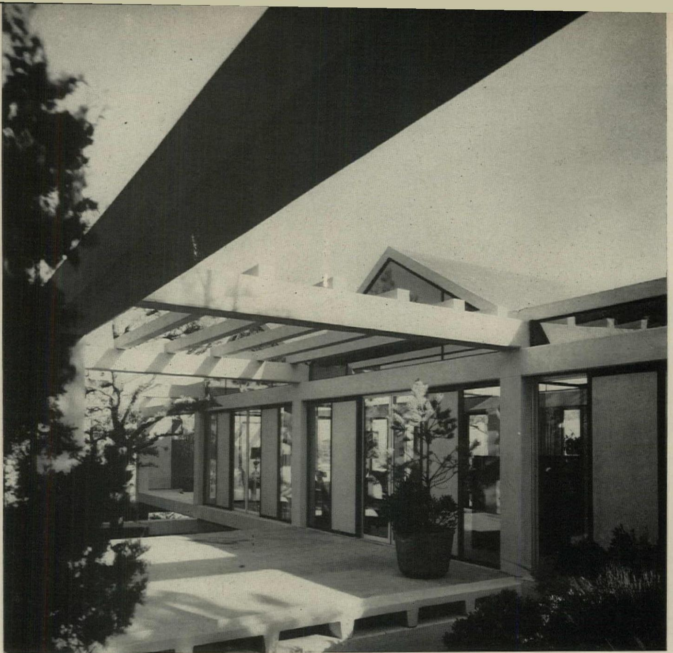
SIDE TERRACE adjoins living room, behind sliding glass doors at right. Posts, beams, floor sections and roof are all precast concrete.
