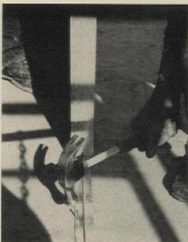
D PARTITION PANEL is held in place at bottom by T-shaped galvanized section which is nailed to floor, fits groove in panel.
