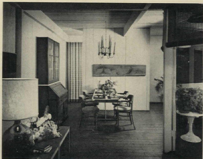
DINING AREA is an extension of the living room, foreground. Short island wall beyond table separates kitchen from the dining area. Door at right leads to center court. Walls, like ceiling and floor, are 2x6 t&g boards.
