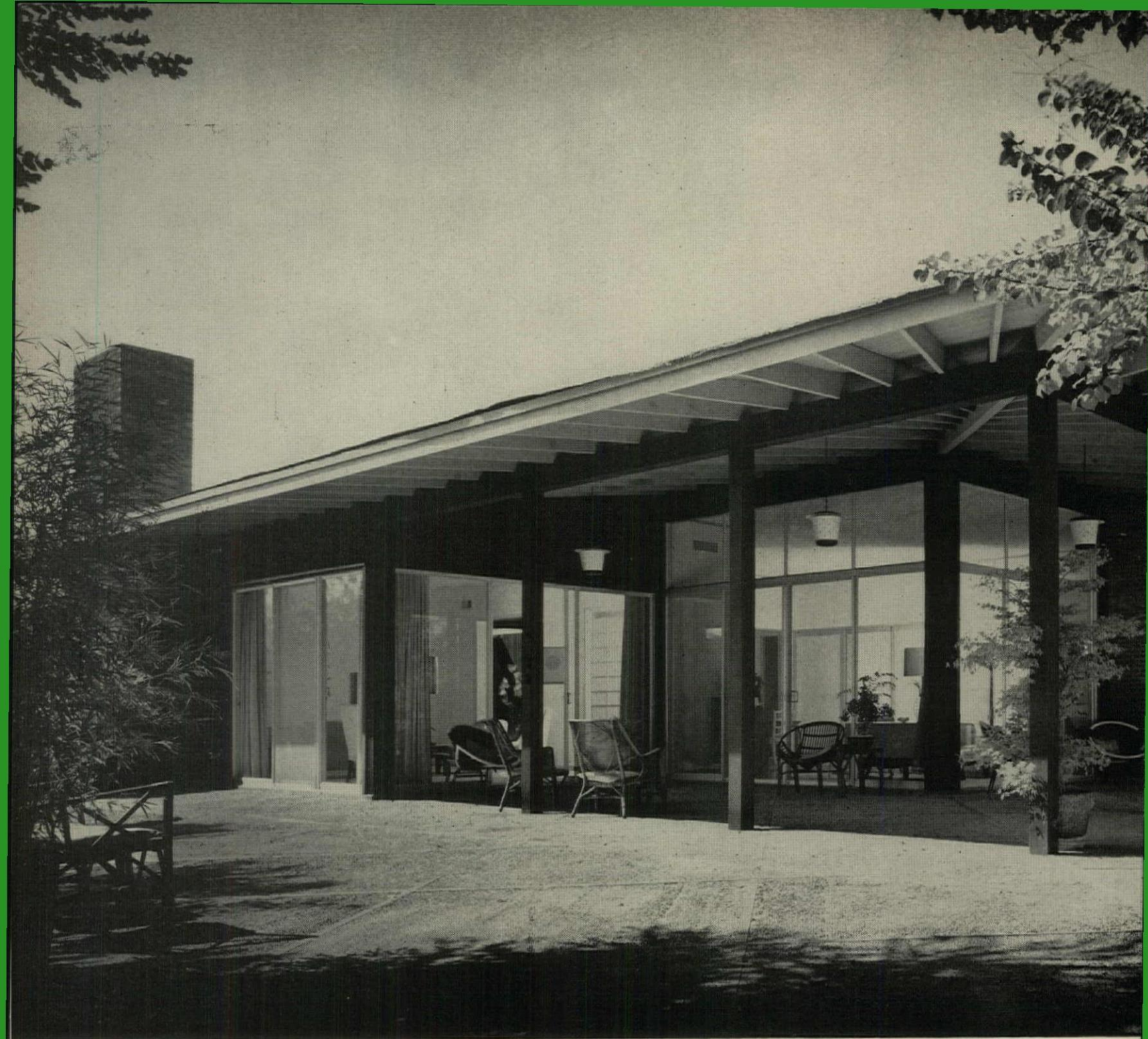
REAR TERRACE is protected by overhanging roof which is 16' deep and 11' high at inner wall. Living room is at left, family room in center.
