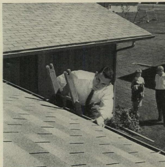
Prospect gets up on the roof to examine the high-quality, long-life Ruberoid Asphalt Shingles used by Seiffert.
