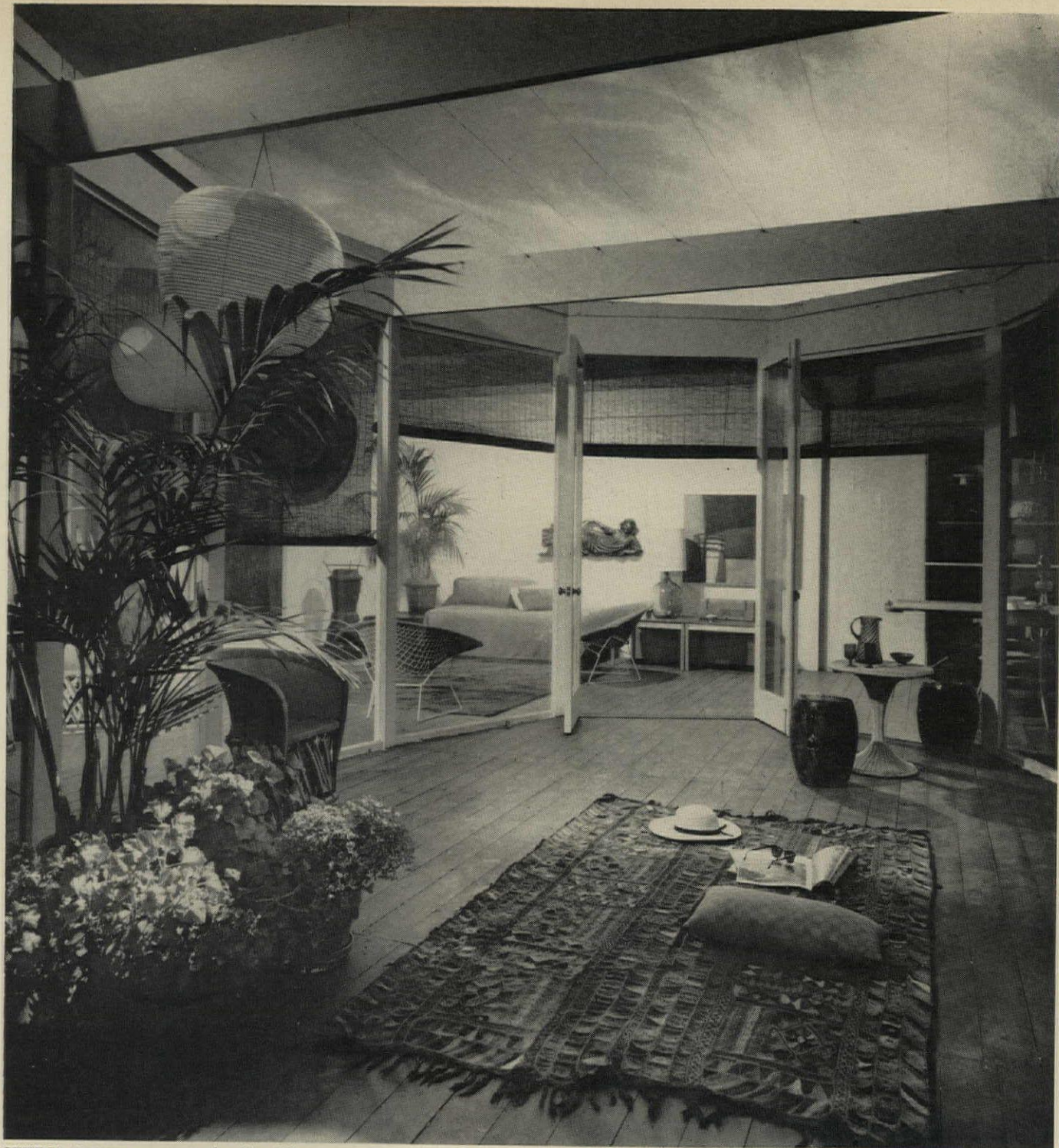
CENTER COURT opens to the sky. Wires strung between roof beams are supports for sunshade. Deck is same as interior floor, has weep holes so rain will drain out.
