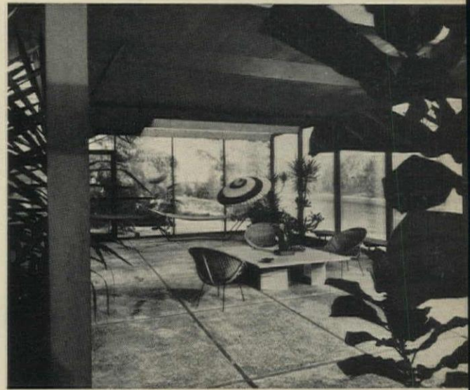
PORCH INTERIOR has floor of exposed aggregate concrete marked off with cypress screed strips. Ceiling is same as inside house. Roof beams are double 2x8's spaced 6'-1 3/4" oc. They rest on double 2x4 posts across front of porch.
