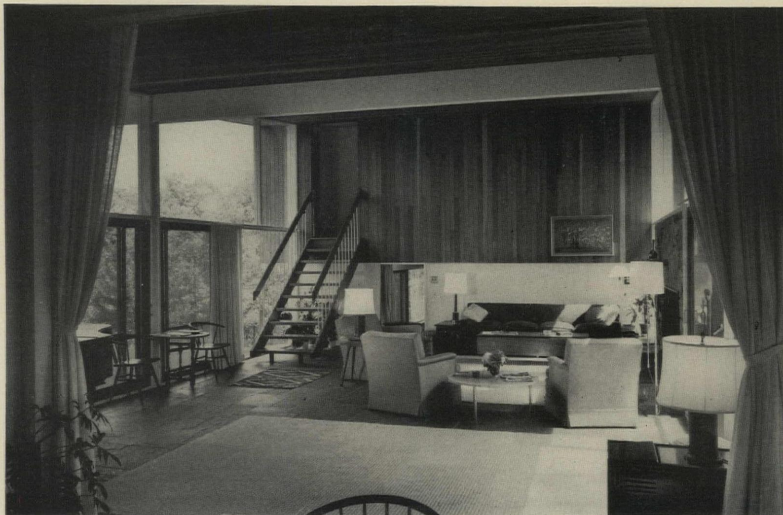
A backdrop of wood paneling highlights this airy living room and blends smoothly with a similar ceiling. Note the unusual, free-standing staircase of wood, and the posts that double as window frames.
