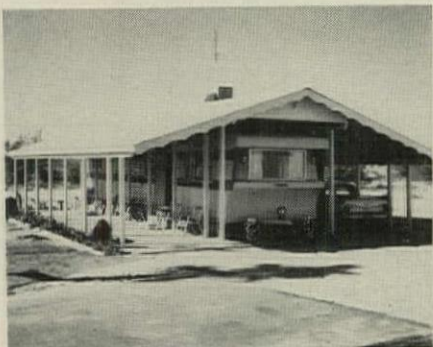
BIG ROOF that covers trailer and the standard paved patio is a popular addition.
