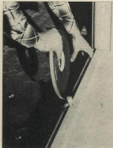
E EXTERIOR PANEL has bottom surface grooved to receive 1 1/2" x 3/4" bottom plate. Rubber seal strip is laid on slab outside plate.
