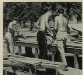
Calwire tools are ideal for building trusses and preconstruction of various kinds.
