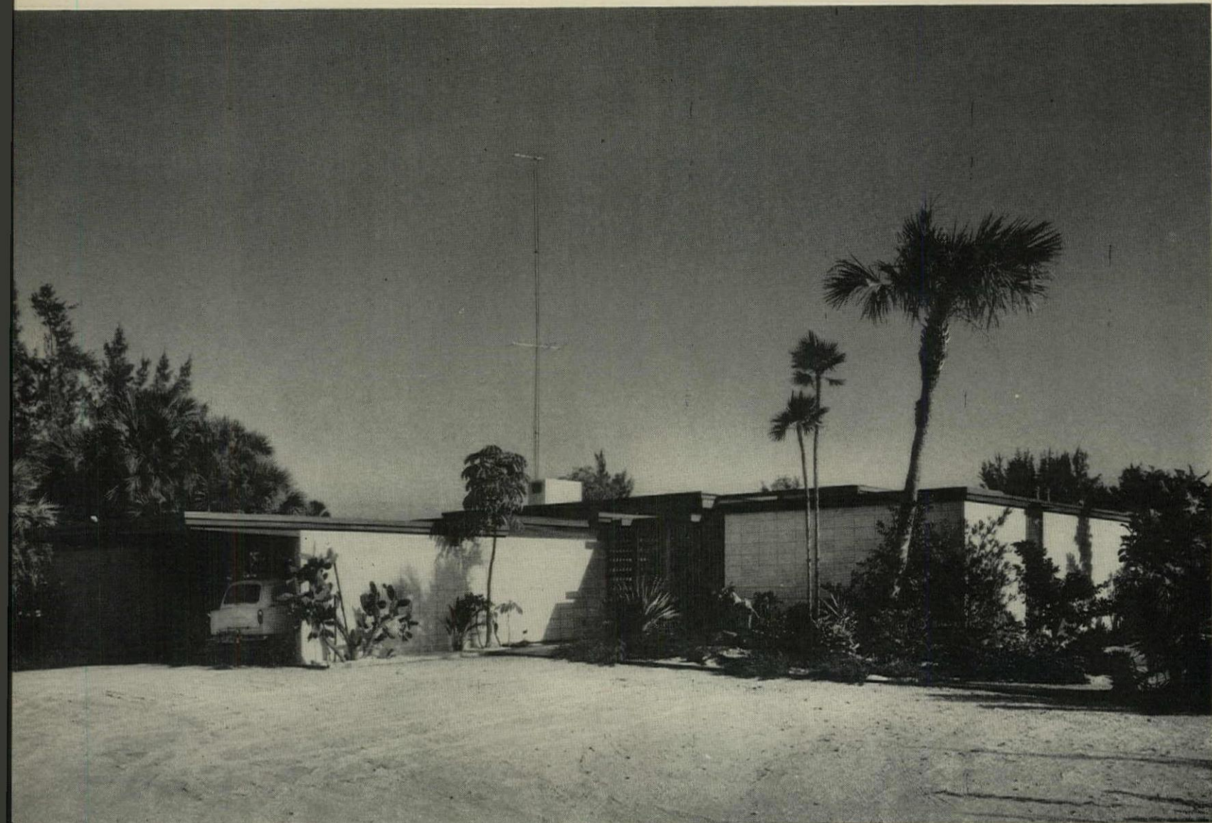
STREET SIDE of house has solid walls with no windows. Limestone "Ocala block" is natural cream color, requires only waterproofing.
