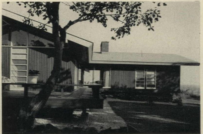
EXTERIOR WALLS are dark-stained redwood, sectioned into "panels" by painted window frames. Deck is redwood supported on piers, gravel under it is granite.
