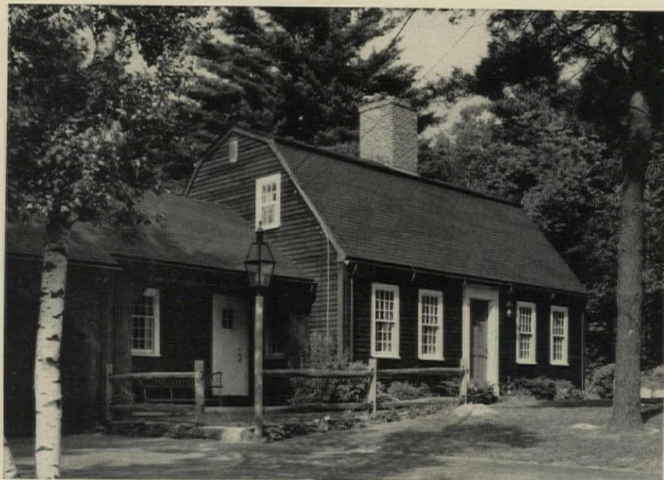
GAMBREL-ROOF COTTAGE , designed to get more head room in the garret of early houses, had pleasing lines that Wills often used in new houses like this one. Other authentic touches: stained siding, white windows.
