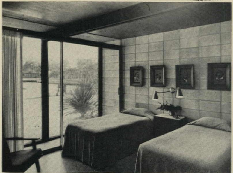
MASTER BEDROOM overlooks canal behind house. Simple construction includes unpainted block laid up in stack bond, exposed roof beams, mahogany plywood ceiling. Thin strips of glass fill space between ceiling and header over glass doors.
