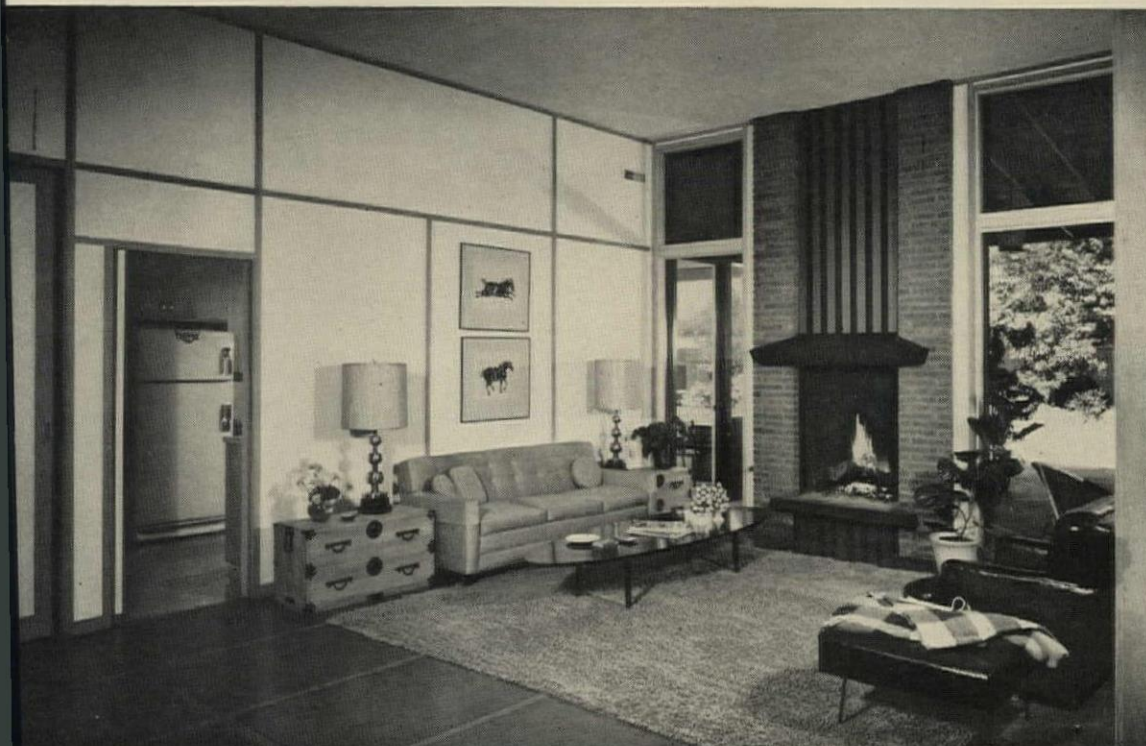
FAMILY ROOM gains informality from imaginative use of materials. Natural wood strips cover joints in wallboard, give wall a panelized look. Floor is colored concrete sectioned off with wood screeds. Fireplace breast is metal with accordion folds.
