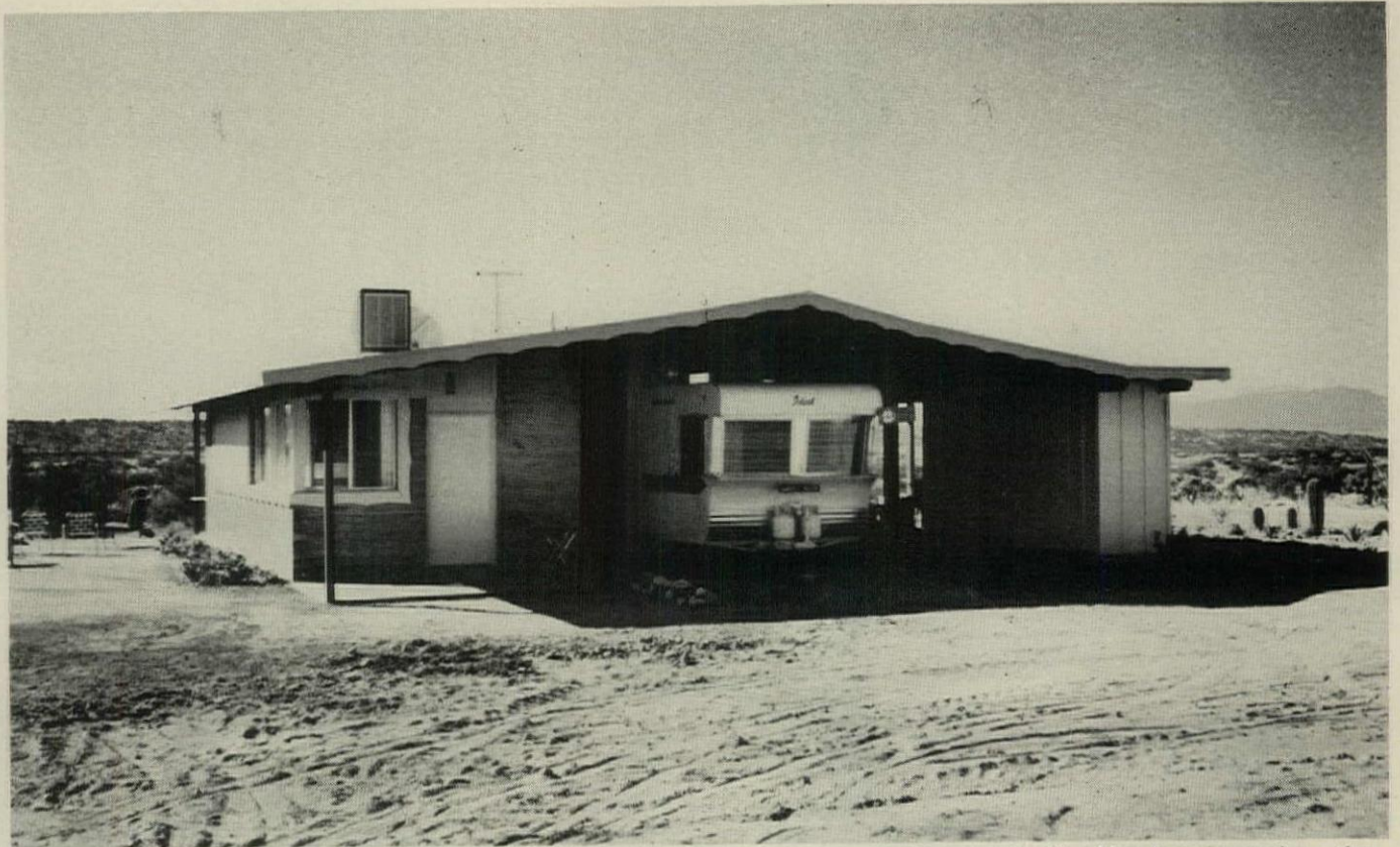
PERMANENT STRUCTURES, with family room, bedroom, and outside storage room, are added by many families. Most have evaporative coolers.
