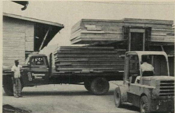
FORK LIFT is used to unload palletized materials from freight car and to load wall panels on delivery truck.
