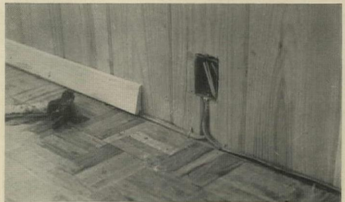
15. Baseboard chase for surface wiring
