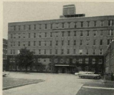
This hospital wing in Rochester, N. Y., was constructed in 1940.
