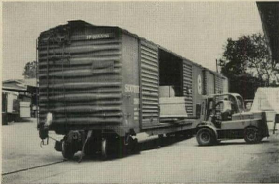
FORK LIFT is used to unload palletized materials from freight car and to load wall panels on delivery truck.
