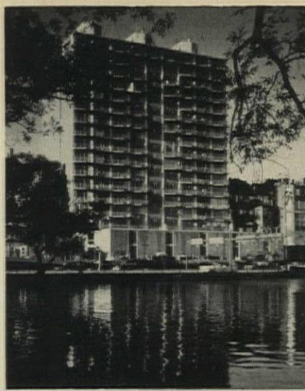
330 BEACON APARTMENTS Boston, Mass.
