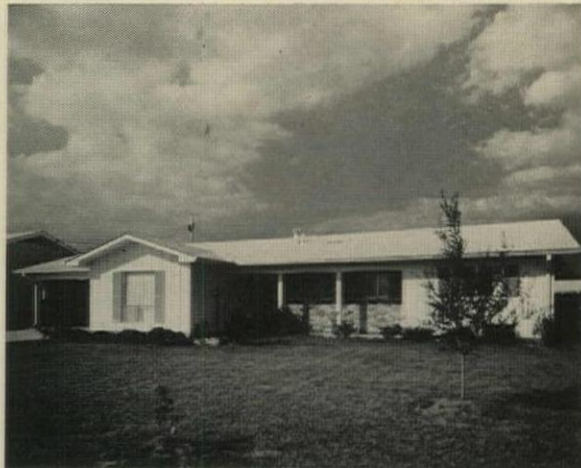
$24,000 BUILT-FOR-SALE MODEL had four bedrooms and two interior baths lighted by luminous ceilings.
