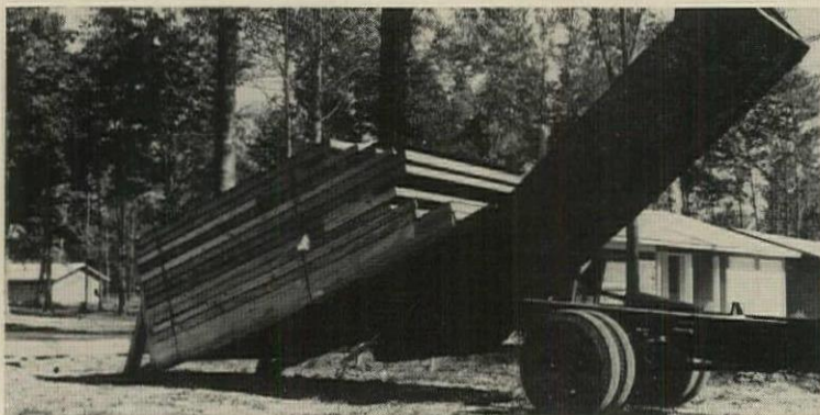
UNLOADING SKID keeps wall panels from breaking when dumped at site.
