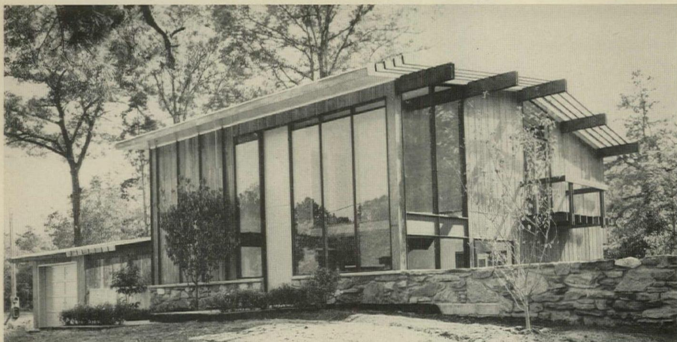
FRONT ELEVATION is lengthened by 4' rafter extensions, stone wall screening sunken garden, and garage and trellised play-area roof, left.
