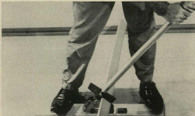
2. SPECIAL SHEAR cuts 10'-long base and cover sections to length. Coupling plates are used to connect and ground straight runs.
