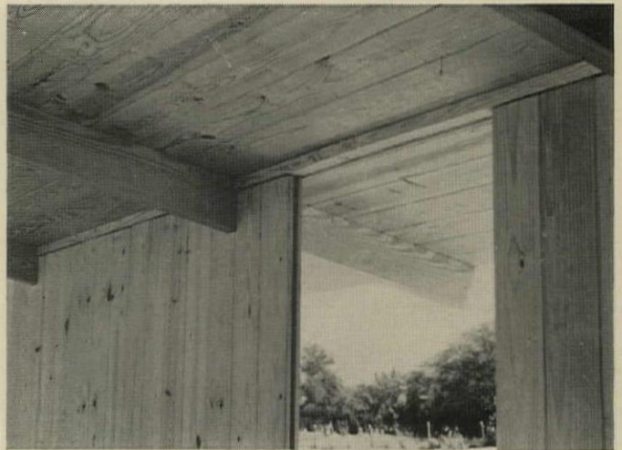
14. Tongue-&-groove decking for walls and roof
