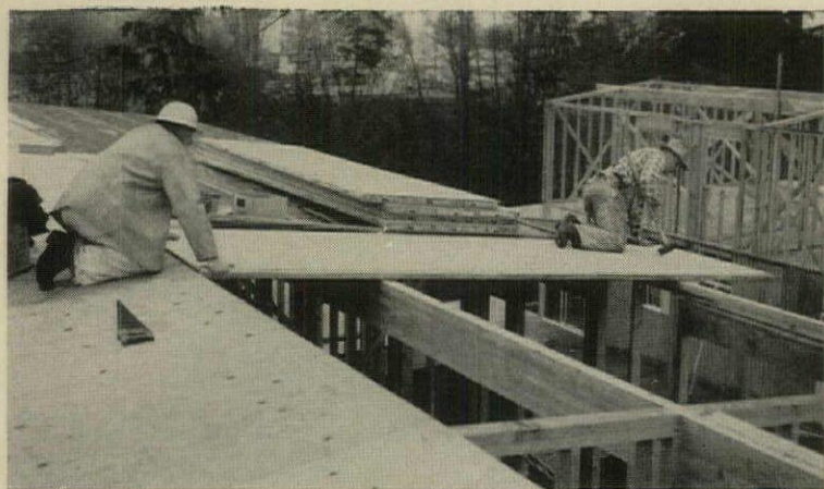
ROOF PANELS are long (16') but light, so two men can handle them. Stressed skin design and short span (8') need only 2x2 framing members.
