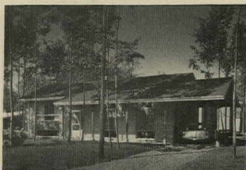
RAISED FLOOR of $10,900 ranch house designed for Cadillac Contracting, Toronto, by Lipson & Dashkin and Norman R. Stone is three steps above grade, allows good natural light in basement.
