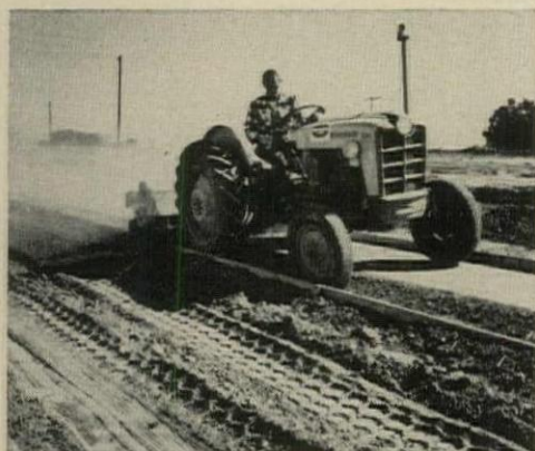
1. NEW GRADER scrapes grade to final contour.
