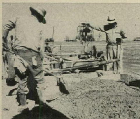
3. FORMING MACHINE shapes curb and walk.
