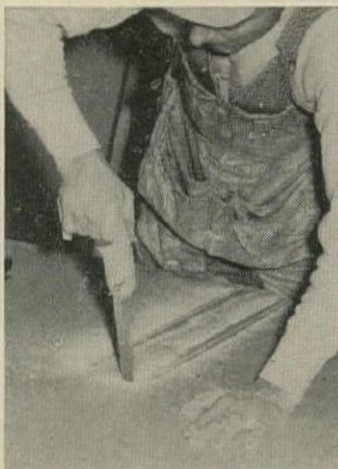
SAW CUTS for wiring chases or other openings are easily made.
