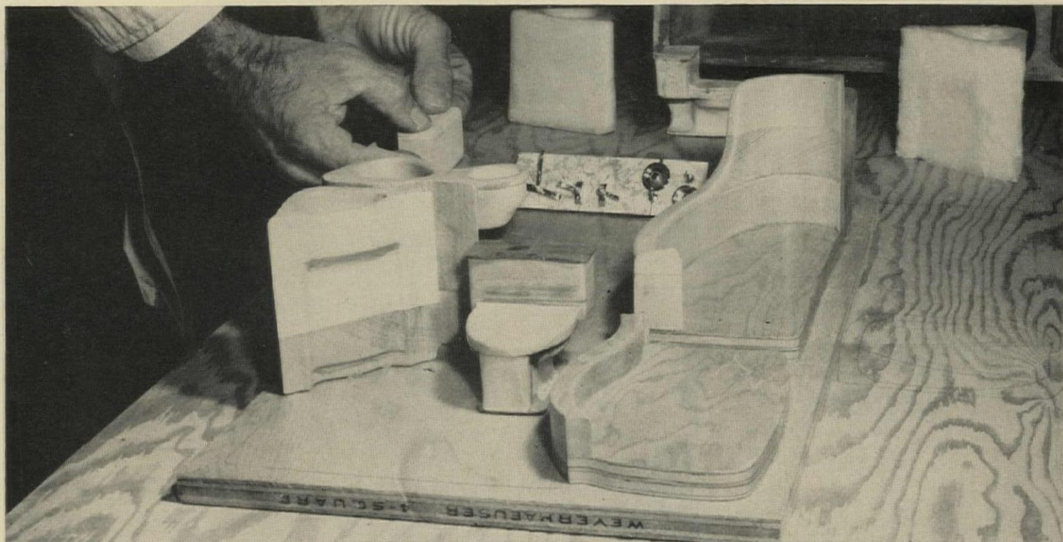
3 MOLDS FOR ONE-PIECE BATHROOM will be used to build small-scale fiberglass-and-plastic mock-up.
