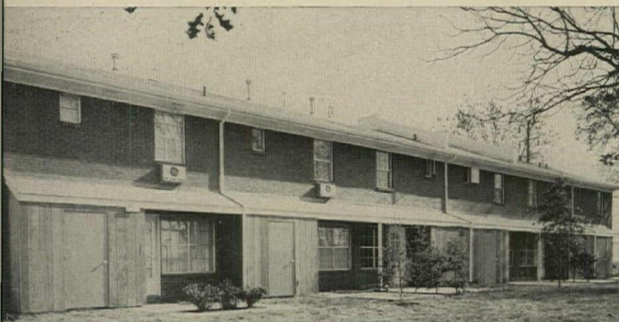
MAINTENANCE-SAVING MATERIALS , shown here at rear of houses, include redwood (for storage sheds), brick (for wall veneer), aluminum (for windows and gutters).
