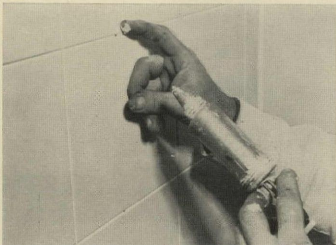
NAIL IS HIDDEN with white grout to preserve full tiled appearance.
