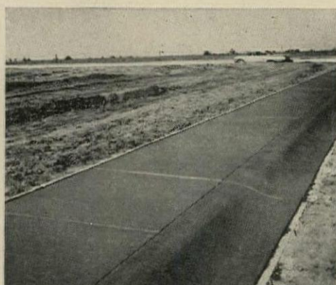
6. CURB AND WALK go down at 16' per min.
