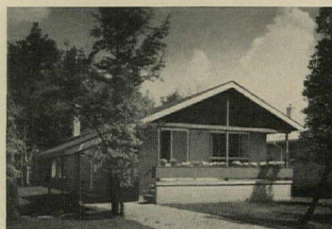
FRONT PORCH shields living room in this $10,900 Cadillac Contracting house, which has plan almost identical with Cadillac house at left. This one also has main floor three steps above grade level.
