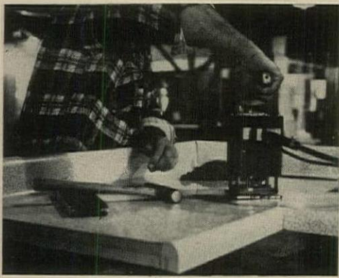
OLD WAY: Plastic laminate countertops were mitered at corners to get a neat joint.
