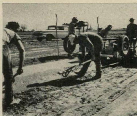
4. FLOAT MEN put final finish on curbs.
