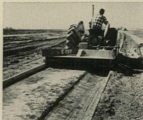
2. WOOD RAILS keep blades at correct depth.
