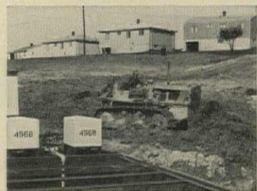
... backfilled and readied for dependable, efficient sewage treatment at the site.
