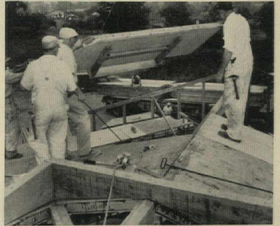
PEAK PANELS are supported by cribwork, the only bracing needed during construction. Girders carry no load, act merely as panel ties.
