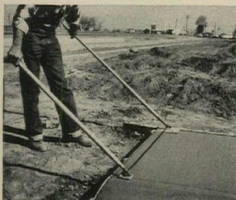
5. FINISHER trowels walks and scores surface.
