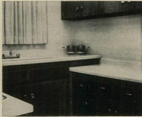
NEW WAY: Side countertops are dropped 4", simply butt against cabinets in sink counter.
