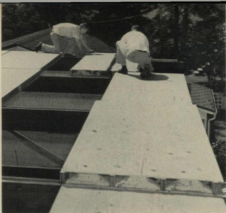
ROOF PANELS are 4'x8', have 2x3 framing members. End blocks are notched for venting. Drawing shows eave detail.
