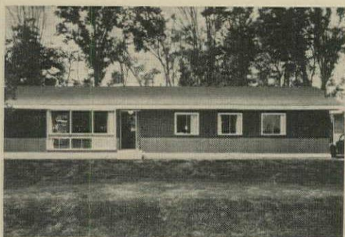
WIDE LOOK of $15,000, 1,350 sq ft Woodview Development house is achieved by keeping roof line low and by aligning bottom of bedroom windows with bottom of fixed sash in living room.
