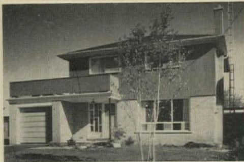
TWO-STORY HOUSE designed for G. S. Shipp & Son in Toronto by Lipson & Dashkin has four bedrooms on top floor, 1½ baths, big entry hall, and family room in basement. Price: $16,000.
