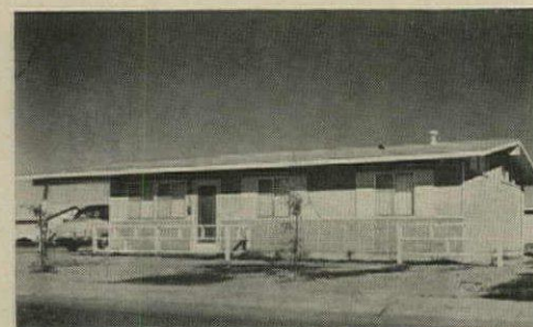
RESEARCH HOUSE , third of five, used polystyrene foam-core panels for roof, walls, and partitions.
