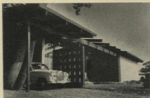
L-PLAN HOUSE built by Teron Construction in Ottawa has wide overhang shielding glass wall of living room. Carport extending to front in foreground is built around large tree. Price: $14,000.
