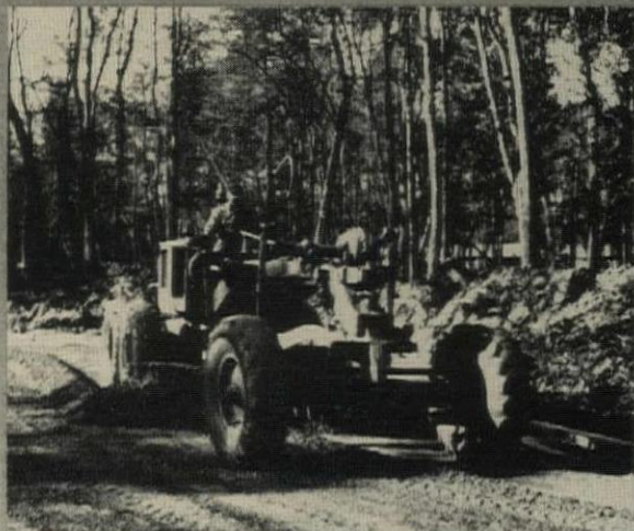
Road grader is charged to job at $1.75 per hour
