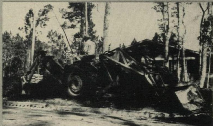
Back hoe with attachments is charged to job at 50¢ per hour
