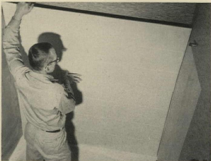
SECOND PANEL is 3x7 tiles, finishes wall to 5' height above tub.
