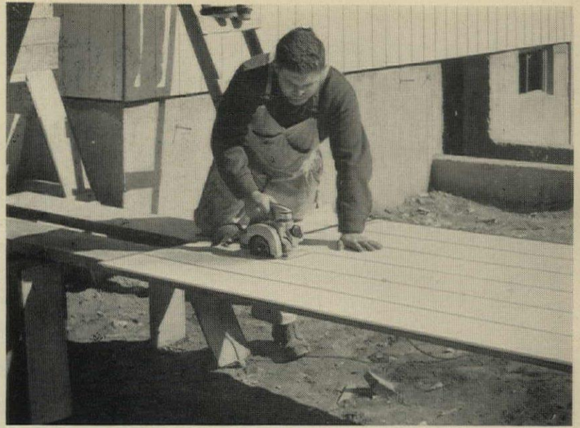
EASY TO SAW AND NAIL. Medema Builders say Insulite Primed Siding "cuts easily with hand or power tools—won't crack, split or splinter." And because its density is close to that of natural wood, no special nails are needed.
