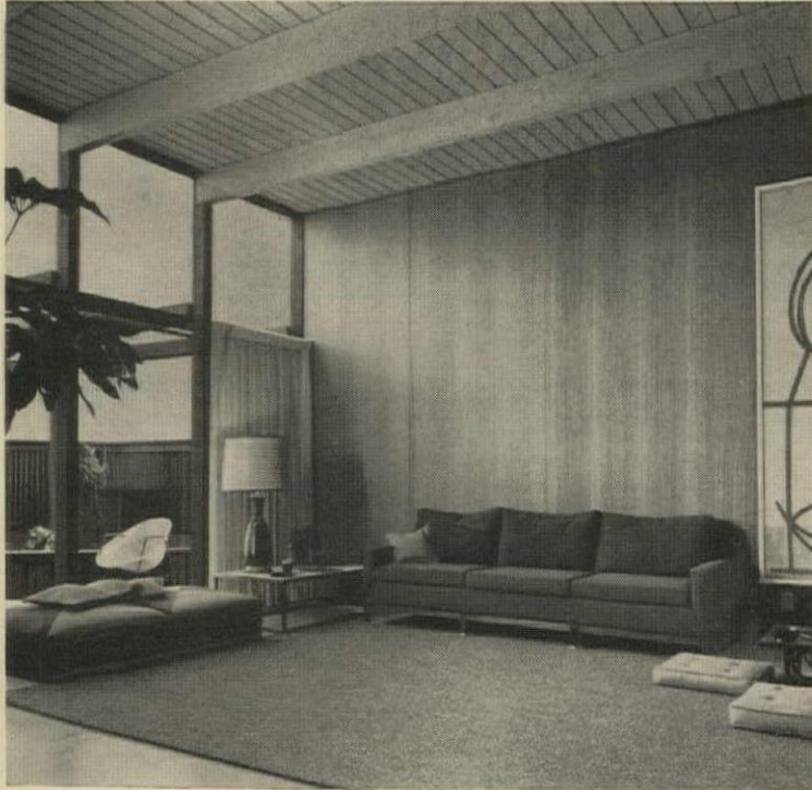
Wood's indoor-outdoor beauty makes a strong selling point in modern living rooms. Here, modified plank and beam construction makes beams double as window frames. Wall paneling is hardwood plywood.
