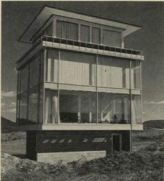
GLASS ENVELOPE encloses first two floors of 26'x26' three-story test house. To provide comparative test data, envelope was not extended to top floor. Walls face four compass points.
