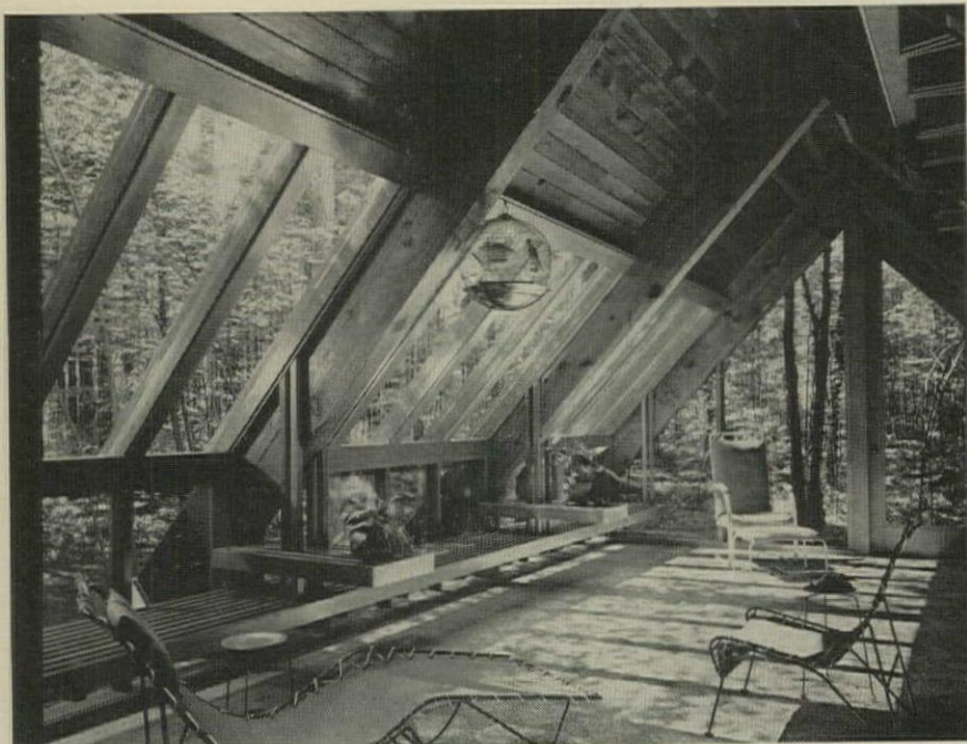
PORCH has fixed glass lights set into roof slope. Lower windows open to provide ventilation.
