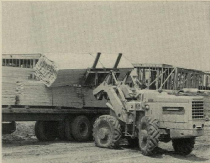
FAST UNLOADING means quick turnaround. Modern lifts can load or unload a truck in 20 to 30 minutes, move up to 1,500 bd ft at a pass.
