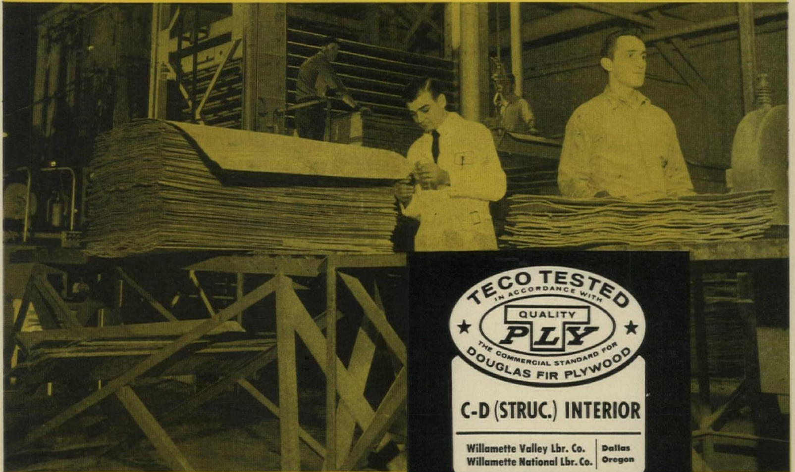
Teco Technician inspecting plies during regular production.
