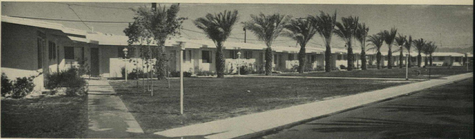
CO-OP APARTMENTS have one or two bedrooms, sell for cash at $8,500 to $12,100. Maintenance charges are $30 to $40 a month.
