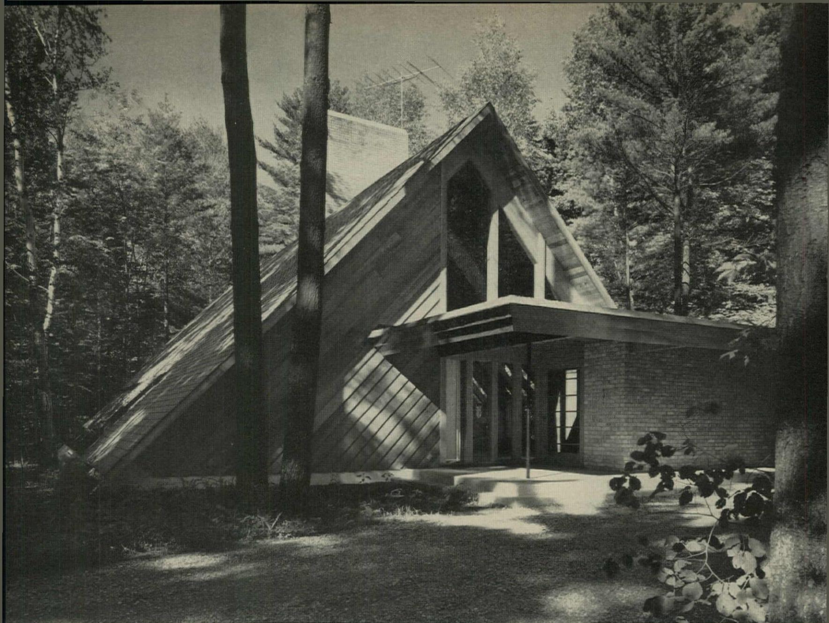
A-FRAME HOUSE in Midland shows Dow's affinity for structural inventiveness and simplicity. Bold diagonal sheathing contrasts with small scale of brick.
