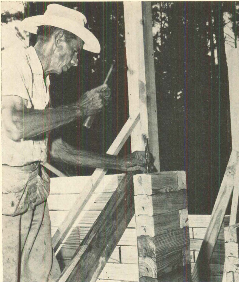
WALL IS LAID UP with milled t&g wood blocks. Techniques: the same as in masonry with glue and 8 d nails replacing mortar.
