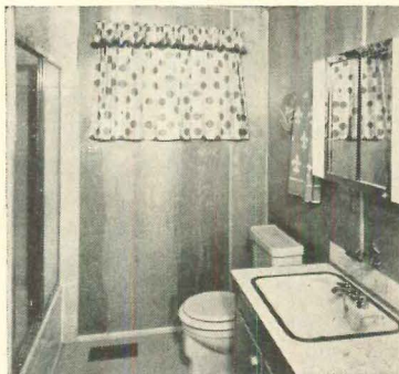
BATHROOM in Midwest house was pre-finished and fully equipped in plant.
