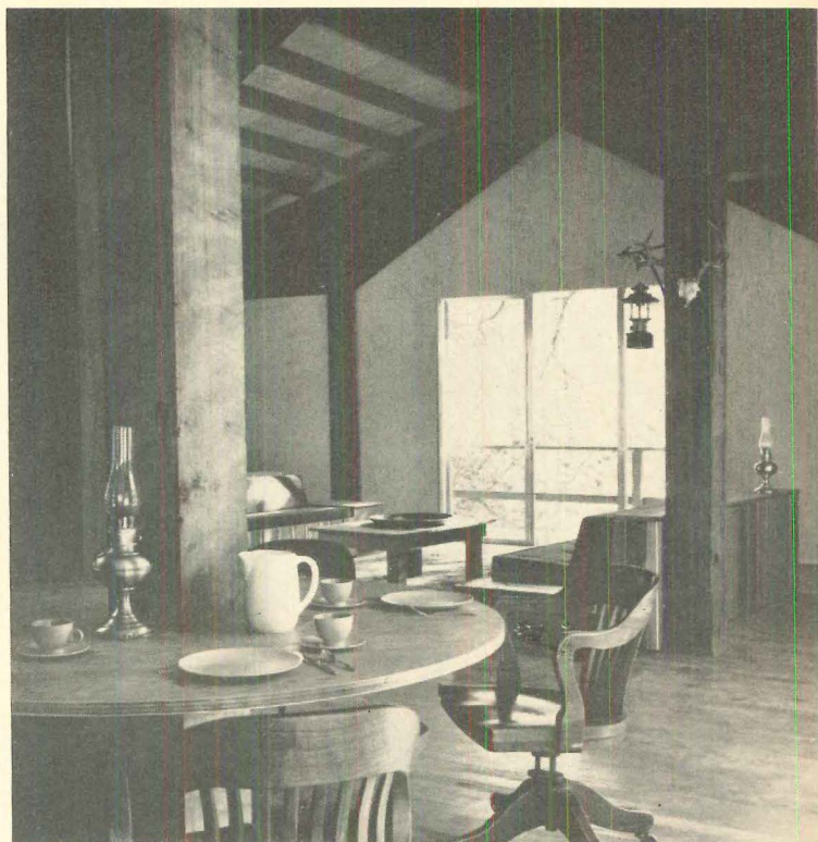
DINING AREA has round table hung from a structural post. The strong structure is emphasized as a design element; posts, box beams, and purlins are stained to contrast with the unfinished plywood walls and the roof decking.
