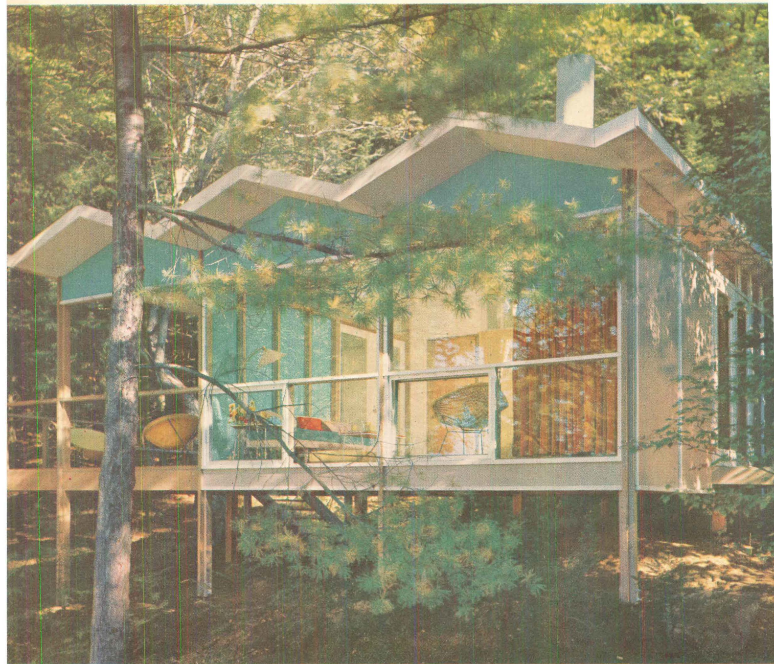
DOWNHILL SIDE OF HOUSE looks out to view through a glass wall or from partly roofed deck. House juts from slope on post foundation.
