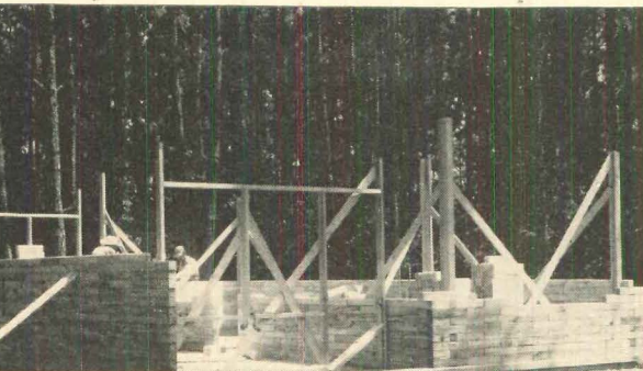
BUCKS are placed when walls reach sill height. Upper ends are trimmed to leave 1/8" between buck and ends of block.
