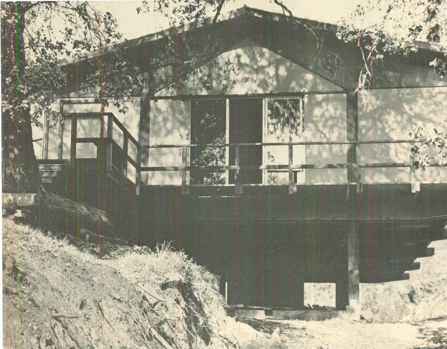
HILLSIDE HOUSE rests on posts that support cantilevered floor and roof systems. At roof line, triangular box beams supporting roof acts as decoration.
