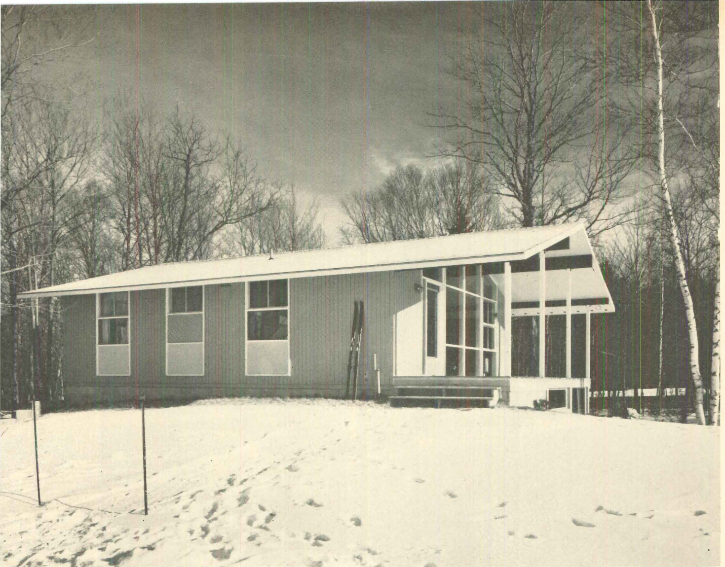
ROOFED HOUSE has simple lines, trim detailing. The roofed-over deck extends the summer-time living space, shades the glass wall from rain and glare.
