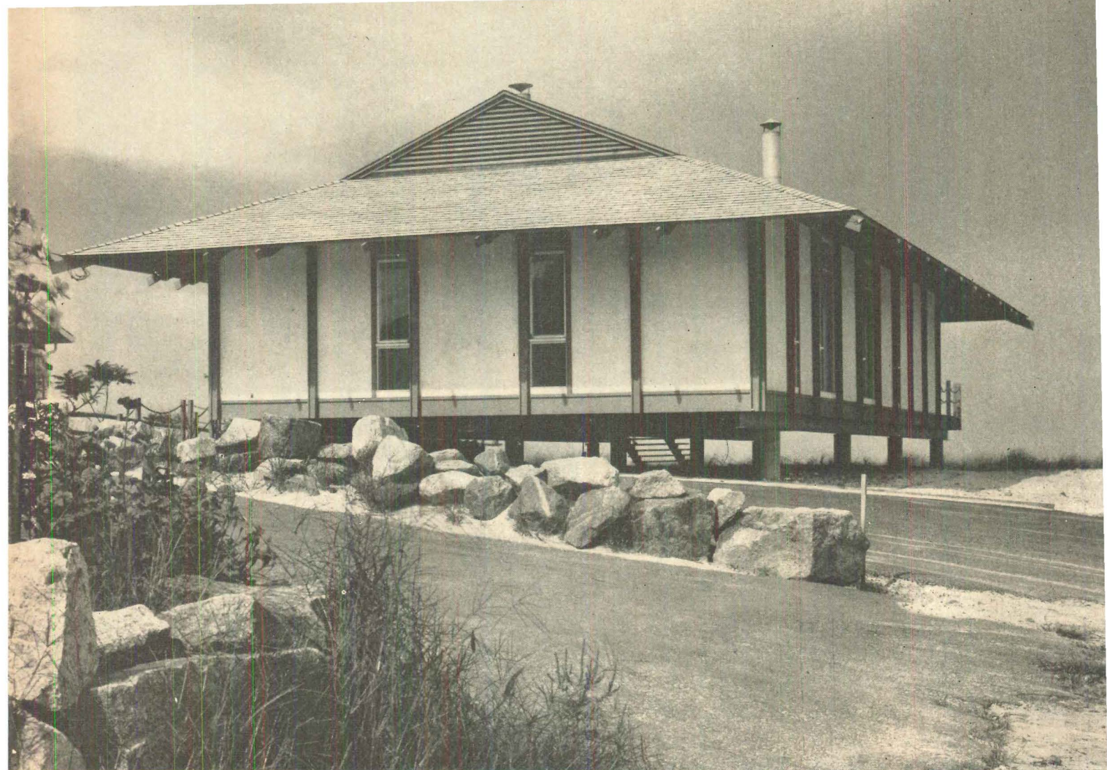
BEACH HOUSE sits on pier foundation which protects it from dampness and storm tides. Overhangs shelter house and deck at rear from glare and
