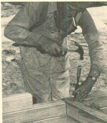
TONGUE IS CHISELED off partition block to get level fit for the next course of block where it ties into outside wall.
