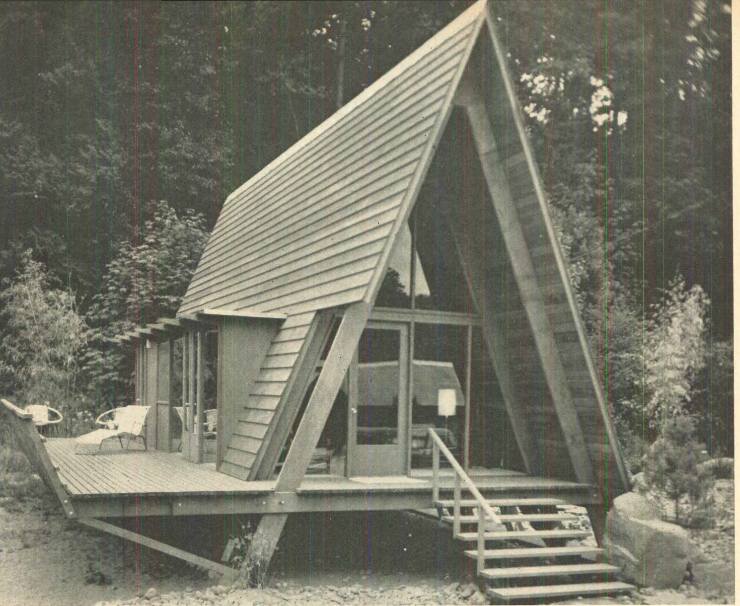
ACME HOUSE has 18'-tall glass end wall. Living area opens through glazed doors, left, to cantilevered deck. Roof is redwood clapboards.
