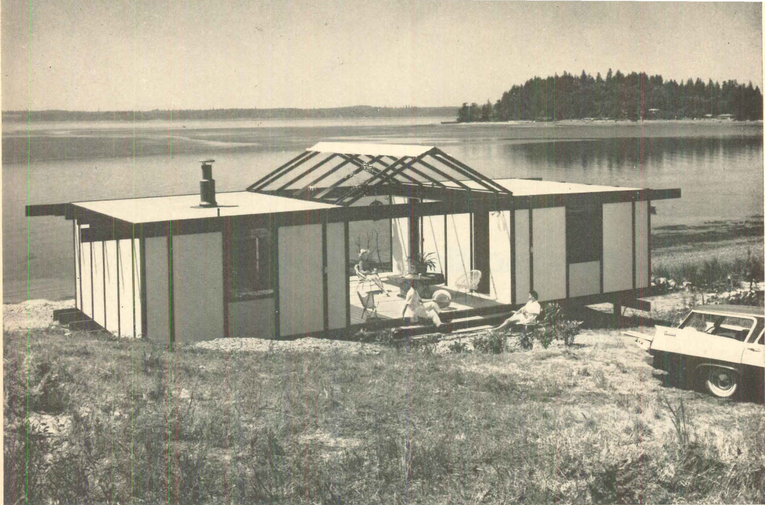
LAKESIDE CABIN encloses 640 sq ft in two units. Open deck between has "convertible" canvas roof as shelter against sun or rain.
