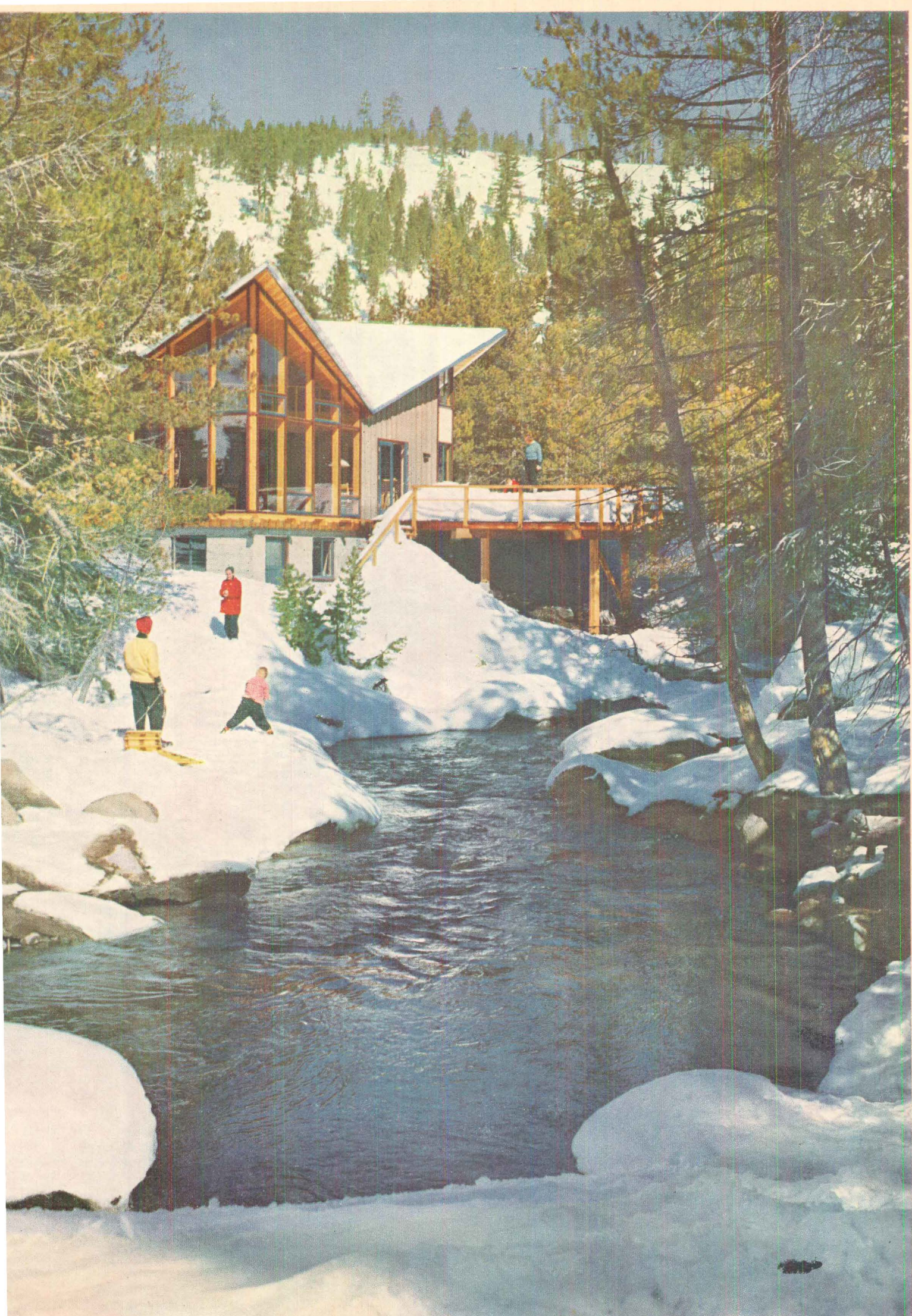
GLASS GABLE overlooking mountain stream lets light into living room and balcony above it. Conventionally framed walls have cedar board & batten siding
