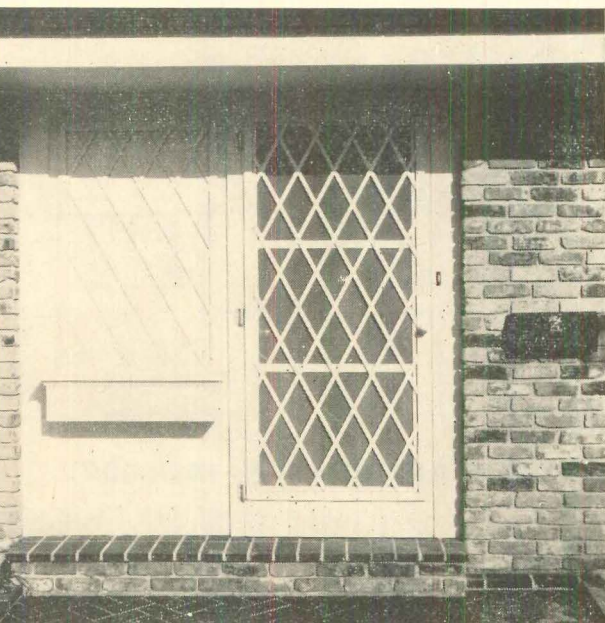
ANOTHER VERSION of the Delmar is typified by this front door treatment. A diamond grille is added to the door, and diamond patterns to panel at left. A planter is also attached to panel.
