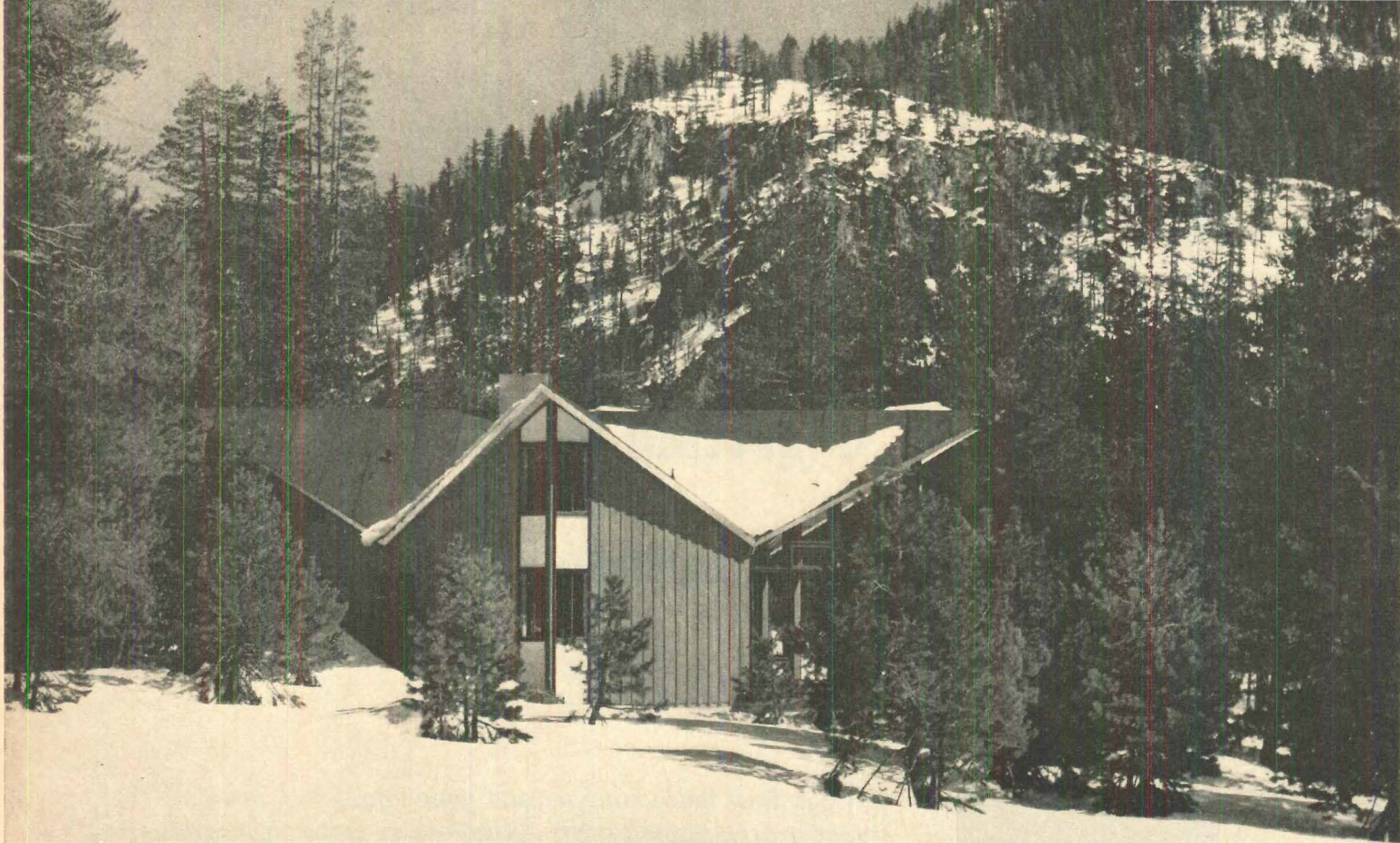
MULTI-GABLED ROOF of Squaw Valley, Calif. house is steeply pitched to shed snow. Laminated 2x4 decking is topped by 1" insulation and built-up roofing.
