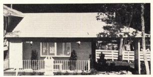
FINISHED ROOF of Jacksonville model has heavy shadow line produced by use of aluminum Bermuda strip shingles.
