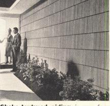
Shake-textured siding is new from National Gypsum. Gold Bond Classic-Shake is asbestos cement with an acrylic coating in ten colors. Deep wood-like striations are complemented by heavy shadow line at the butt. Siding is immune to rot, weather, vermin, fire, and dimensional change.
