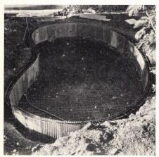
New pool system is designed to bypass specialty contractors, make installation a job for builder's crews. Sidewalls are formed of flexible corrugated steel that will take any shape, will flex with freeze and thaw cycles. Floor is made of reinforced concrete. Earth is backfilled against steel form, capped with a reinforced concrete ring. Average pool should go in place for less than \$2,000.
