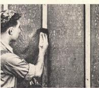
New plywood siding gives the look of resawn lumber in a 4'x8' sheet, for a materials-plus-labor saving of 15% to 25%. The new panels may be applied directly to the studs eliminating the need for sheathing within the specifications of FHA minimum property standards.
