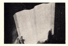
New look in plastic comes from the sharp-lined corrugations in Alsynite's Ridgeway fiberglass building panels. The new sheet is designed for porch, carport, and patio use, contains a filtering additive to control light and heat. Ridgeway is finished with Alsynite's new Superglaze, carries a written ten-year guarantee.
