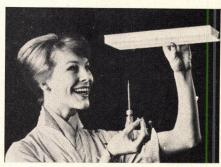
Slim fluorescent fixture is only 7/8" thick. Alkco's Little Inch undercabinet light delivers 40 foot candles at 15", can be mounted singly or in runs. Alkco's diffuser is acrylic, a tough plastic that will neither warp nor discolor.
