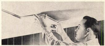
TILE IS PLACED against ceiling; pressure spreads cement evenly.
