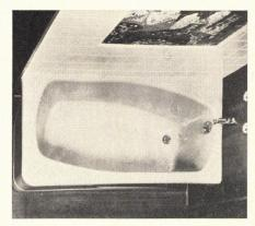
New corner tub has all the features of Contour model introduced last year: offset cavity; wide seats at two corners; narrow, easy-to-grasp front rim. Tub is 5' long, 32" wide, 16" high. Corner model adapts well to remodeling. In new construction, corner tub can make bathroom look roomier. Tubs come in white and six colors.
