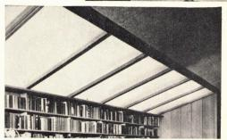
SKYLIGHTING. Aftic space is transformed into a smart, unusual studio, with lights of wired glass in the Luminex® pattern with Satinol® finish. This installation adds exterior interest to the house as well.
