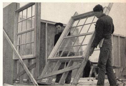
Fits all frame wall and panel construction! Here unit is set in standard stud wall construction. In multiple openings just butt Strutwalls against each other for large economical glass areas. Absence of separate casings provides clean, trim lines. Note narrow meeting rail gives more glass area.
