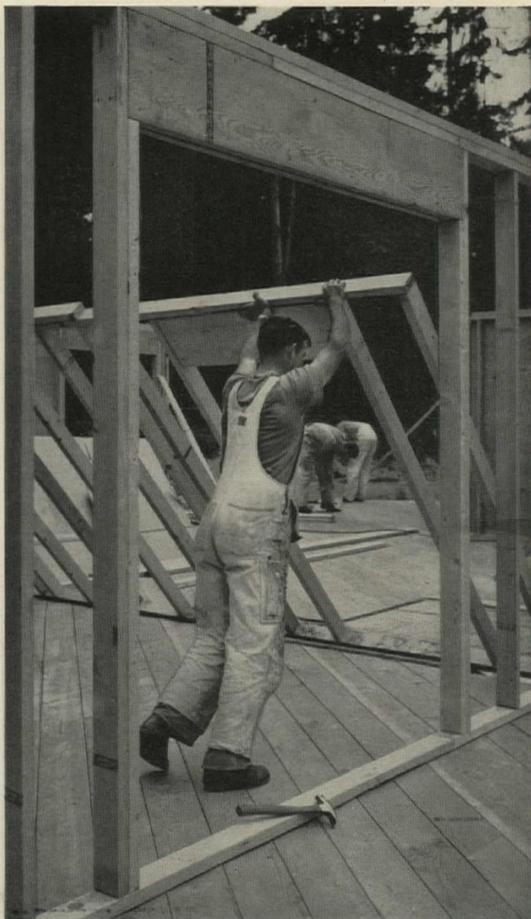
Cost-cutting teamwork is possible with wood framing. Inclement weather need be no deterrent to pre-assembly. Diagonal sub-flooring makes sturdy, resilient floor base with natural insulating qualities.
