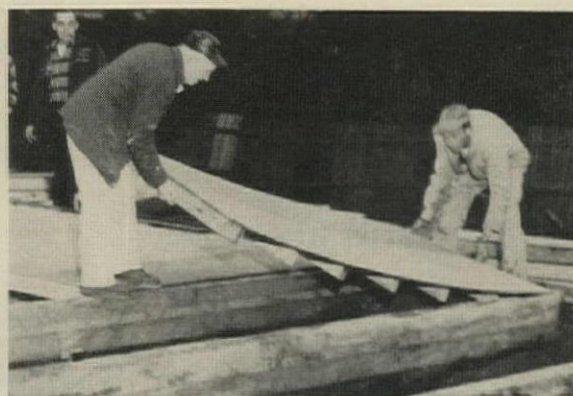
SUBFLOOR PANELS are dropped between beams.
