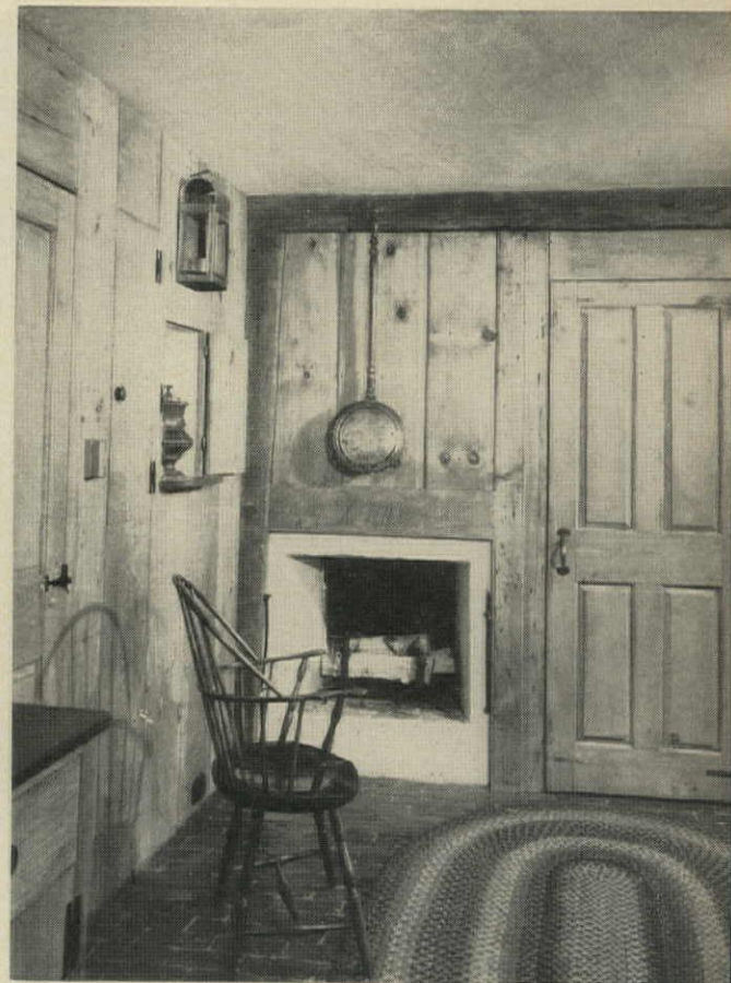
DINING ROOM FLOOR is old sidewalk brick; paneling is all pine. Small fireplace shares same chimney as living and family rooms.
