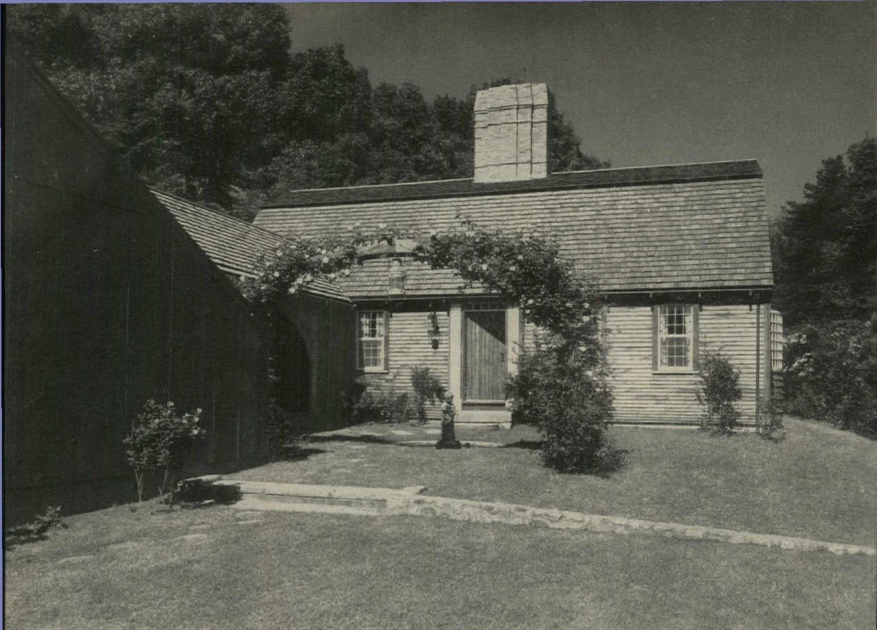
ENTRANCE to the house is past a rose arbor, once part of an old estate. Gambrel roof is of old hand-split shingles.
