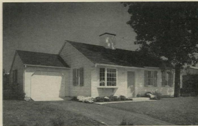
DEERWOOD MODEL for National Homes has small-paned windows, narrow clapboards, massive chimney of authentic New England style.
