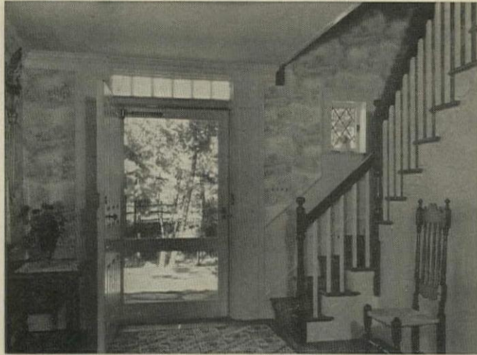
COLONIAL HOUSE HALL gets daylight from small panes set in over the entrance door. Note the scenic wallpaper and the detailing along the open-string stair. Small stair window has diamond-shaped panes.
