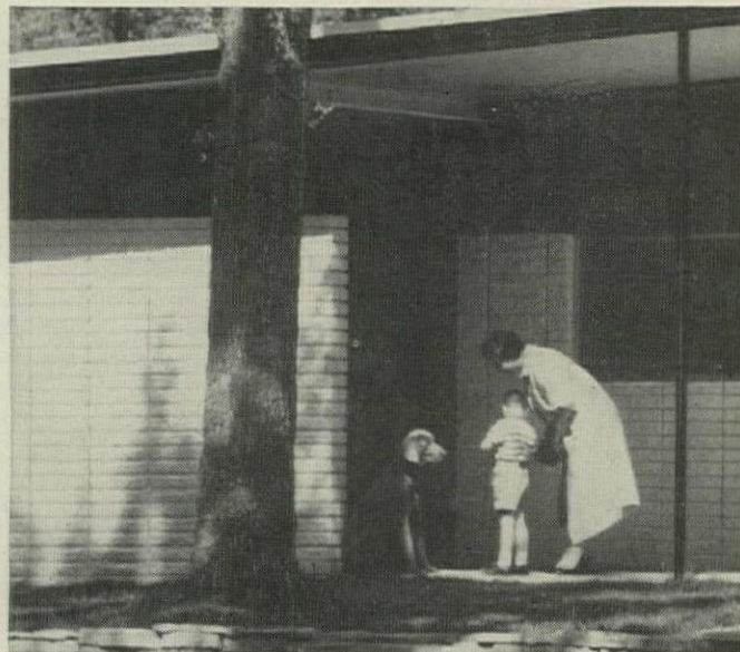
Design interest is achieved with coarse-textured block laid in a stacked bond
