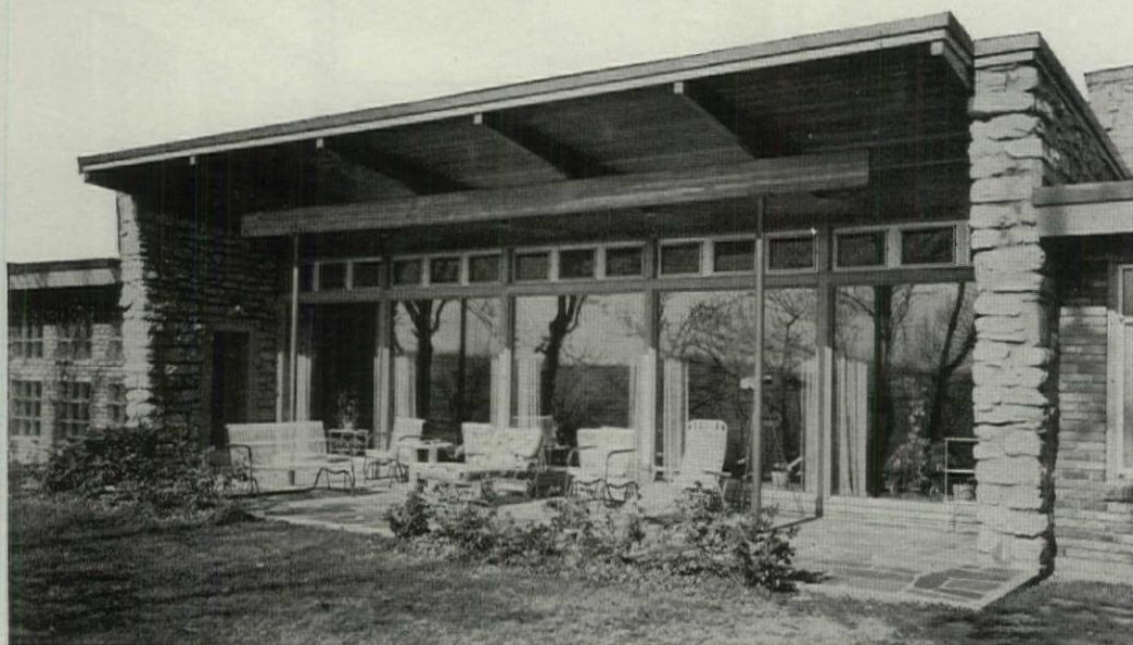
EUGENE IMBUS RESIDENCE, Cincinnati Architects: Garriott & Becker, Cincinnati. The five 3-7/16" x 11 3/8" x 32' beams are tapered for overhang and supported by a 3-7/16" x 11 3/8" x 28' 8 1/4" longitudinal beam.
