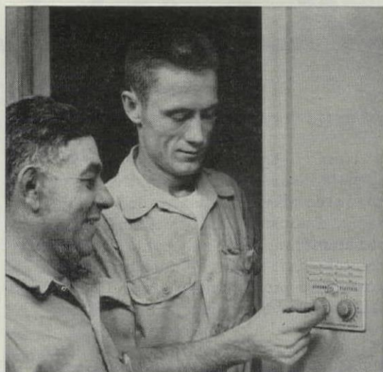
"One twist of the dial, and 12 lights come ON" says Pat Sirpilla (left)—as Ellis Bush, electrical contractor, demonstrates the G-E master selector switch.
