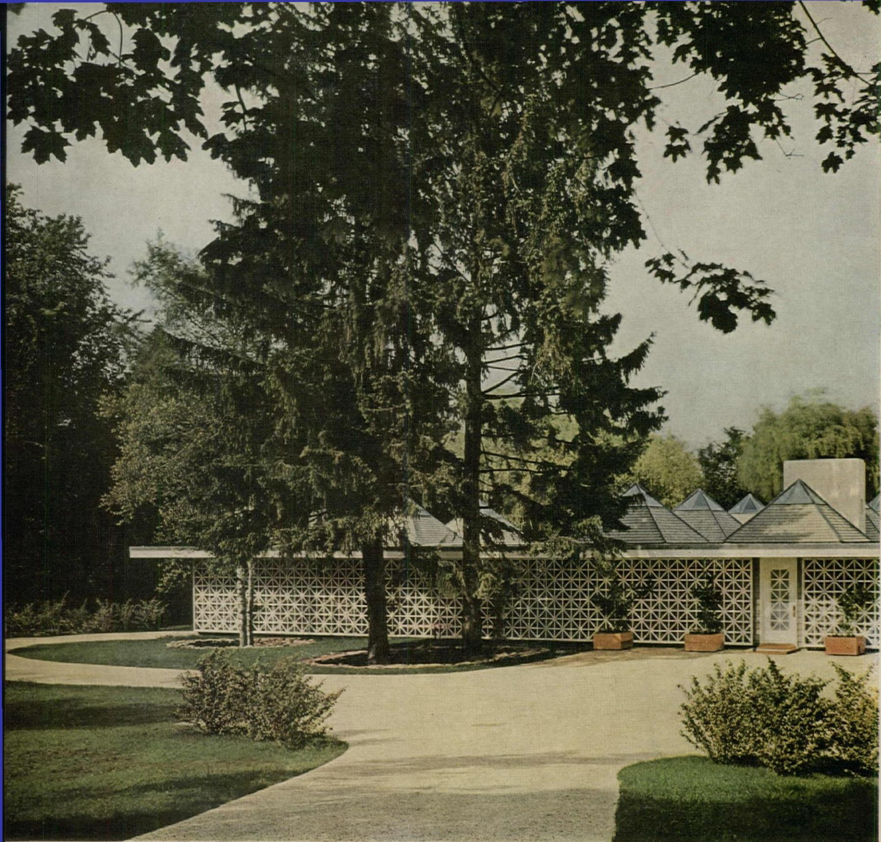
GLASS-TOPPED PYRAMIDS (12 in all) and latticed facade turn simple flat roof and shingle house into a highly decorative residence.
