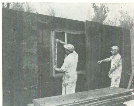
SECOND FORM locks plumbed frame in place.
