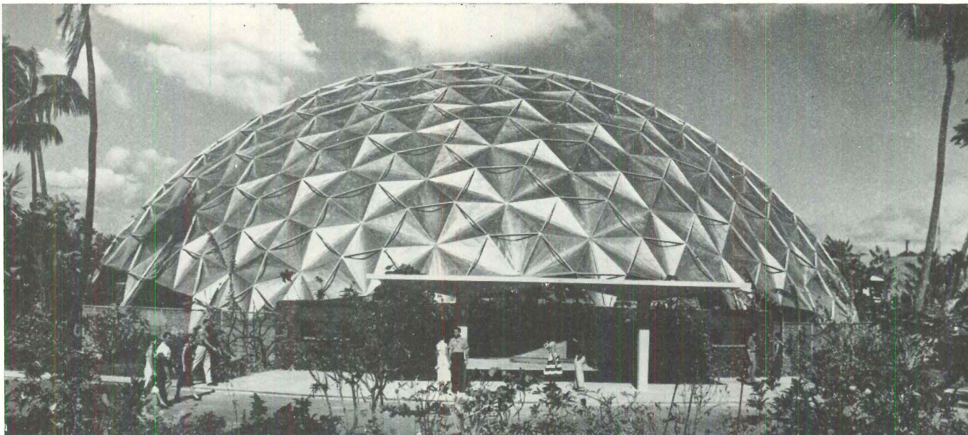
ALUMINUM-DOMED AUDITORIUM in Honolulu spans 145 ft without interior support. Structure is a geodesic dome.
