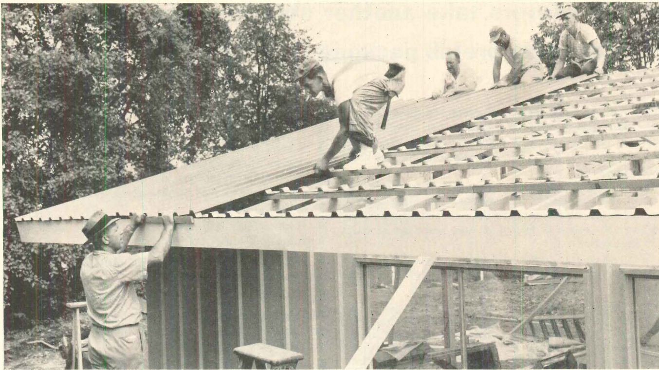
ALUMINUM-SKIN HOUSES have roof and wall panels that can be made only on heavy presses, may mark beginning of new trend.
