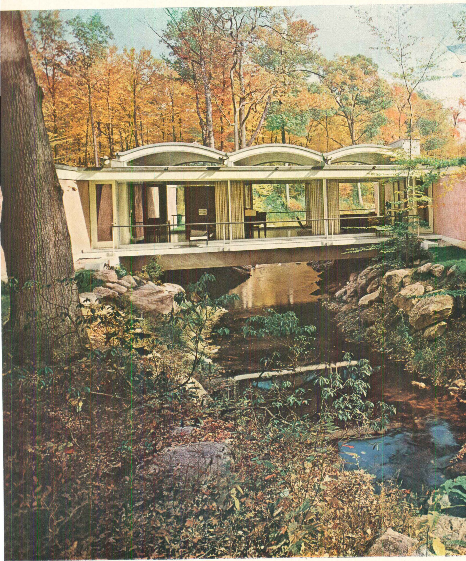
House bridges stream with 47' living-dining room. Glass walls emphasize bridge effect, also give a view of brook, both upstream and down. Balconies parallel both sides of bridge. Three vaults add a sense of motion.
