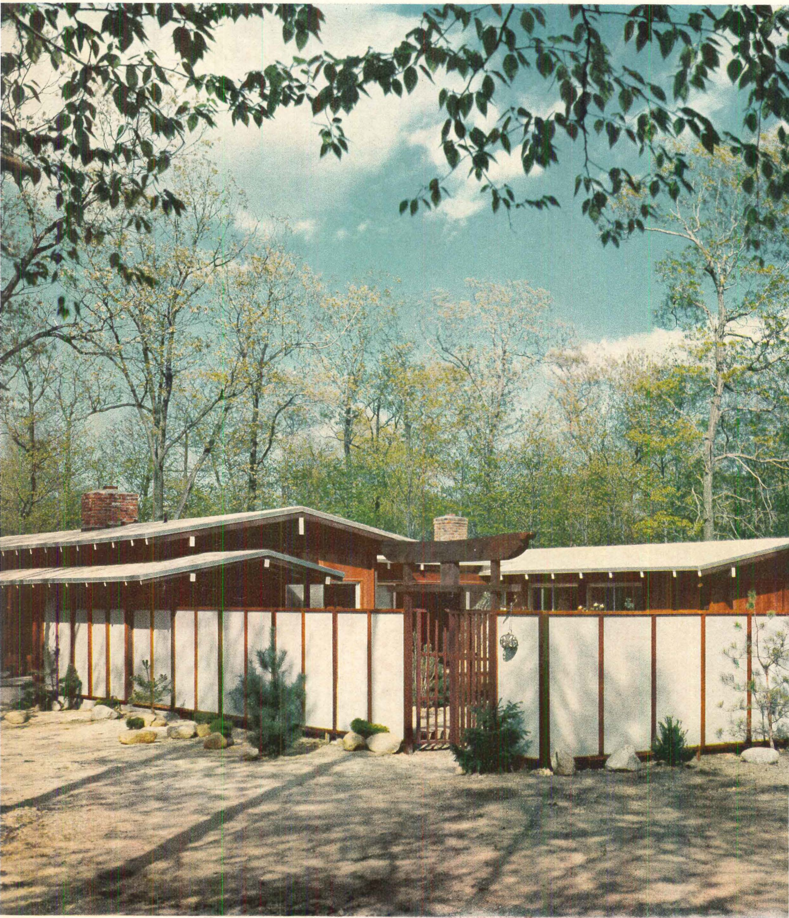
Garden wall extends from kitchen wing, left, around to bedroom wing, right. Wall panels are asbestos-cement left in a natural grey color and framed with redwood. Exterior walls of house are vertical redwood siding.
