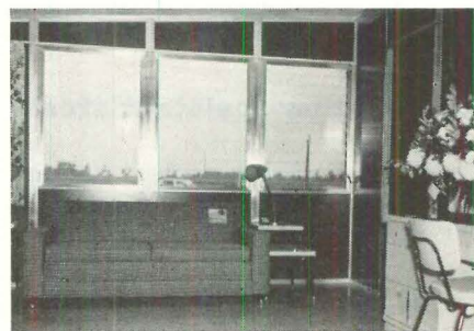
INSIDE , aluminum extrusions used for panel connections do double duty as trim. Panels are faced with wood-grained melamine.
