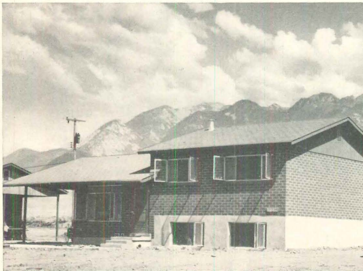
Larger of these two houses is first home equipped with copper tube plumbing in Cannon-Papanikolas development. Copper cost 13¢ more. Smaller home saved 16% using copper plumbing.
