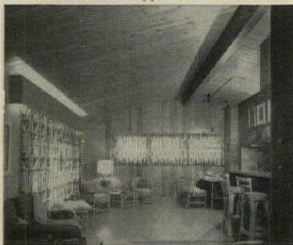
Rilco ridge beam 33' 6" x 5 1/4" x 13", Laminated lookouts 7' x 3-7/16" x 8 1/8", Rilco Fir Deck
