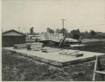
8:20 AM Trailerload of trusses arrives
