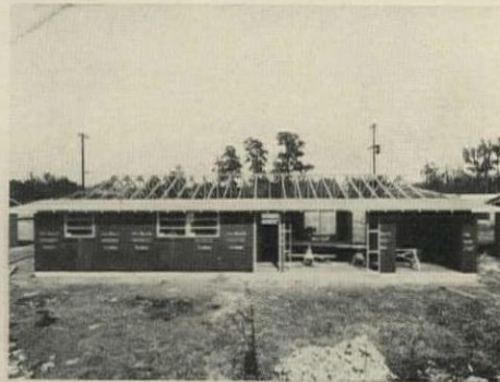
2:30 PM Sheathing is nailed to trusses
