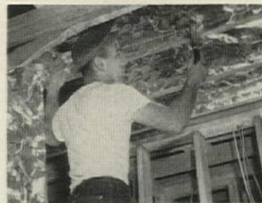
Save money on "one-man" installation. Lightweight blankets are self-supporting while handy tabs are stapled.
