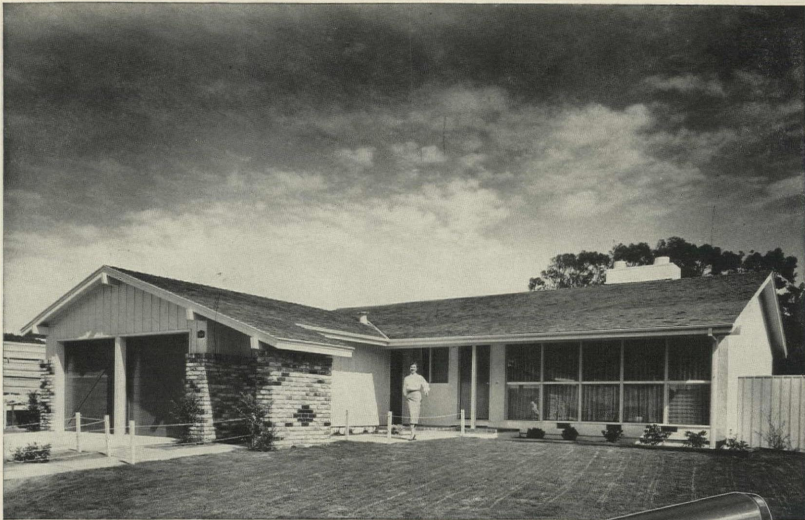
One of 10,000 attractive Stoneson-built homes in the San Francisco area.
