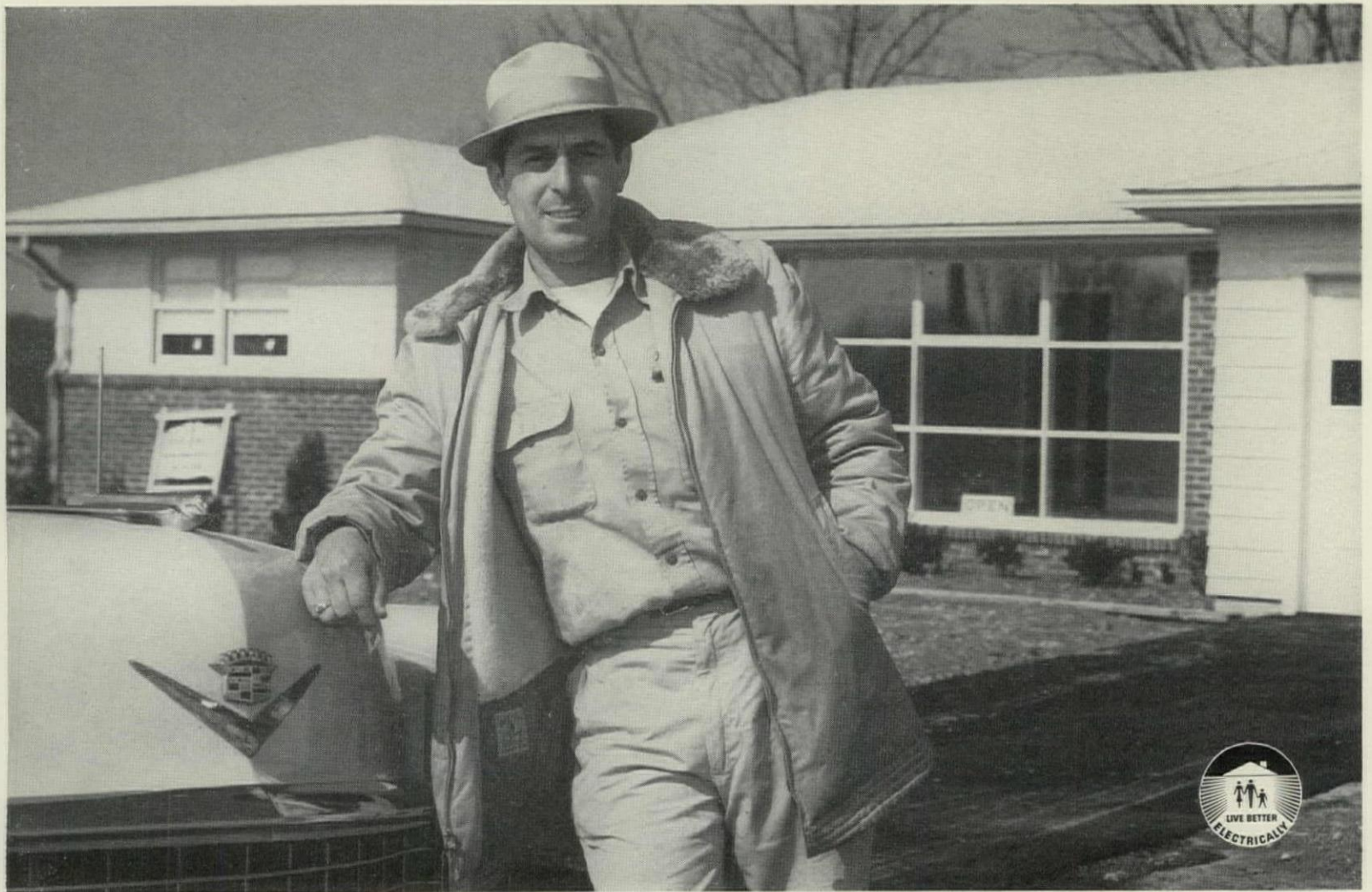
Mr. DeCesaris stands in front of a house in his attractive Oaklawn development, where G-E remote-control wiring is offered to customers at the same price as ordinary wiring.
