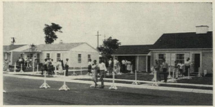
IN CHICAGO the Alexander Construction Co of Colorado Springs sold 565 of these National Homes prefabs in one month.
