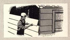
HARDBOARD SIDINGS. Beautiful, durable, easy to paint. Channel-Lap\* siding applied with aluminum channels; factory primed; invisibly fastened; self-ventilating. Verti-Groove\* panels offer modern vertical plank effect. Texbord\* lap, panel, or shingle siding; striated surface.
