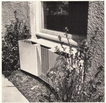
**OUTSIDE GRILL** fits over outer face of heat pump, provides plenty of space for air flow. Grill was designed by George Nelson.
