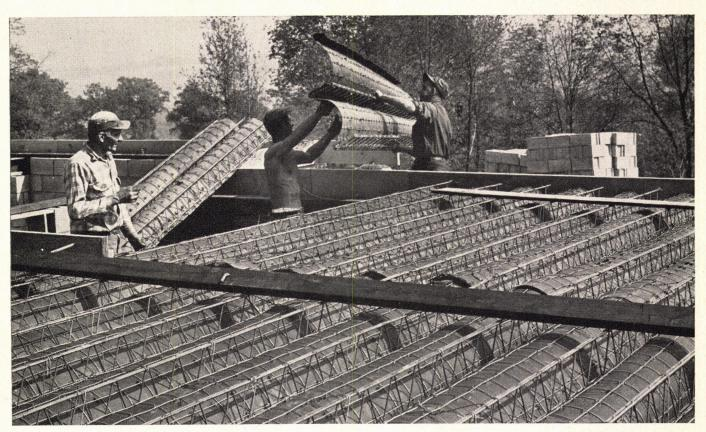
**STEP 1** Arched sections of wire-reinforced, paper-backed lath, with welded wire trusses laced between arches, are set in place. Outer end of 16' sections rest on foundation walls. In crawlspace or basement houses, inner ends rest on block wall down center
