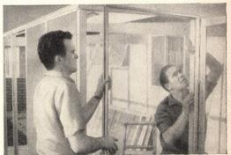
Fiberglas Screening in prefabricated panels spans large areas without denting or sagging and resists damage.
