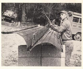
AT THE SITE Wire trusses, or reinforcing bars, are laced between arches. Male and female edges, formed in the arches by machine shown at left, lock arched lath sections together, help give sections strength to carry load.
