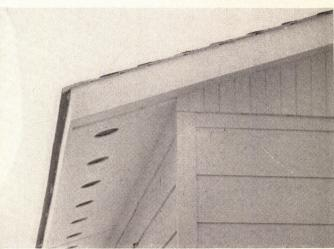
Test No. 15: "Soffit was designed to snap-in place—saved \$25"
