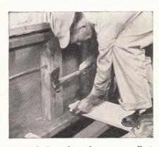
Wide baseplate along two walls is recommended to provide a good nailing surface for flooring ends, increasing rigidity of the installation.
