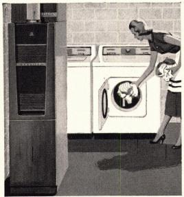
How about a furnace that permits the addition of cooling later? Then this Carrier Winter Weathermaker or "Furnace with a Future" is for you. Plenum for cooling coils is installed with the furnace. Ducts are sized for heating and cooling and insulated where necessary. Electric service for both (at least 100 amp.) is provided. And condensate drain and outdoor pad for refrigeration section are included.
