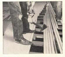
6 Use only tongue-and-groove and end-matched strip oak flooring. Blind nail to each screed. Stagger end joints for strength and appearance.
