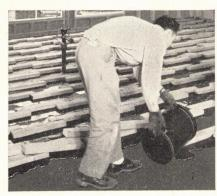
2 With moisture barrier in place, apply additional hot mastic under previously laid out screeds. Finish flooring is nailed to the screeds.
