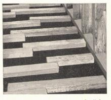
5 Leave a minimum gap of 1" between ends of screeds and baseplate around edges of room to allow for normal expansion of the finish flooring.
