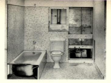
PACKAGED BATH UNIT, available to prefabbers this month, comes with white or colored fixtures (including wall-hung toilet, not shown), ceramic tile wall and floor panels that fasten to the frame of the
