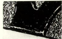
Over an extra weight base, on the exposed "weather half" of the shingle, an additional heavy coating of asphalt is applied in a distinctively grained pattern.
