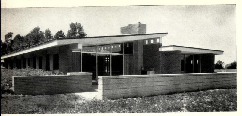
ALL-GLASS END WALL is made possible by the pre-cast roof channels, which span the 22' between bearing walls without intermediate support.
