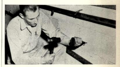
The Feldman Bros. Co., steamfitters, use a chain held by SHURE-SET wire loop fasteners, to support radiators. There's no drilling necessary.
