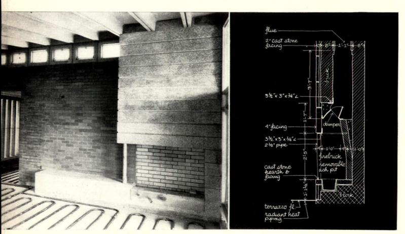
**CAST-STONE FACING** on fireplace is made of exposed granite and quartz aggregates in a colored cement matrix. This same material is used in the terrace wall (see top photo, page 144). Its compressive strength is 7,500 psi.
