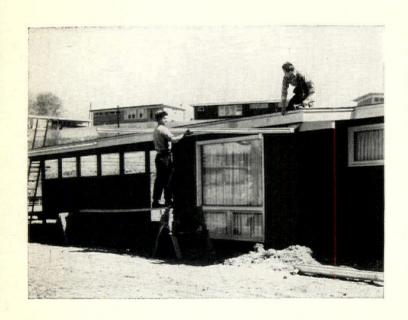
NEW! House-Long Gutters by Republic Steel. Lengths up to 32 feet can cut gutter installation costs by 50%. Long lengths eliminate seams and points of potential failure. Made by Republic's Berger Division from highest quality continuous galvanized steel. Send coupon.
