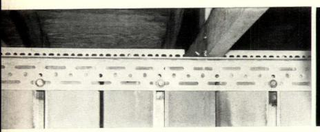
**ASSEMBLY DETAIL** shows inside of panels at top of wall. Metal channel runs full length down center of each panel, provides grip for anchor bolts wherever needed. Steel angle, in addition to tying panels together, acts as "plate" for roof trusses. Lag screws, driven into roof framing through top flange from the outside, tie the roof to the wall.
