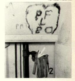
SLASHED FIRE HOSE (arrow) typifies vandalism, as does burned scrawl on walls above. In one 12-floor unit, not a hose worked.
