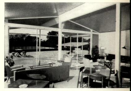
**INSIDE THE HOUSE**, no painting is needed because the interior finish is anodized permanently into the panel's aluminum skin.
