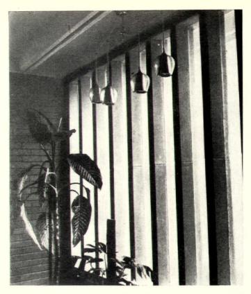
**PRE-CAST MULLIONS** for front-entrance window trellis are made of the same strong, marble-aggregate-surfaced concrete used for the window frames at left. Windows are glazed with fixed ½" plate glass set into a cast-in rabbet on the outer side of the mullion and caulked in place.
