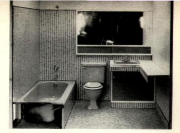
house, luminous ceiling, and prefabricated copper plumbing wall. In the photo left wall panels are removed to show plumbing wall; at the right is a complete unit except for fourth wall (missing in foreground).
