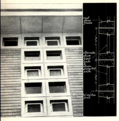
**CAST-STONE WINDOW FRAMES** in another of the bearing walls take roof load, transfer it to brick and block wall on which they rest. Both fixed and projected aluminum sash was cast right into the strong (7,000 psi) concrete, which has a dense uniform surface of marble aggregate.
