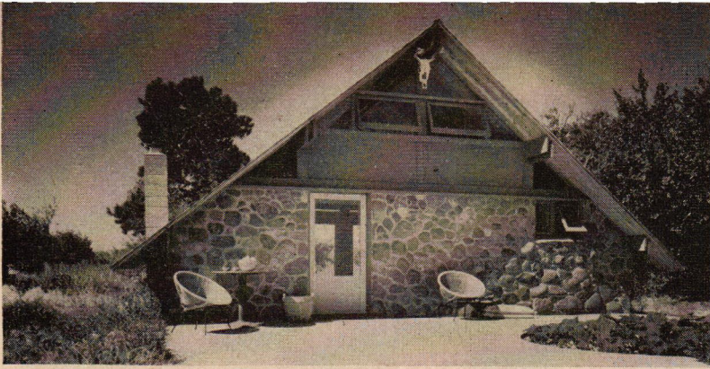
Entrance-side windows are for bath, right, and parents' sleeping balcony.
