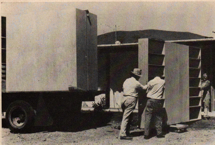
Shopbuilt cabinets were installed after frame, are movable for flexibility.
