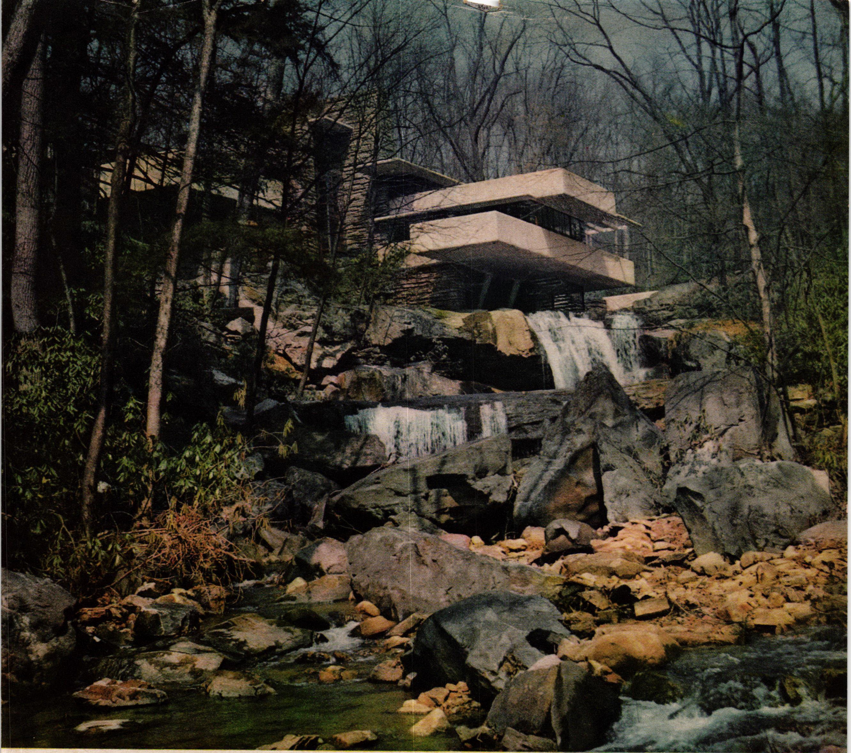
Kaufmann house, Bear Run, Pa., Frank Lloyd Wright, architect (1936). Photo: Paul Mayen
