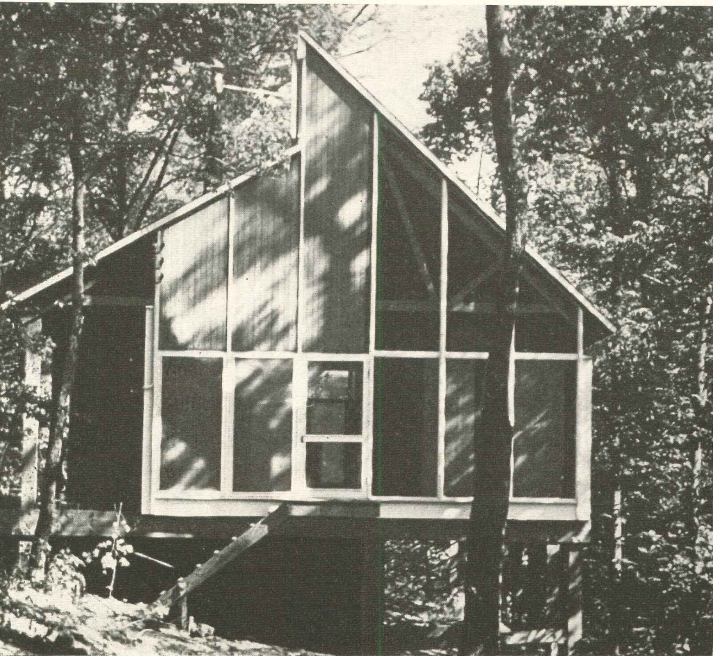
North elevation expresses dramatic truss frame with clerestory strip above. End wall panels are filled with glass or vertical redwood siding.
