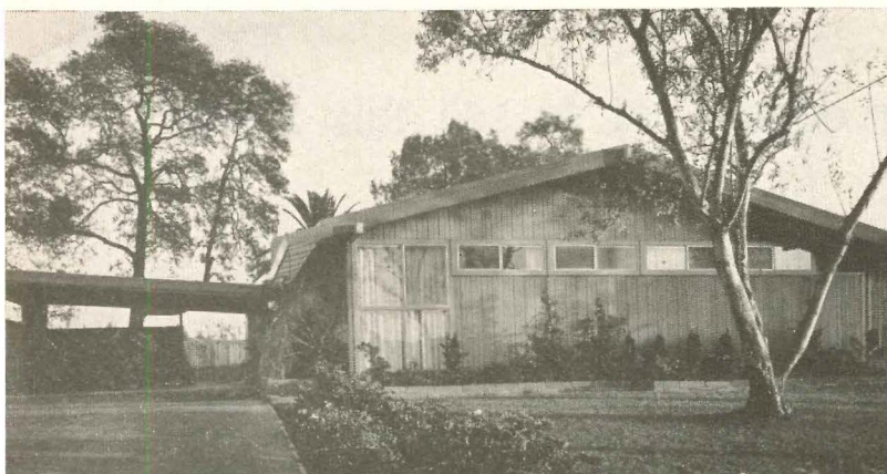
Striated siding has texture interest; windows create a pattern
