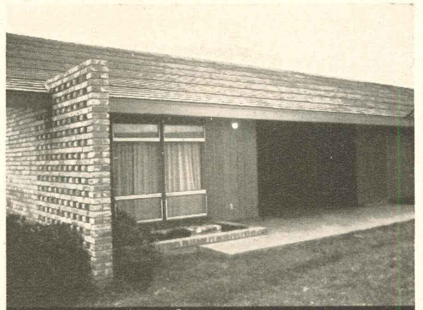
Builder: Ervin Blossing of B.K. Builders; Architects: Christensen & Connata
