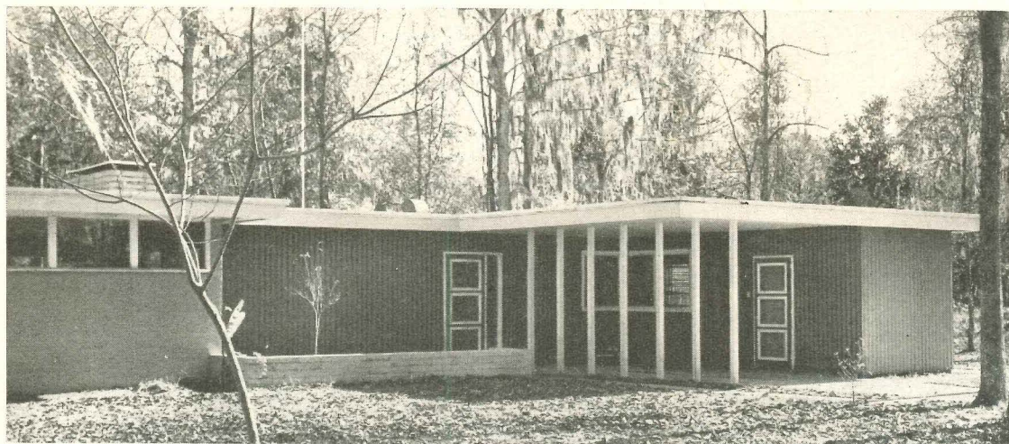
Corrugations give strong vertical lines to contemporary house, overlap one curve (4") where panels meet
