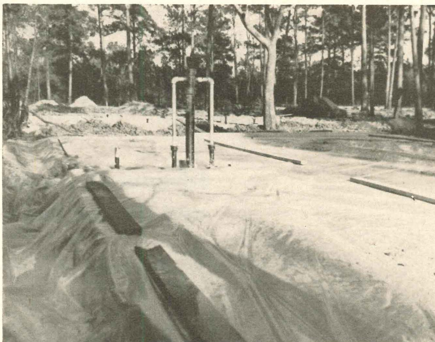
Film is kept flat with planks and a few shovelfuls of sand
