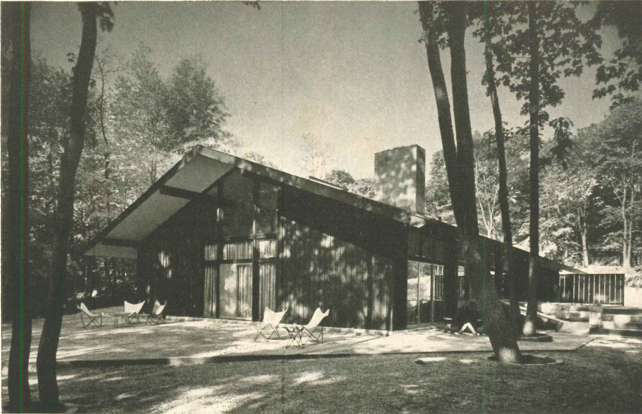
A 5-in-12 roof reaches way down to shelter the terraces that surround the house. Actually, eaves stop 6'-9" above terrace level. Glass end wall faces east and best view.
