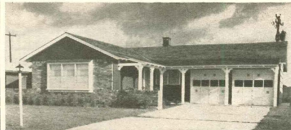
4. Early American "ranch" by Architects Dunaway & Jones, was built by S. E. McCrory. Facade is foreshortened by strong vertical posts.
