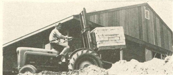
Fork-lift unloads pallets from truck . . .
