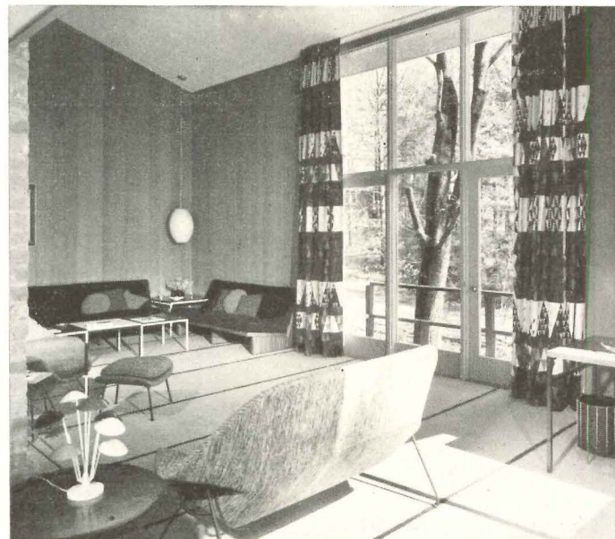
Living room ceiling follows 4-in-12 pitch of roof
