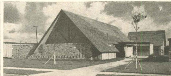
8. Old English design with a modern twist (sliding glass doors to yard) was designed by Christiansen & Cannata for B-K Builders.
