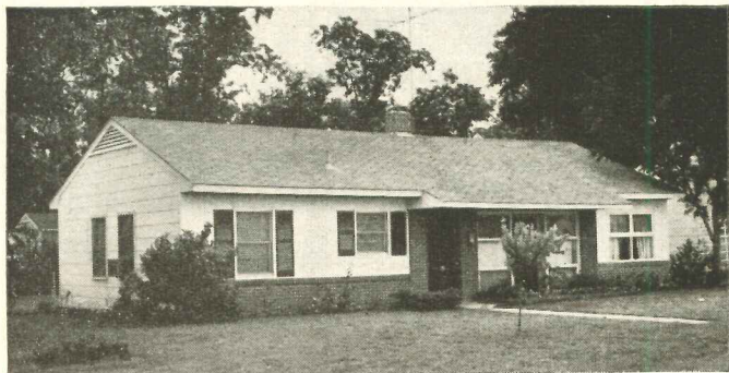
2 1952: Powell dropped house off crawl space and onto slab, gave an even longer lower look to an already enlarged house.
