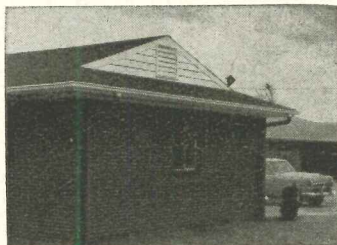
One 24" exhaust fan mounted over garage . . .
