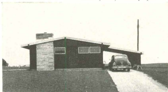
Versatility of Lu-Re-Co panels was demonstrated on this house with vertical redwood T&G siding. Panels were sheathed completely sided in Thompson's yard; final strips of siding over panels were applied on site. Method: siding was shiplapped end so it could be slipped into place. Builder: Ozier-Weller.
