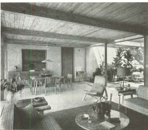
Post, beam and plank structure produces two wide-open walls on long sides of living room. Planks span 8' between beams.
