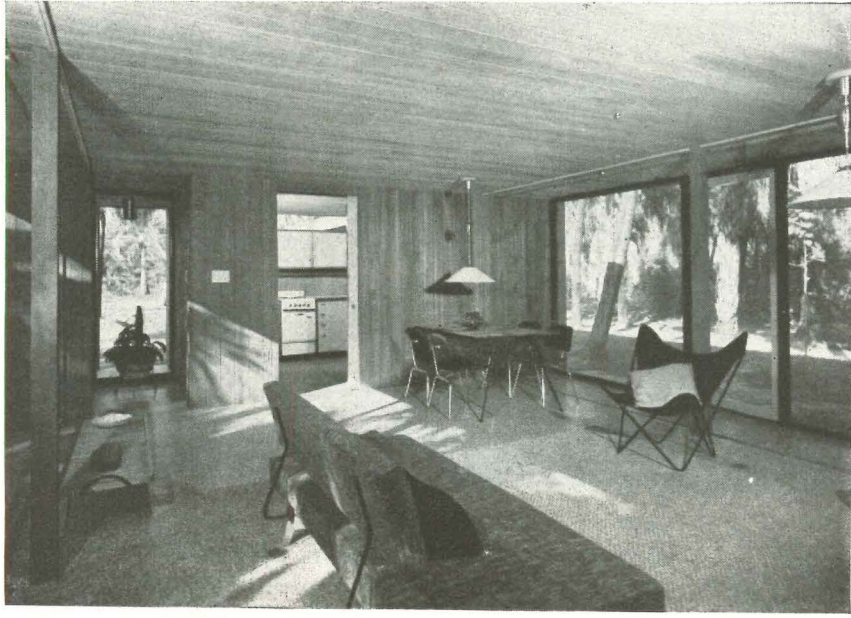
Dining area with kitchen beyond. Floor is 3/4" terrazzo
