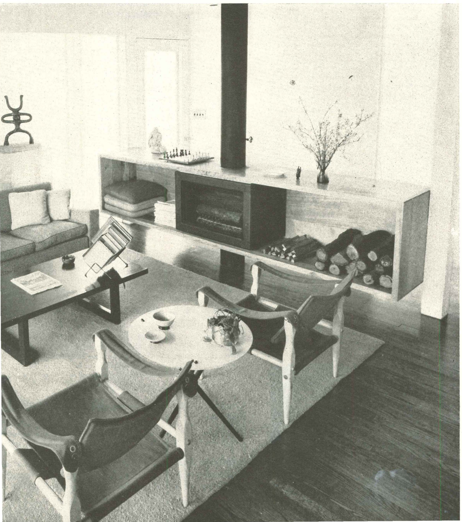
ing living-room feature is built-in metal fireplace. Designed as a "space-divider" cabinet, the metal unit helps heat the area. te unit is hung between two structural posts. Open passage cabinet counts as part of spacious living area.
