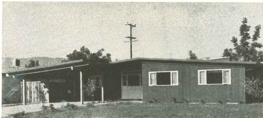
Movable sash flanking fixed sash in a privacy-high window facing street have balancing appearance of shutters, are far more useful.
