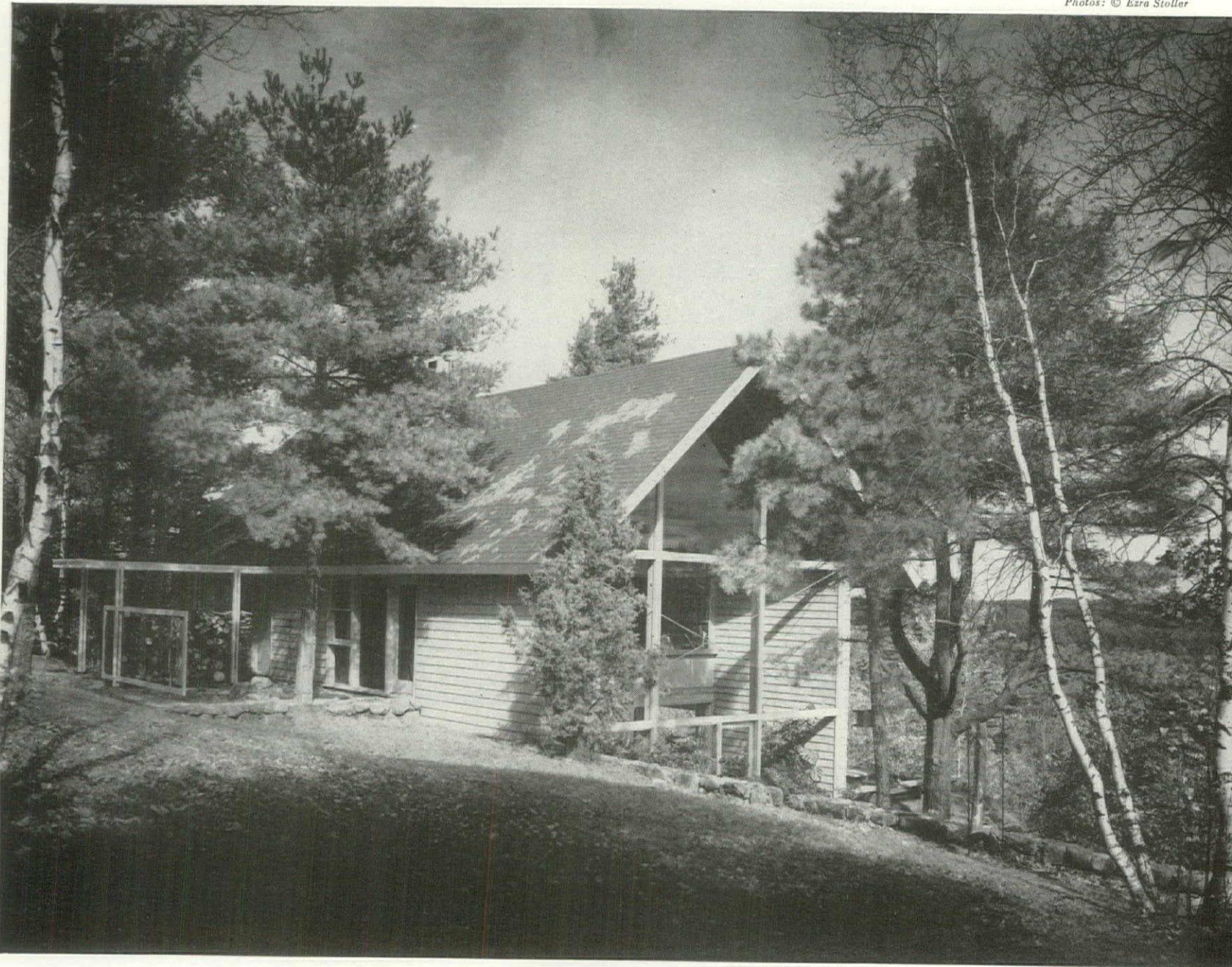
House on a hillside encloses living space with its uphill foundation wall. Terrace below gets main view (right), privacy from road (left).
