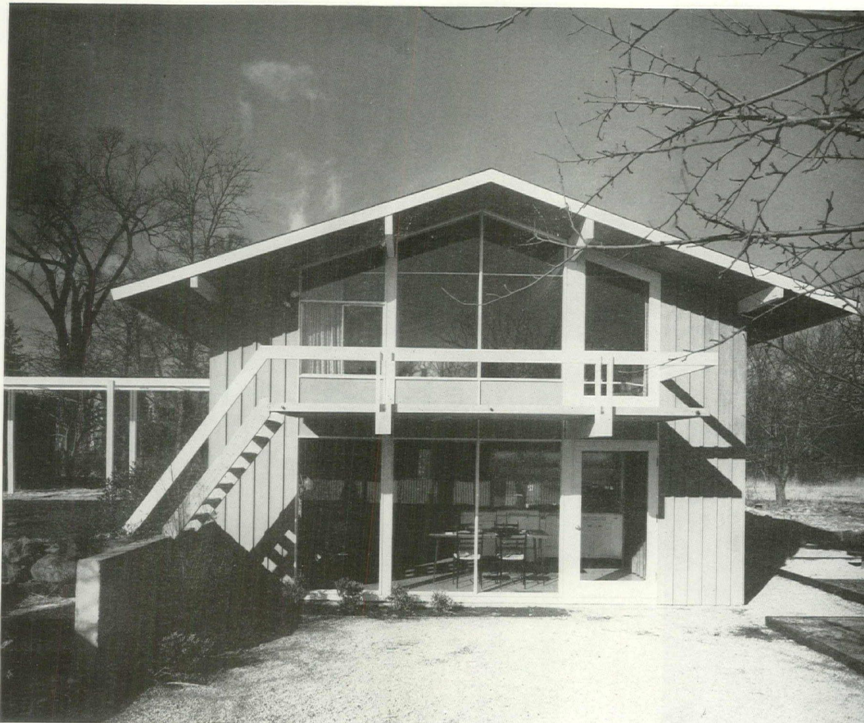
On sloping sites one end of lower floor can open at grade to an outdoor living terrace. Note extension of foundation (left)
