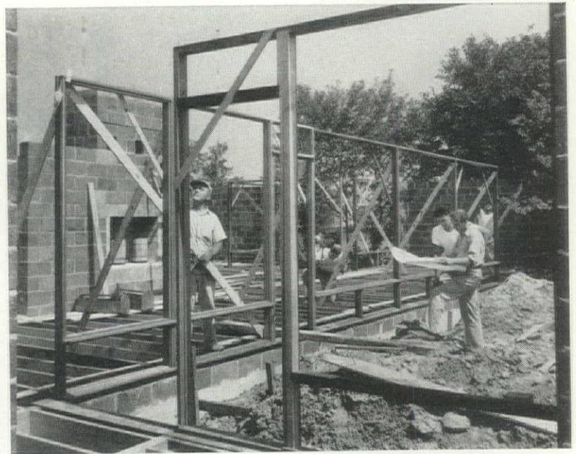
Basic design unit is 8' x 8' bulk frame milled locally to von Gerbig's design
