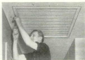
Complete automatic shutter unit fastens with screws to ceiling opening frame; flange forms ceiling trim.
