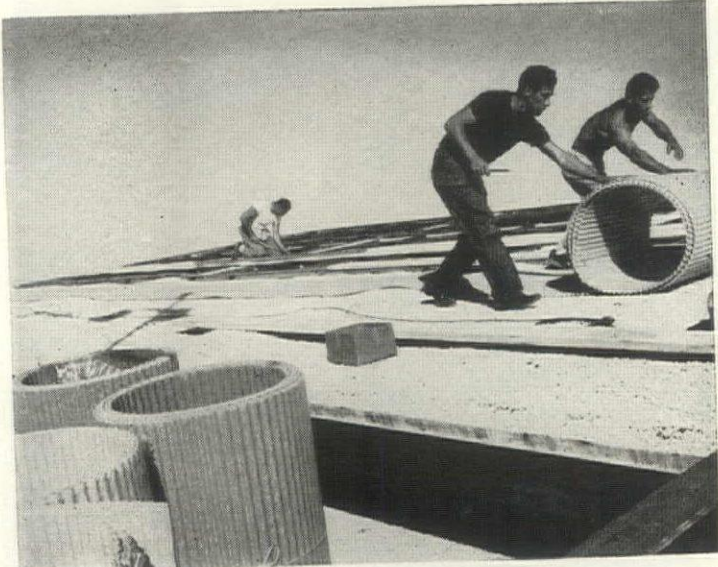
Rolled out from a 100' strip, the translucent plastic sheathing is easy to handle and apply.
