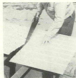
Tinsnips cut the flat, fibrous Alsynite panel (left); an ordinary hand-saw can be used on the ribbed Chemoglas sheeting (right).
