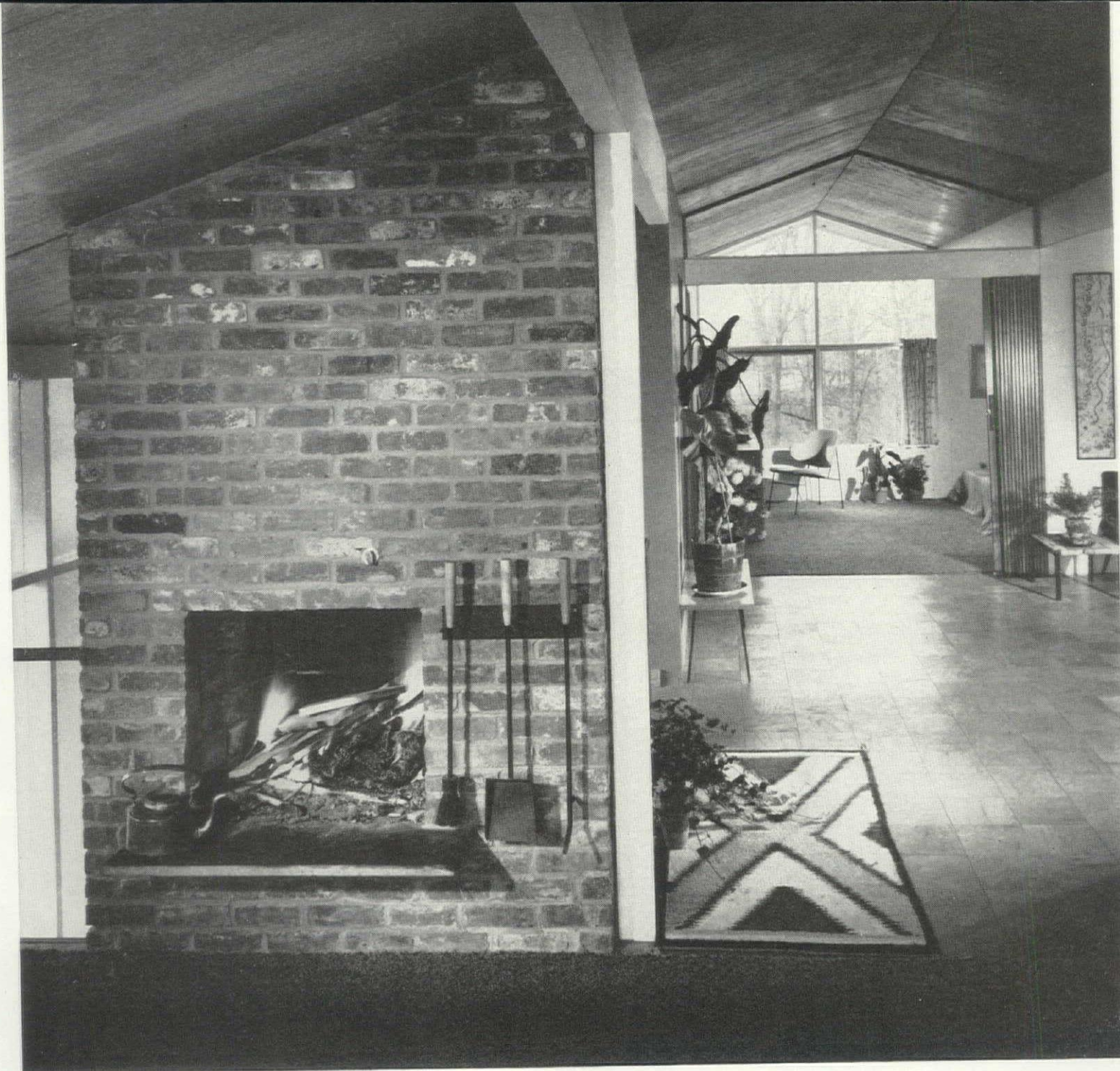
3. Bright, spacious interior is possible with roof supported on four posts and two beams, partitions placed only where necessary. This view, from living end, shows parents' bedroom almost 40' away.
