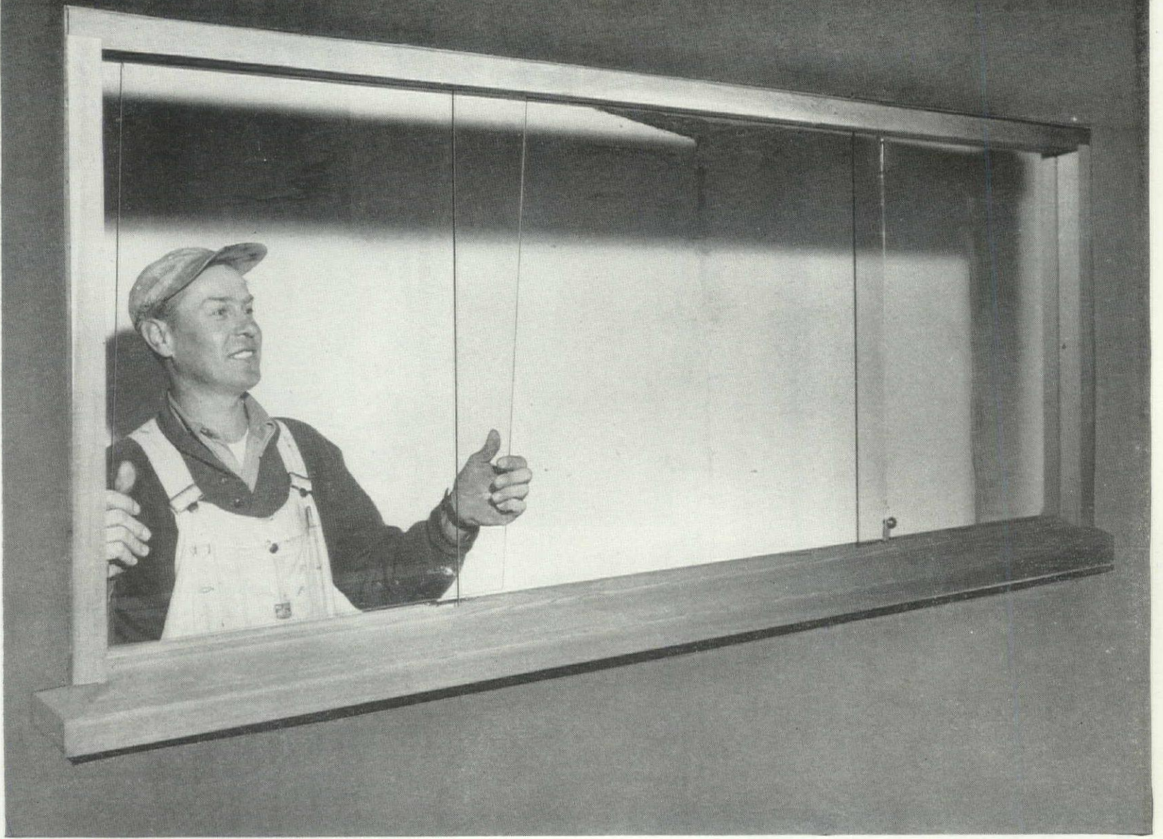
The glass panes lift out to simplify painting or washing.
