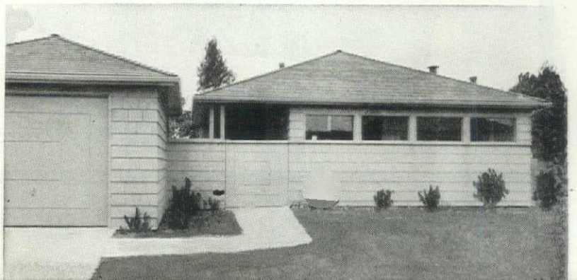
Installation showing a typical arrangement of Pierson Sashless Windows.
