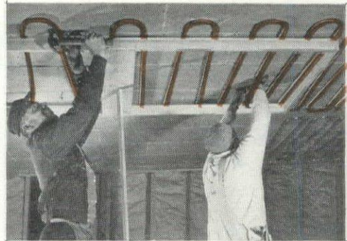
Lightweight PG's are easily installed. Trim, straight grids fasten tightly to ceiling — permitting a minimum, even thickness of plaster.
