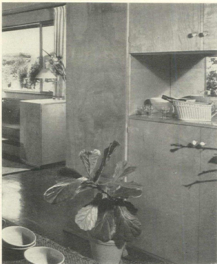
Closest unit facing dining area contains bar on one side, hanging space for coats on the other. Mirror in back of bar counter, which gives the appearance of a pass-through opening here, reflects light onto the mixing shelf.
