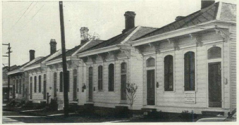
AFTER REPAIRS —paint, cement steps and walks, refurbished toilets and kitchens, and strengthened foundations—Conti St. presented this improvement, and one woman in the neighborhood was organizing a garden club.
