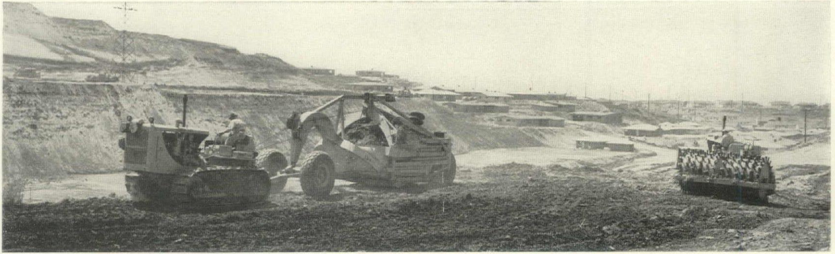
A million cubic yards of earth were shifted by carryalls (left), wetted down and then compacted by sheep's-foot roller (right).
