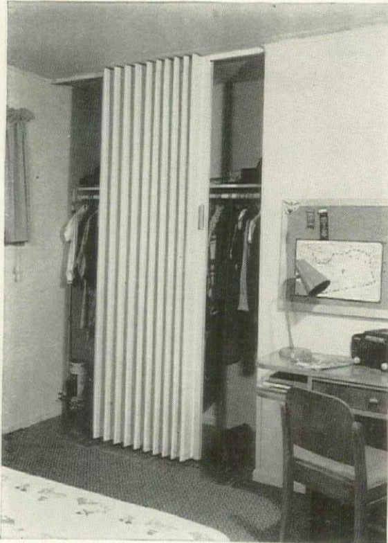
National Homes puts "Modernfold" rolling post doors on their big floor-to-ceiling double closets, to get full accessibility. No need to "build out" or "build down" to door.
