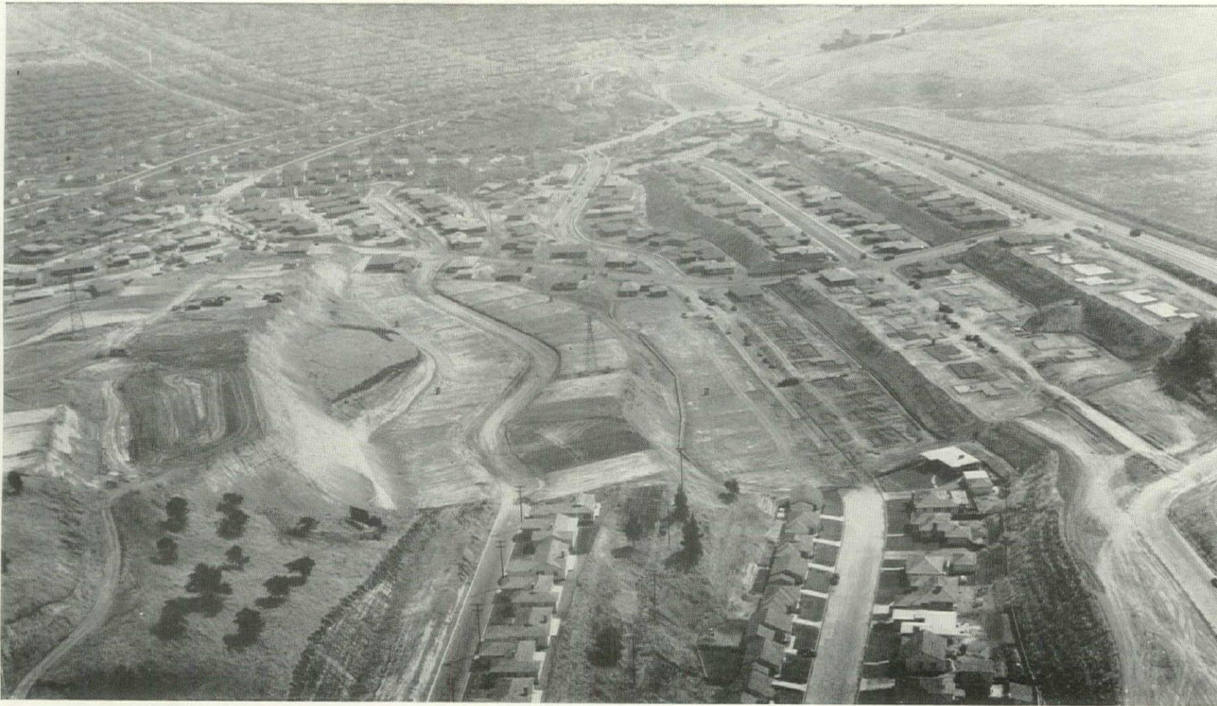
Broad terracing shows in sharp contrast to older development (foreground) which left most of hillside unusable
