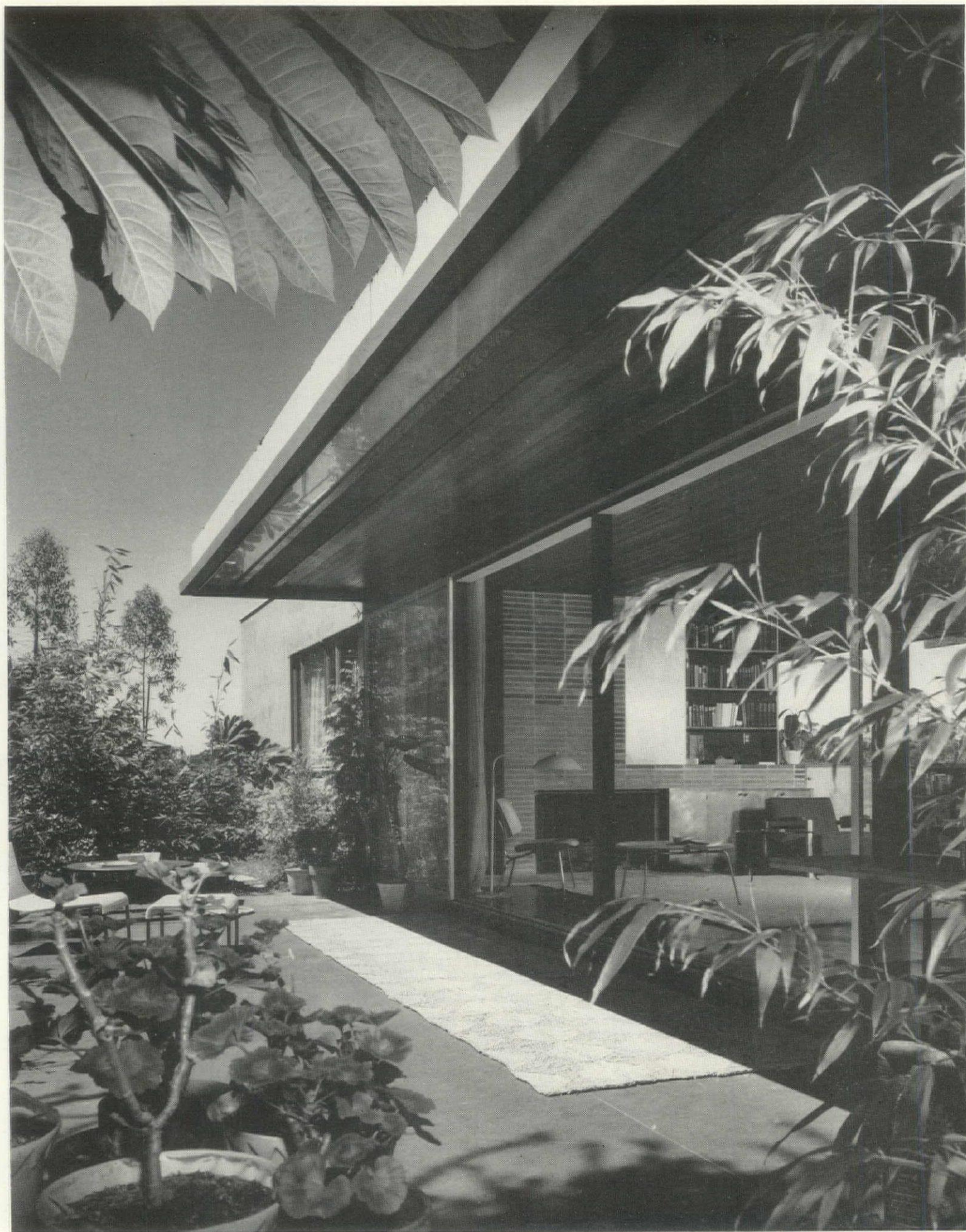
Outdoor living room was created by leaving a level space 12' wide in back of the house, opening up both living and dining areas through large sliding glass doors. Sense of indoor-outdoor enclosure is heightened by the wide roof overhang and by the planted back slope, which makes a fence unnecessary.
