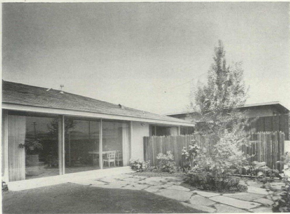
Typical house, shown also in plan and photos (right) is one of six models offered
