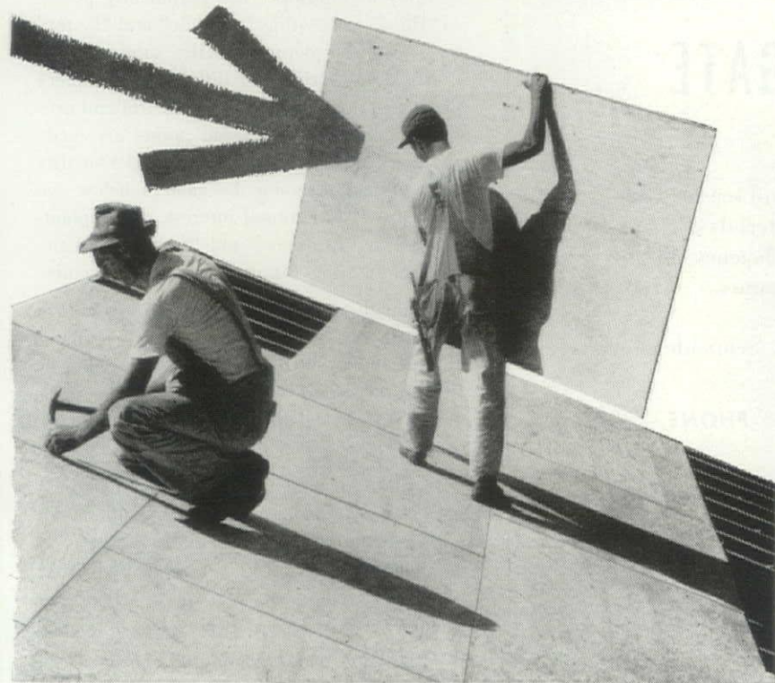
PlyScord holds nails well. Tests on roofs exposed 2 years show minimum force of 85 lbs. required to pull cedar shingle from 5/16" PlyScord. In case of asphalt shingles, roofing is invariably torn from PlyScord without loosening nails. Other tests and actual experience shows 5/16" PlyScord holds nails as well or better than 1" soft pine boards.
