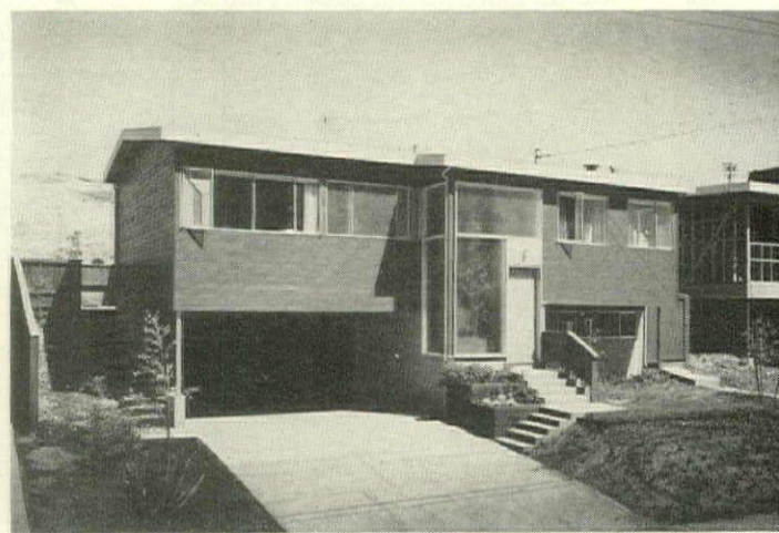
Lower floor, with glassed-in entrance for extra daylight, has carport, storage area, furnace room, an unfinished 14' x 24' room, bath with shower. Fences give privacy on 55' lot.
