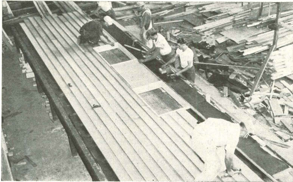
Side walls are completed down to siding, window frames in Trinity's shop. Jig tables are at convenient work height, materials close by. Overhead travel hoist moves entire panel to back of shop where prime coat of paint is applied.
