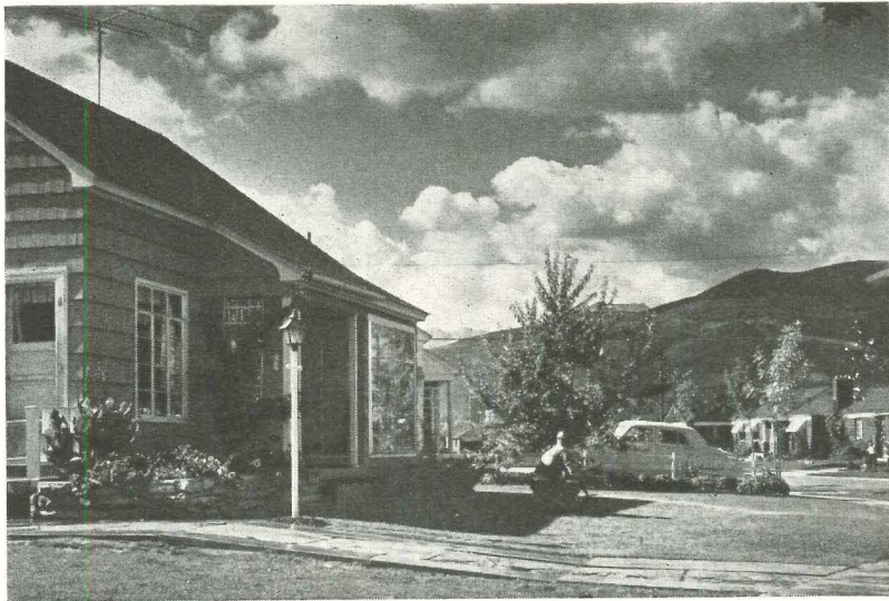
Brockbank's houses from 1946 (above) to 1953 show his own progress
