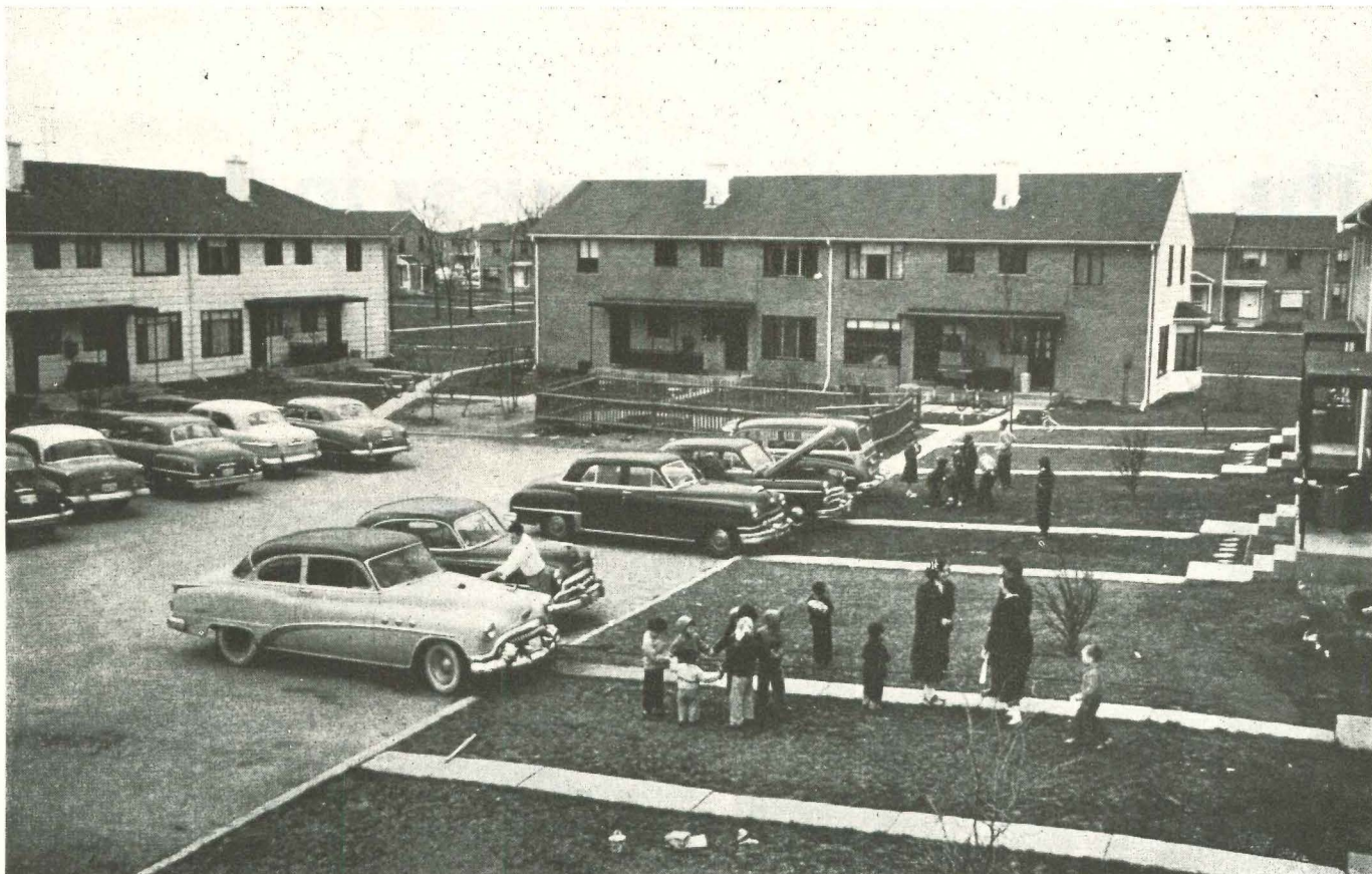
Rental courts: residents congregate on the cul-de-sac street. Note "tot yard," center background
