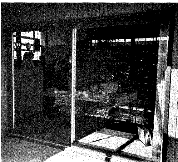
Sliding glass doors with wood top and bottom, aluminum sides and frame, builders say are about half price. A south California firm makes them. See details at right.
