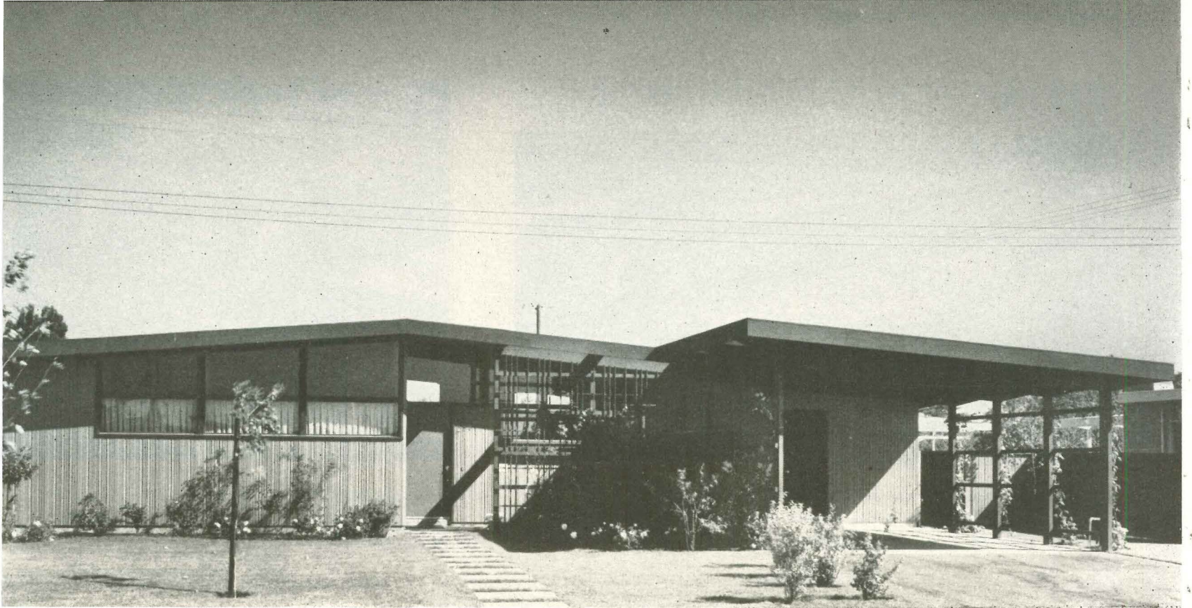
Scored redwood siding, same as used on luxury houses, gives rich appearance
