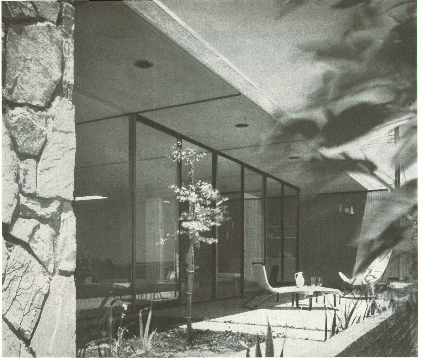
Massive stone chimney, left, vertical siding, right, and ceiling plane extend outdoors to frame the "view garden"
