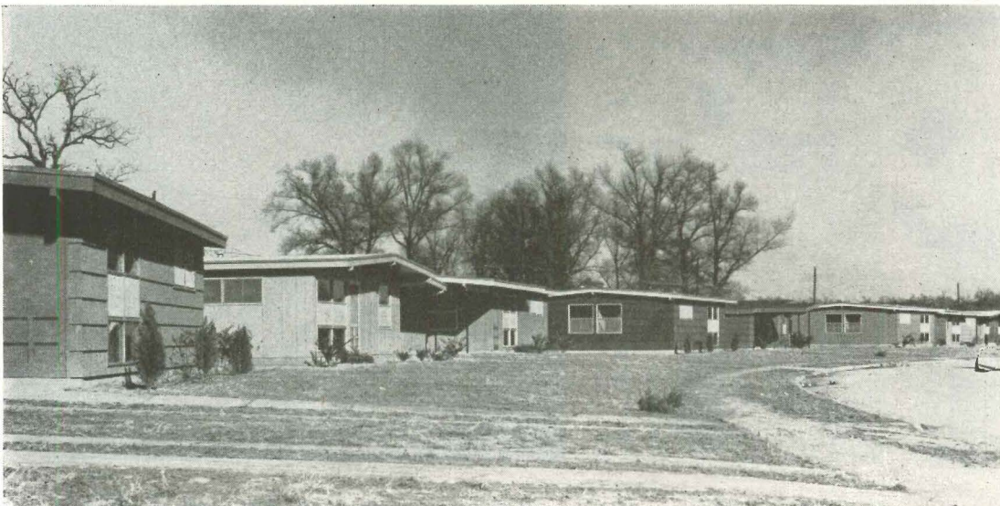
Setbacks, nearly uniform, do not appear so because of curvilinear streets, offsets in faces of buildings. Slab construction relates house to ground closely.
