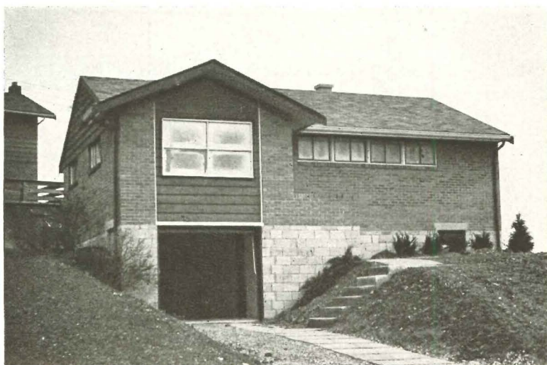
Sloping terrain permitted basement garages. Since site of development was previously undeveloped land, promotion accented community recreation areas, new gas lines, $250,000 sewage disposal plant and roll curbs. Wide overhangs, new in this price class, were well liked by buyers. Circulation through living room may be a problem since traffic flow from front door must cross living room to get to the kitchen and bedrooms.
