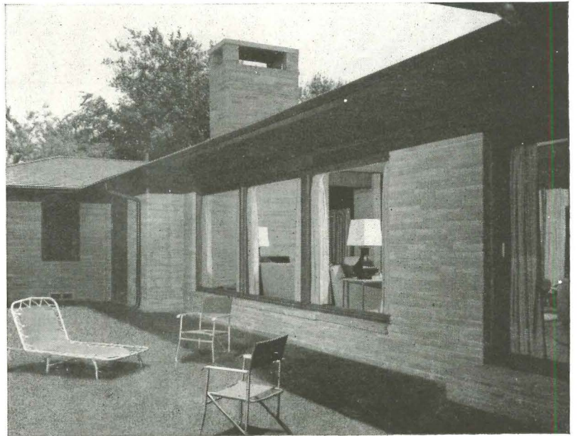
This exterior view shows how Architect Welch provided a roof overhang to shade south windows from the sun in summer.
