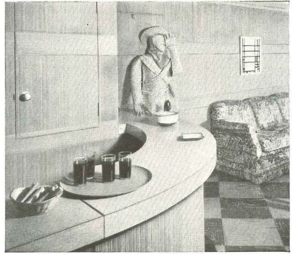
Here's the corner of a playroom designed by Fred Gerstel which shows an interesting built-in and horizontal-vertical Weldtex treatment on the wall. Note bar top of Westinghouse Micarta.
