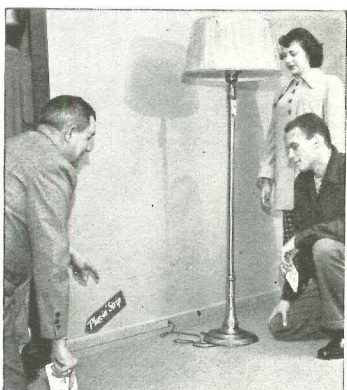
Plug-in strips are economical, permit free furniture placement. Lamps may be turned on or off directly or from central wall switch.
