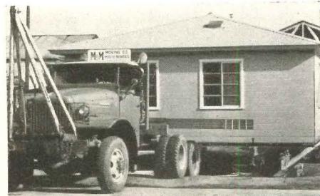
Right off assembly line, a Mobilhome is trucked to site, set on foundations . . .
