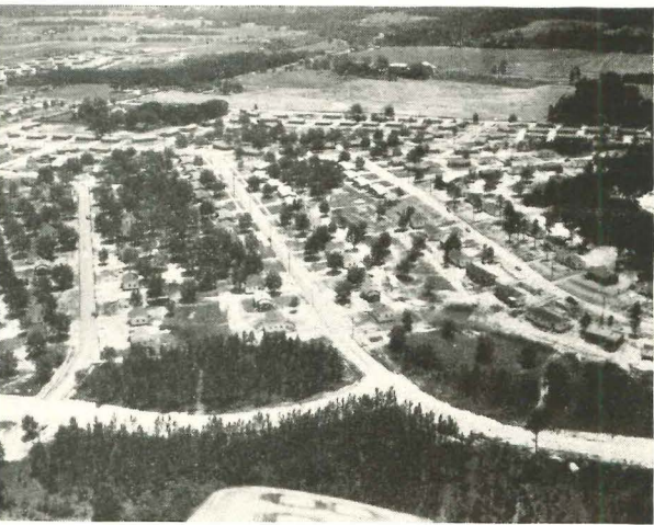
... concentrates on building large subdivisions of govern- ment-programmed housing in critical areas like the Savannah River, these 180 five- and seven-room units in Fleming Heights, Ga.
