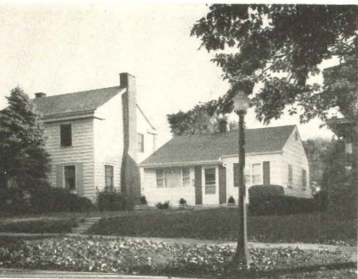
Not uncommon are prefabricated houses among conventionals. Small house is two-bedroom General Industries model.
