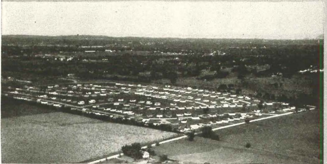
Flood-disaster housing was supplied by Page & Hill, which built a 250-unit project in Topeka, Kans. (above), another for Pierre, S. D.
