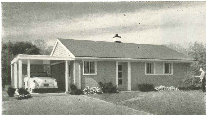
"195X" research house at Mequon, Wis. (plan, right & photo, p. 93 by architect John Normile. It has open plan, rear living areas and rear bedroom to go on narrow lots.
