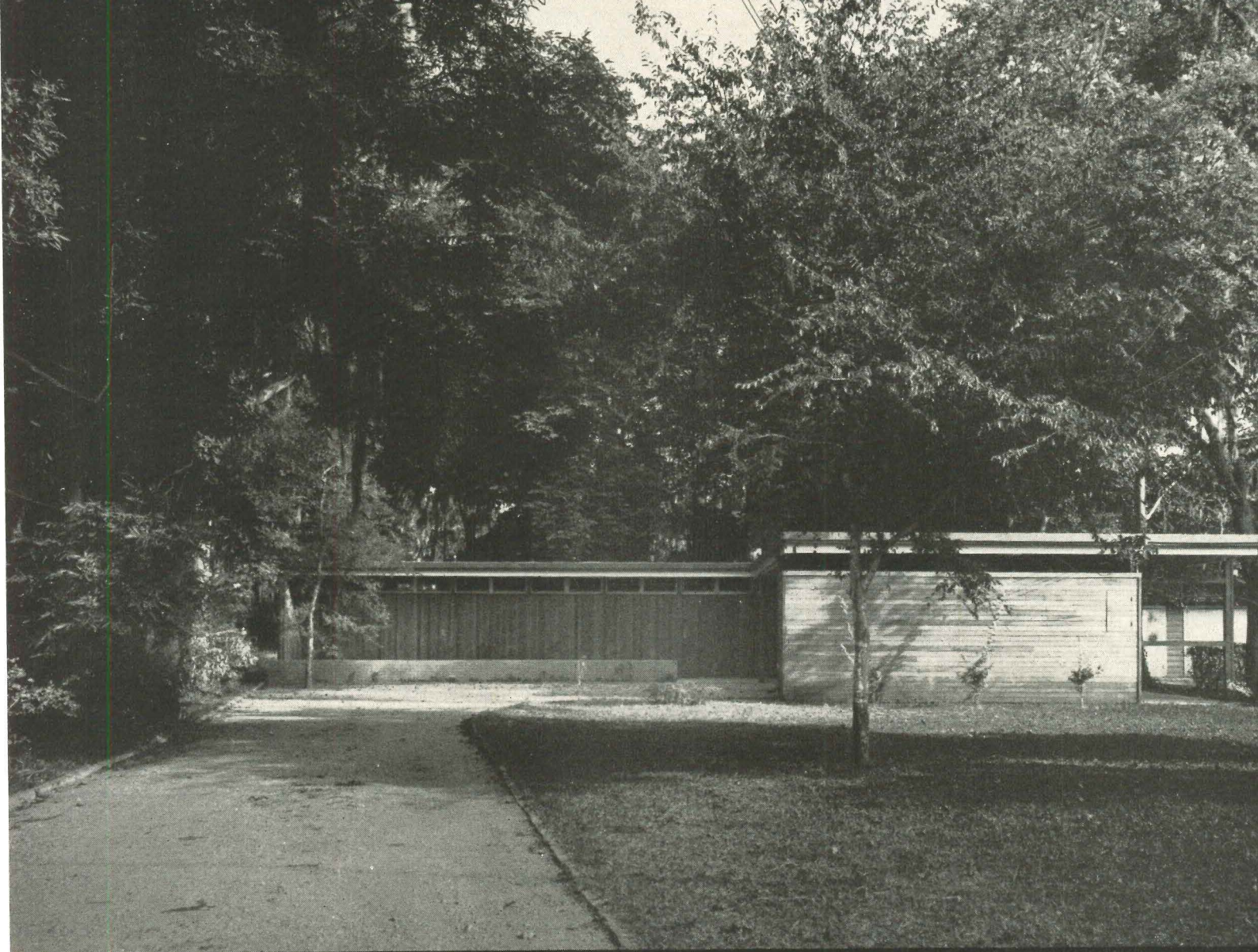
The front of the house, facing a 90° curve in the street, meets the problem of on-coming car headlights with a nearly solid wall. A strip of windows at the ceiling line provides adequate light and cross ventilation.
