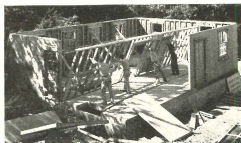
Walls are up at 11 a. m. Interior wall frames, often shipped in full-length sections, are easily tilted into place.
