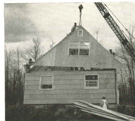
Some firms ship panels complete with windows and doors, insulation and interior surfacing.
