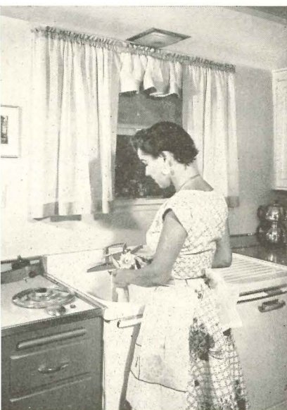
In the Blo-Fan electric exhaust ventilator, simply loosen one part by hand, and the grille and motor assembly are easily removed. Washing with soap and water cuts all grease off the parts.
