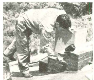
Rest of masonry, left, is built over the synthetic rubber flashing to provide tough, weather-resistant joints that, tests indicate, should be good for 20-30 yrs.
