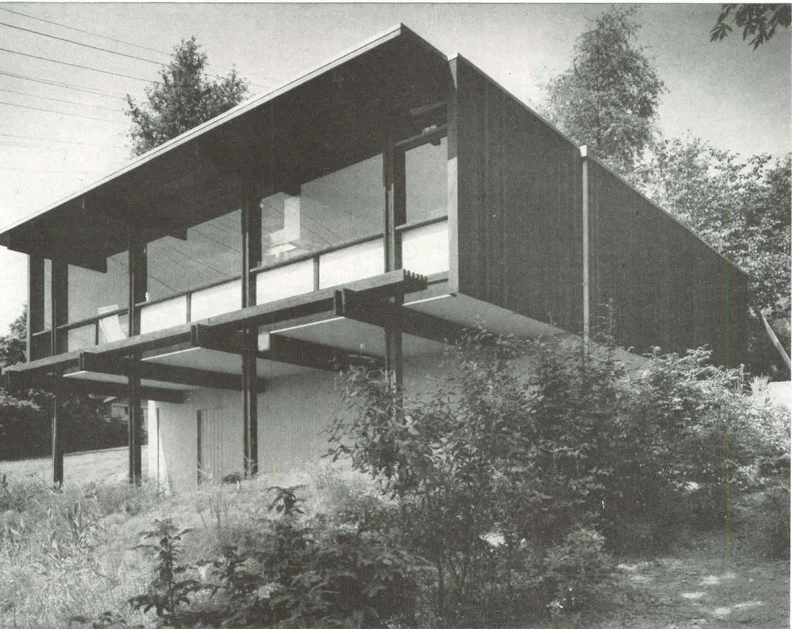
East elevation has glass wall for main lake view and morning sun, wide overhang to reduce sky glare and hot noonday rays, catwalk for window washing. Gray-white panels below windows are of cement asbestos board.
