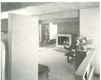
View from entry, below, shows open plan, exposed beam-plank ceiling.
