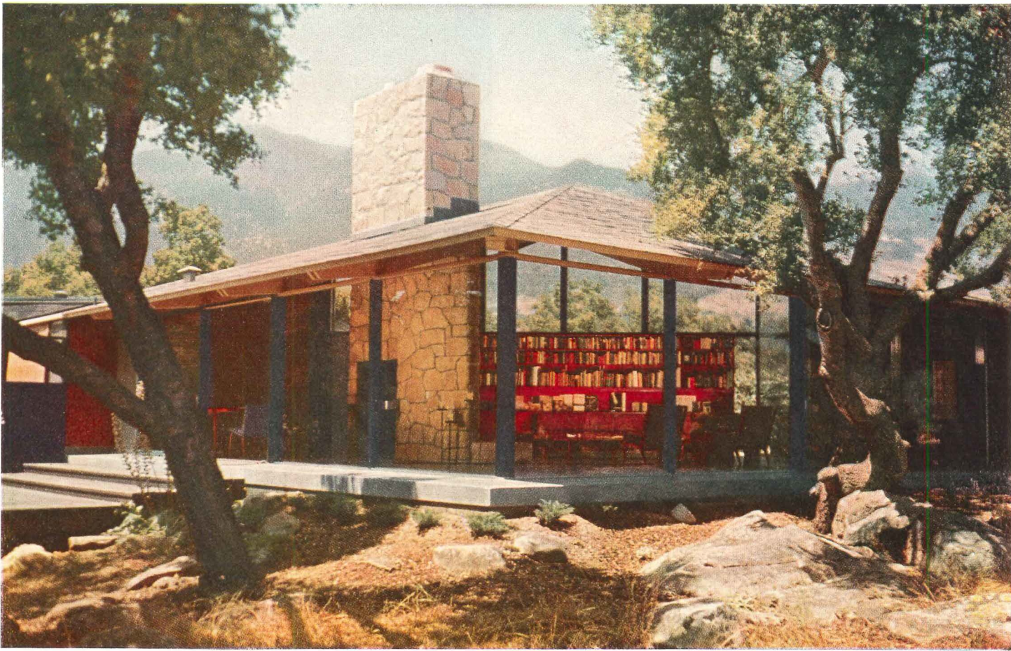
Southern tip of glass tent is shielded by low roof, deep overhang
