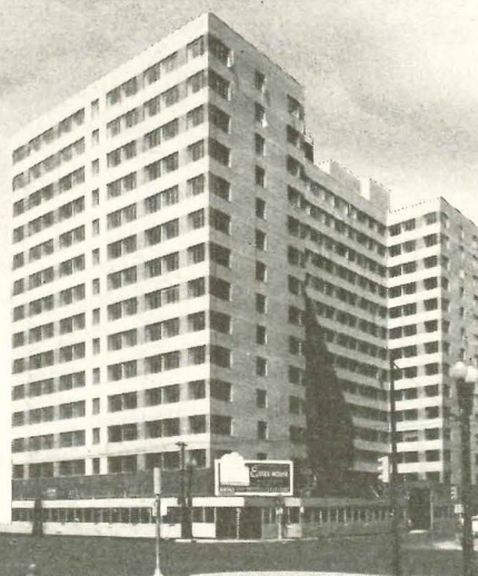
Essex House 390 Dwyer Kitchens
