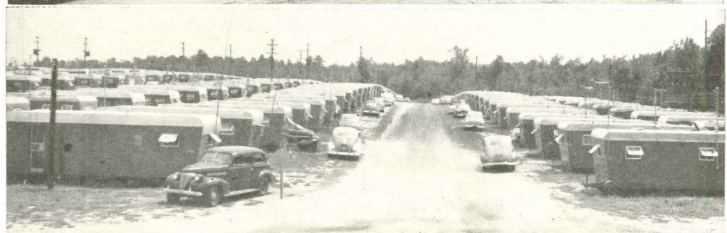
TEMPORARY HOUSING for construction workers at the AEC's Savannah River project include the barracks (at top, photographed during construction) and this trailer city at Barnwell, S. C.
