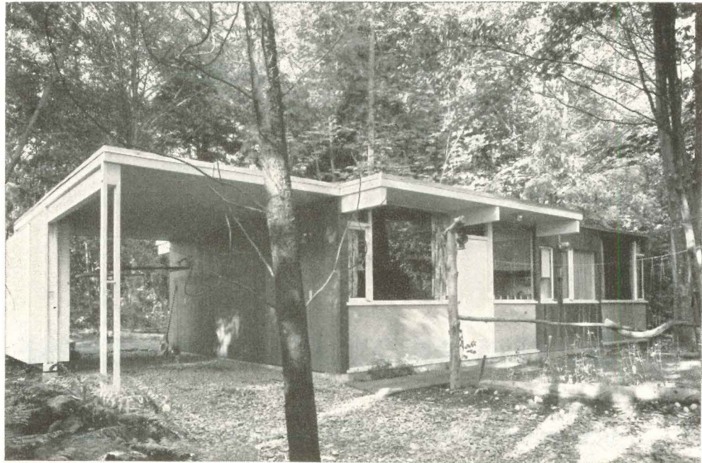
Reversible plan permits main entry on kitchen (above) or living room sides
