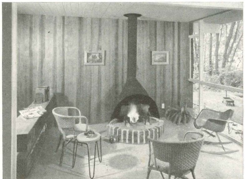
Living room: beam ceiling, cedar-plank and glass walls, $62 iron fireplace
