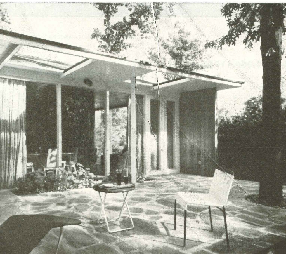
Solid wall of the new living room extends to shelter-glass wall and adds privacy to the terrace. Wide overhangs cut glare, have openings to allow sun to fall on a planting bed which parallels the glass wall.
