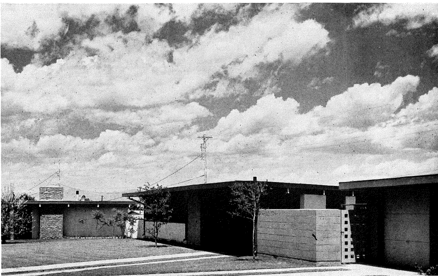
Pumice block walls connect the houses, below, make them appear larger and hide side service yards.
