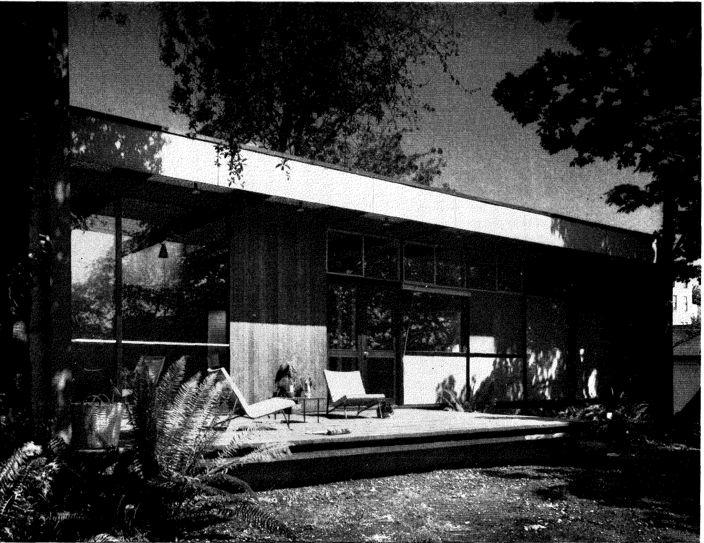
Garden facade is almost all glass, faces west. Porch at left is cantilevered like rest of house. This cantilever all around the periphery of the building gives it lightness and grace, crisply defines the building's silhouette.
