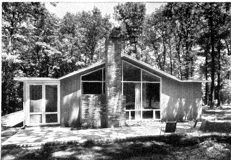
New gable end of glass lights living and bedrooms
