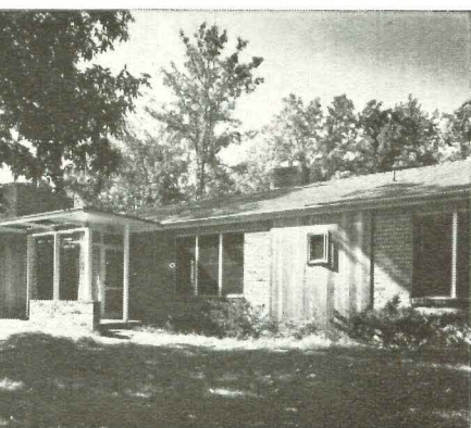
ing wing, left, ties into old house
