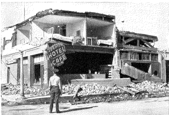
JUANITA HOTEL , where one man was killed, was rated as completely destroyed as was building at right. Construction: unreinforced brick.
