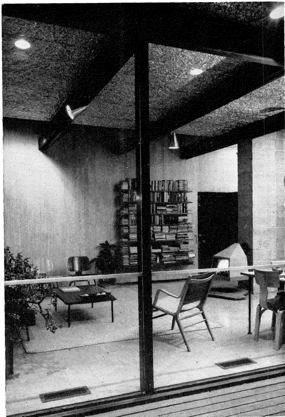
Skylights are angled to make light bounce off aluminum-foil surface and back onto east wall. Picture below shows night lighting, reflections in aluminum-foil ceiling.
