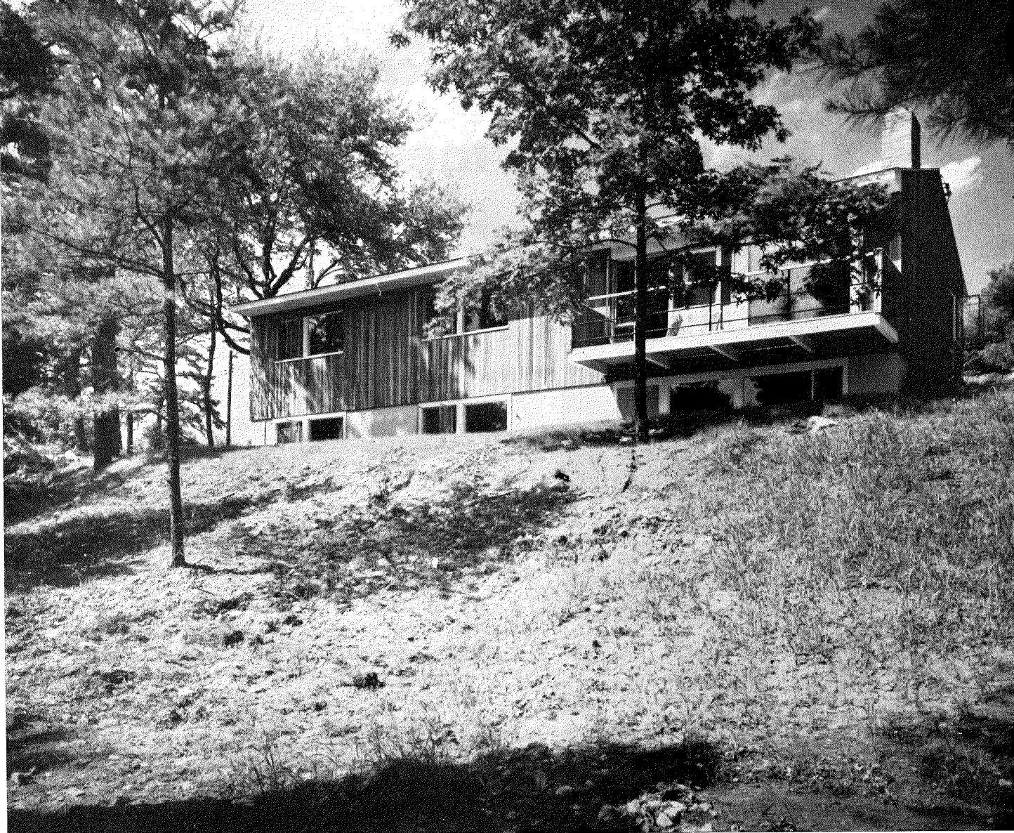
Upper-story living room of this hillside house opens through glass to balcony and view
