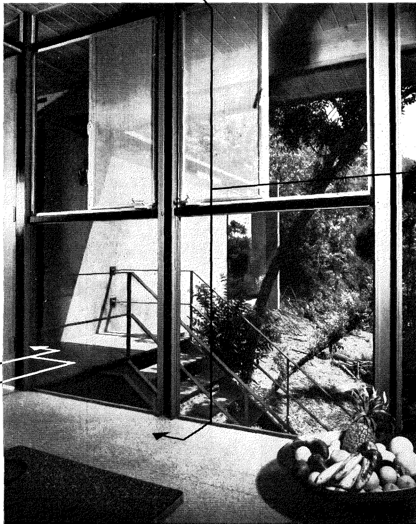
Wall panels, above, are bolted or screwed to column flanges. The cement board for the two opaque panels of the study is a Canadian material with a smooth, black-and-white stippled finish.
