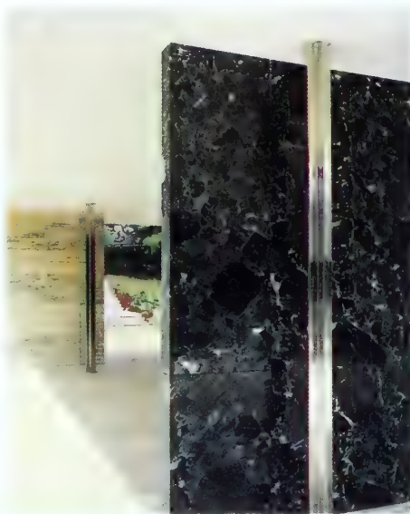
Structural columns of steel stand inches in front of nonstructural marble walls.
