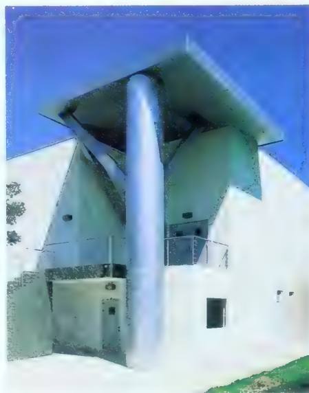
Gehry's Information and Computer Sciences—Engineering Research Lab, University of California at Irvine, 1986.
